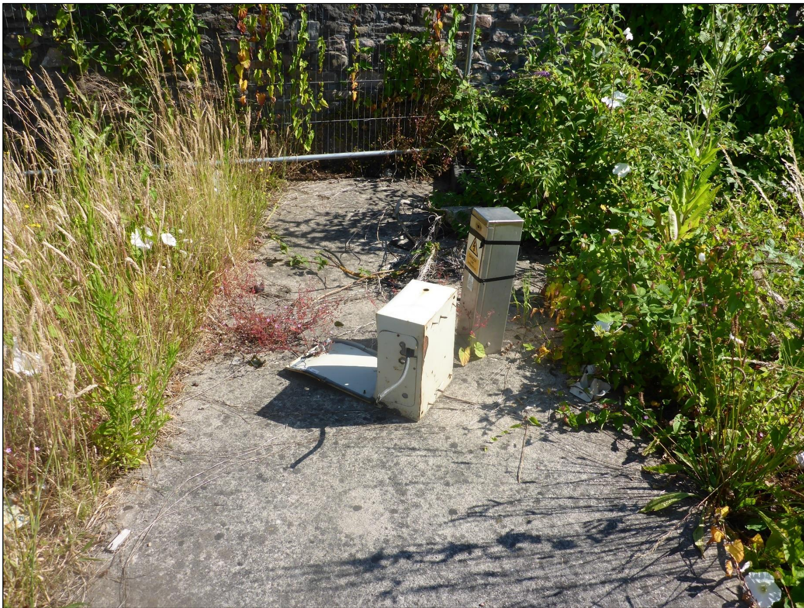
Figure 3. Concrete plinth and electricity cable on west of site.
