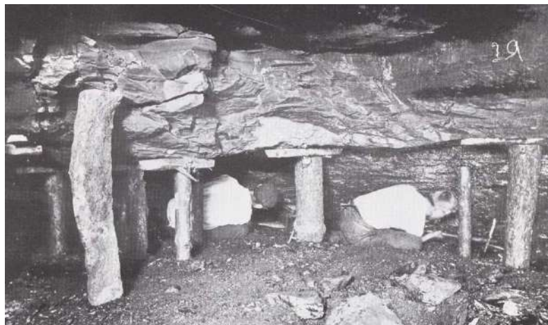
Undercutting the coal on a face at Coalpit Heath Colliery about 1900 (Burrows collection, BRO)
