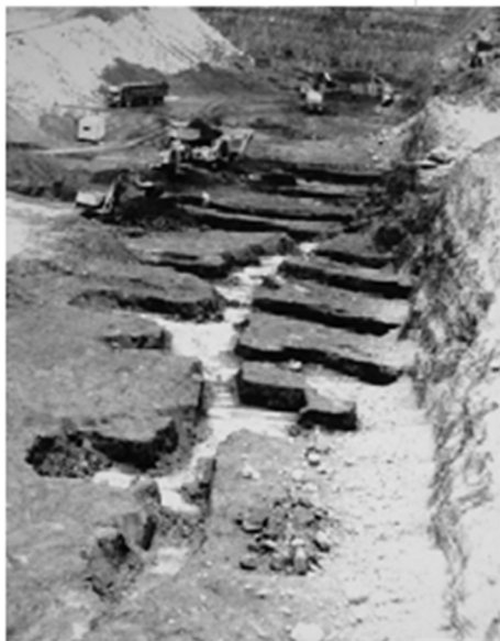
Evidence of early heading and stall mining uncovered in South Wales in 2002 at Morrision, near Swansea. Photo courtesy of Richard Jones©
