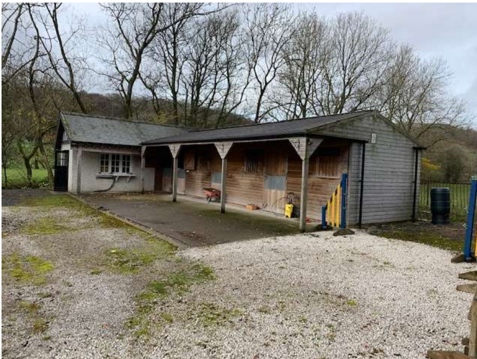
Existing timber stables to be retained and used for cycle storage
