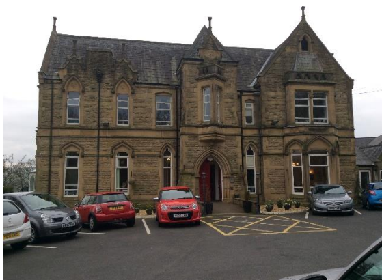
Front elevation viewed from Church Road
