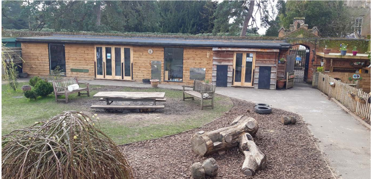
Image 4: Outdoor classroom with office located at Nursery Lodge
