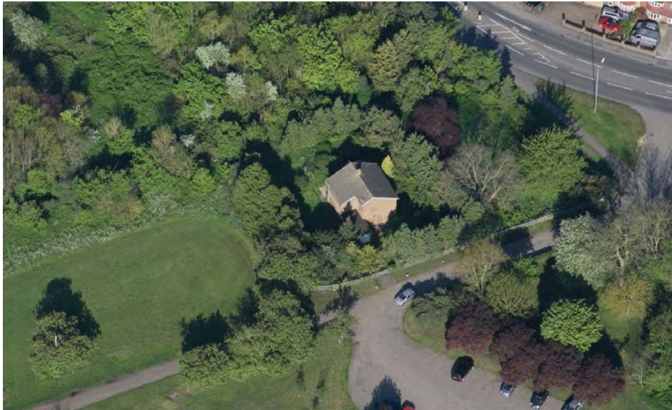
Image 1: Site aerial view facing west (Bing Maps)
