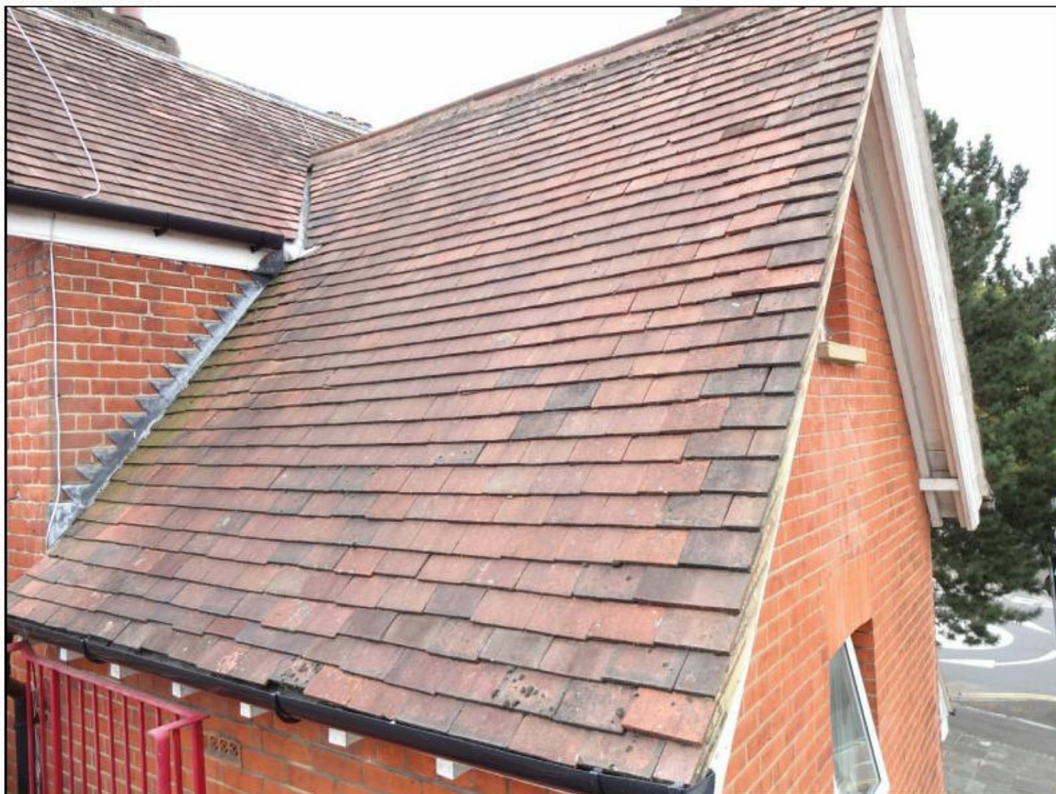
Figure 4. Example of tightly fitted roof tiles. Epsom Lodge Care Home, Epsom. 09.09.2020
