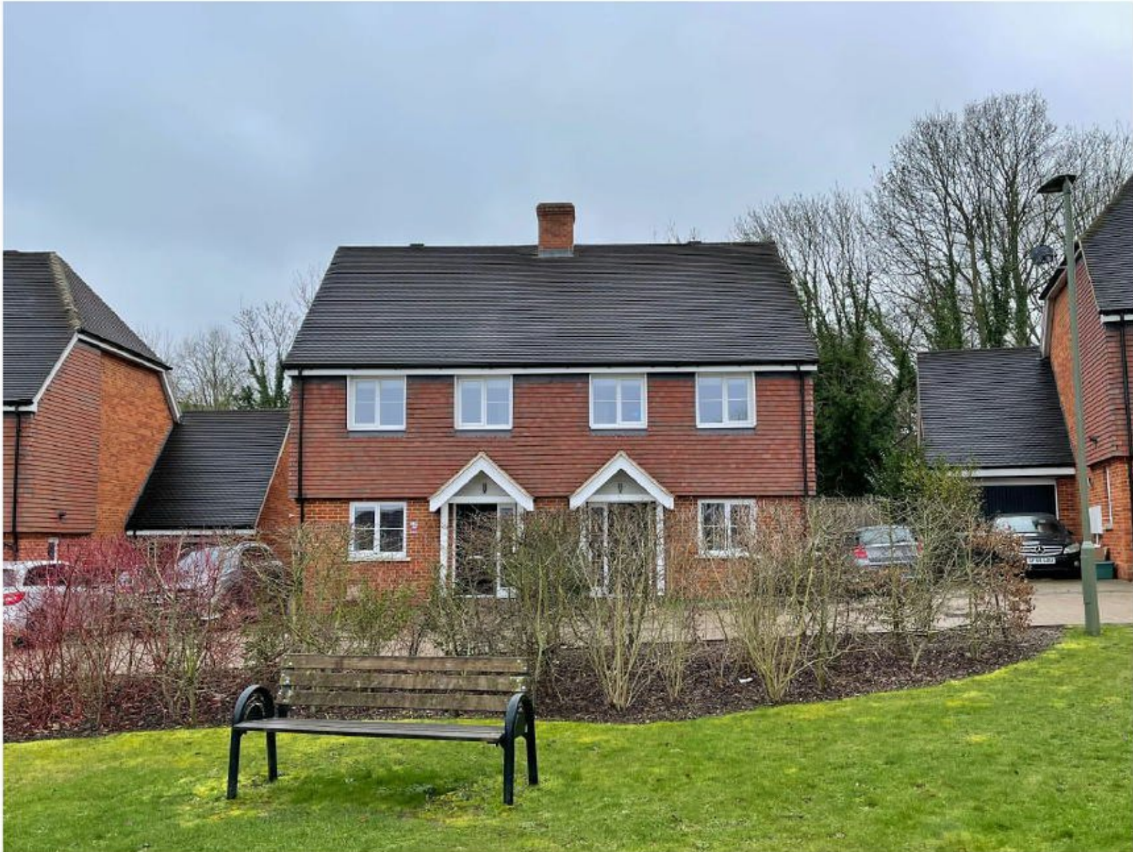
Front roadside view of property
