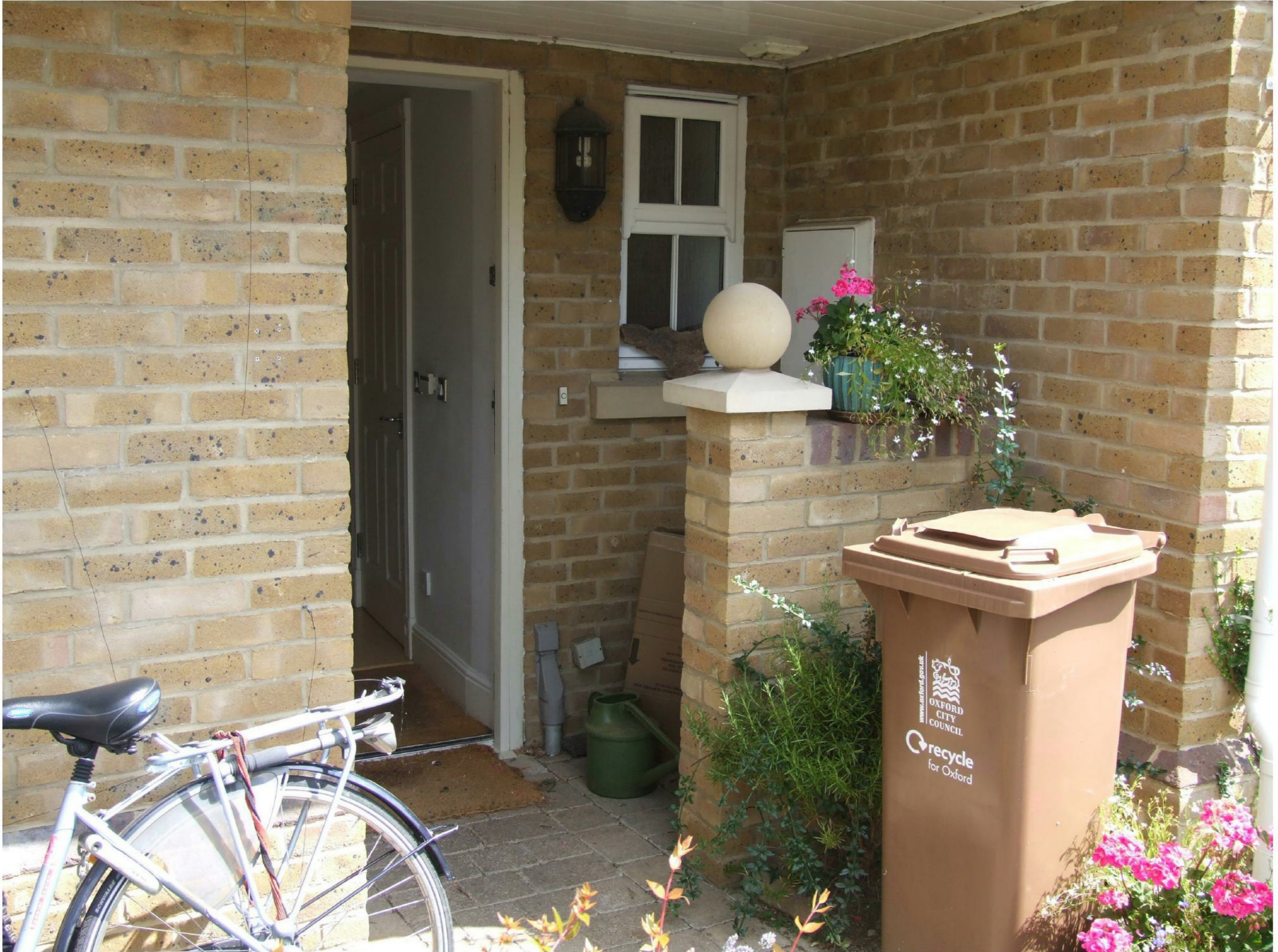
09 Similar dwelling in Burgess Mead showing typical arrangement of existing bin area.
