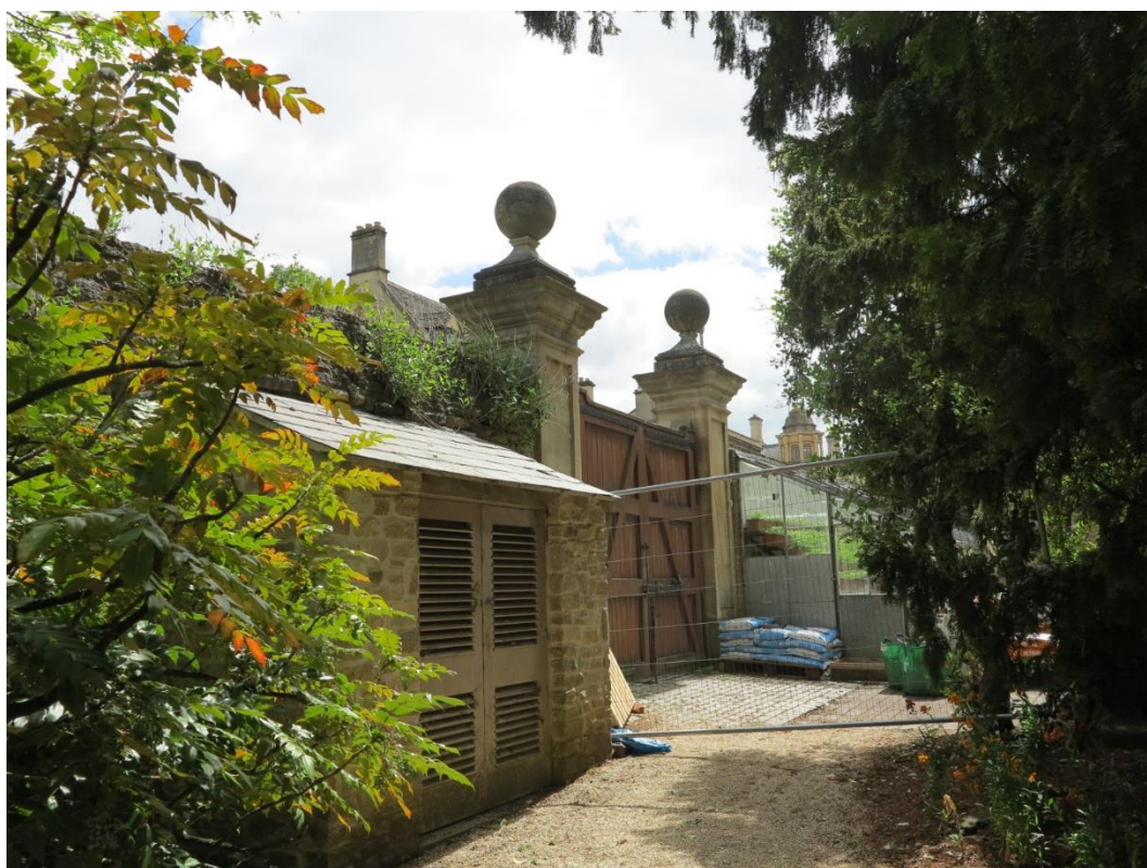
Plate 2. The existing gas utility building
