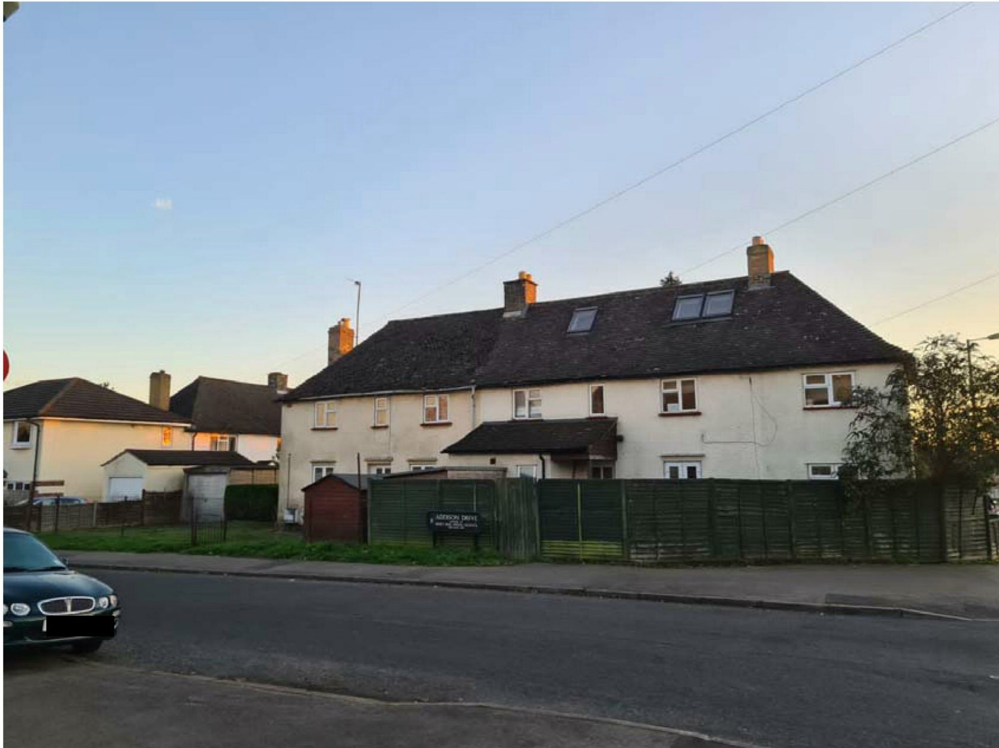
View of rear elevation from Addison Drive with No. 112 and side extension to right.
