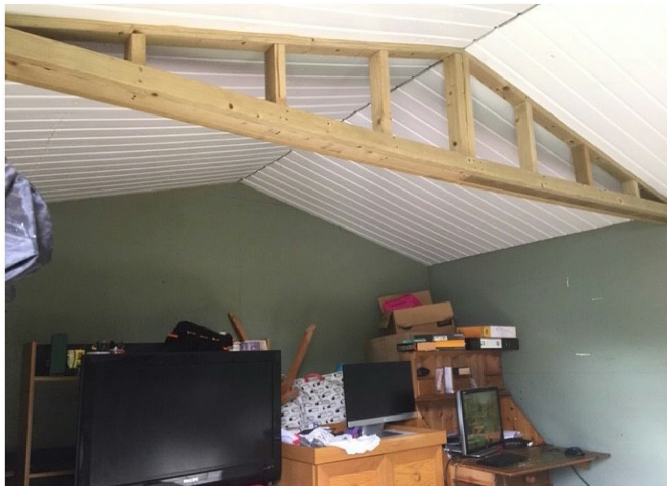
No. 42 Outbuilding (Proposed Mini Gym) – Interior View
