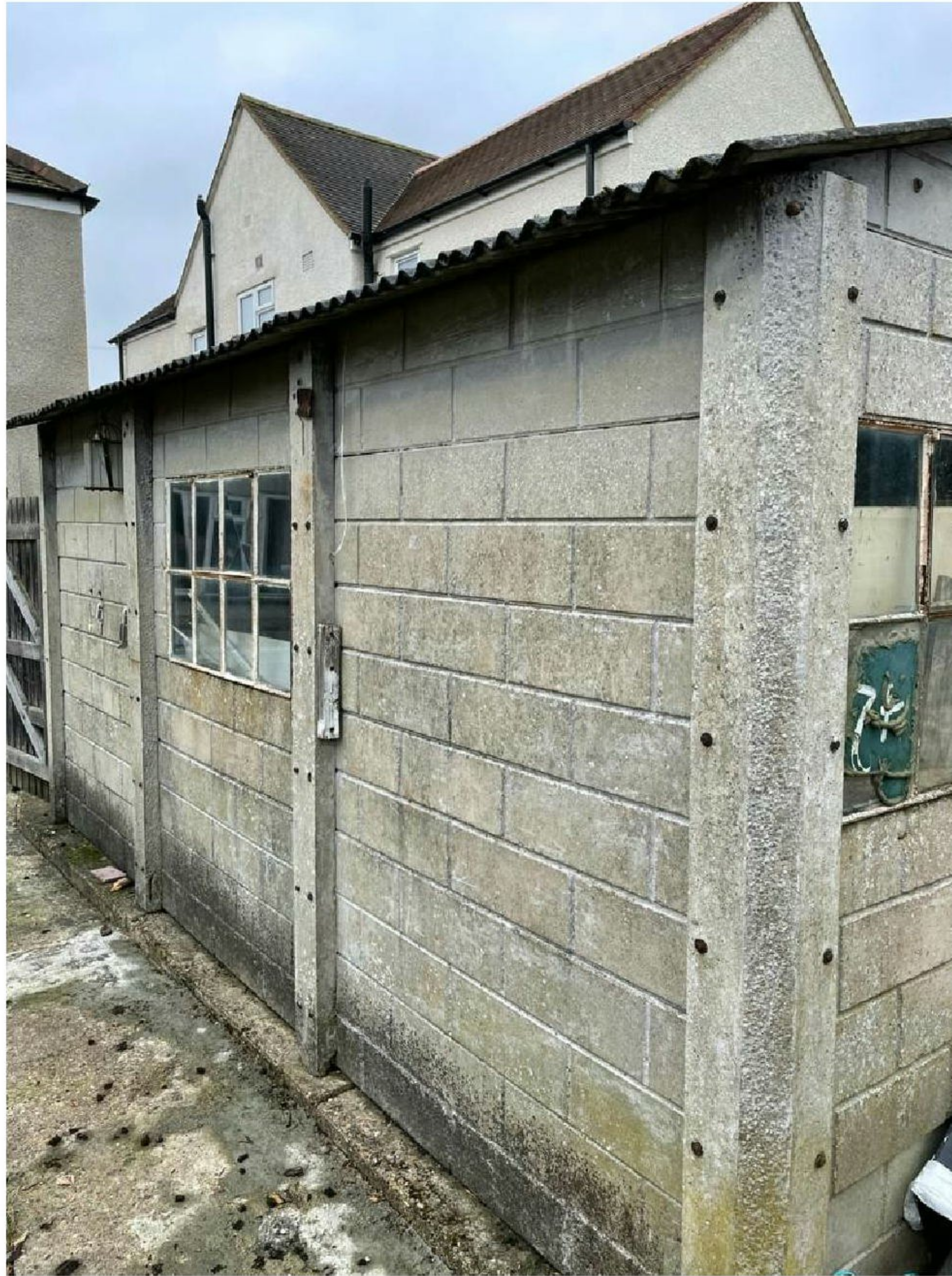
No. 42 Garage - Rear Corner View
