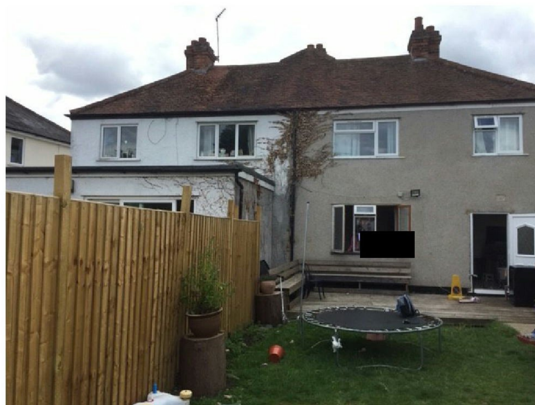
No. 40 and 42 Main Dwelling - Rear View
