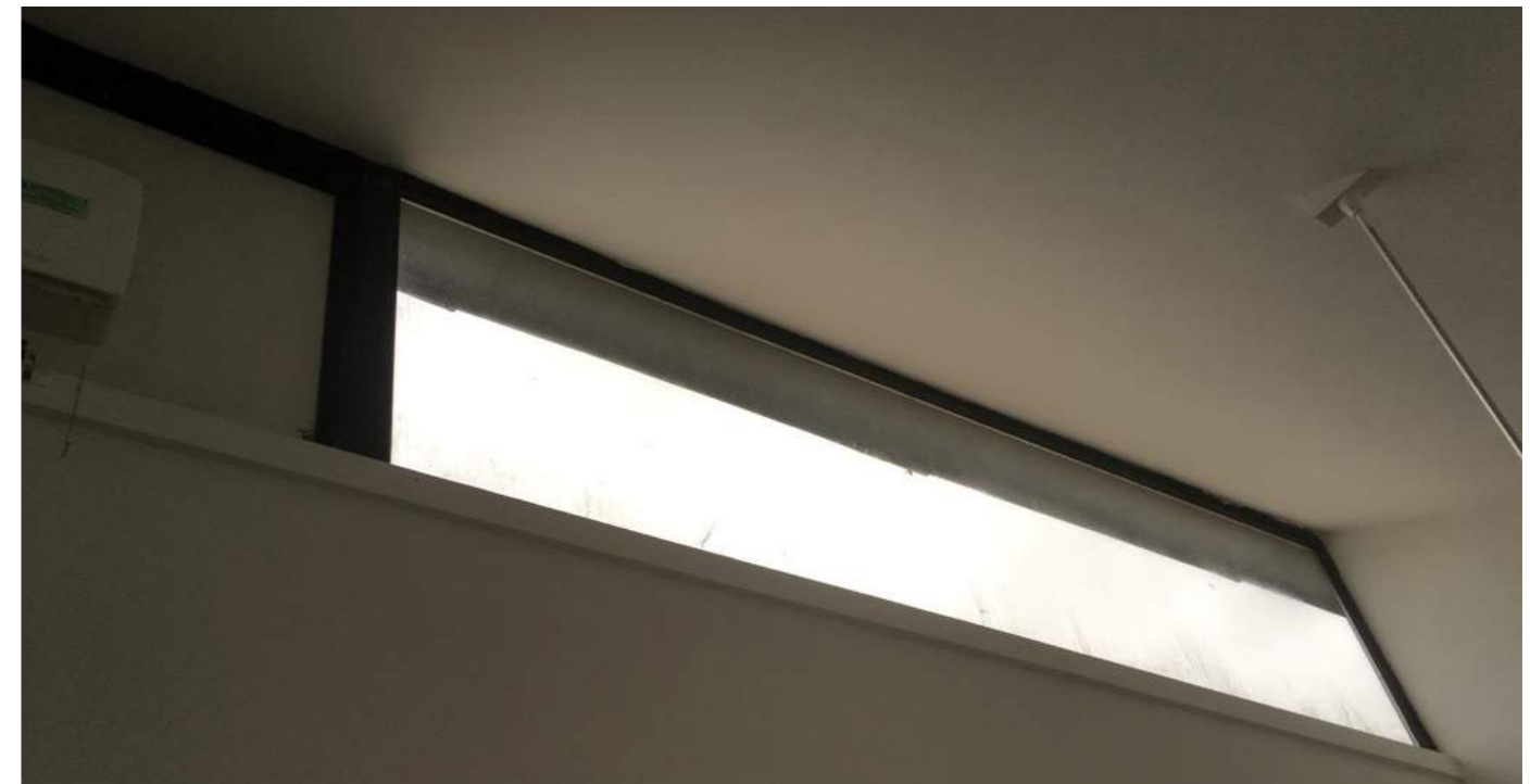
Type 4 & 5 - Interior view of F,G,H-Block
