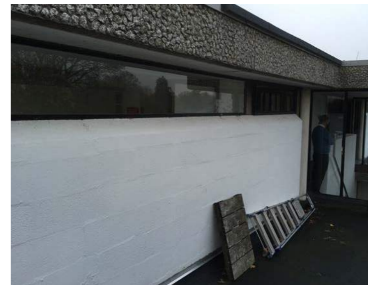
Type 8a - Exterior view - Penthouse
