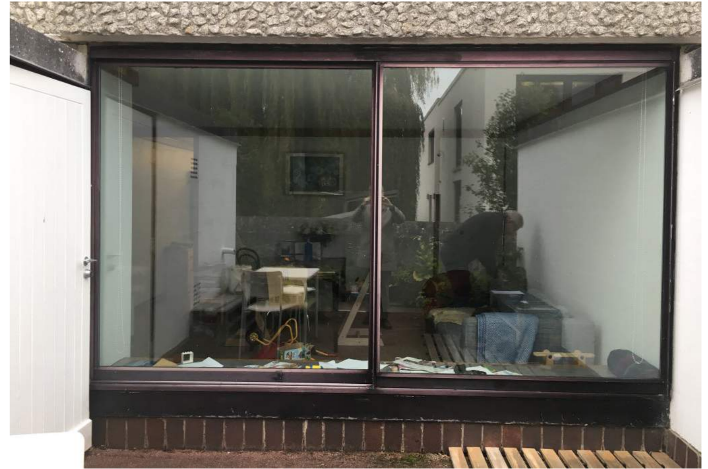
Type 1a - Exterior view of F, G, H-Block
