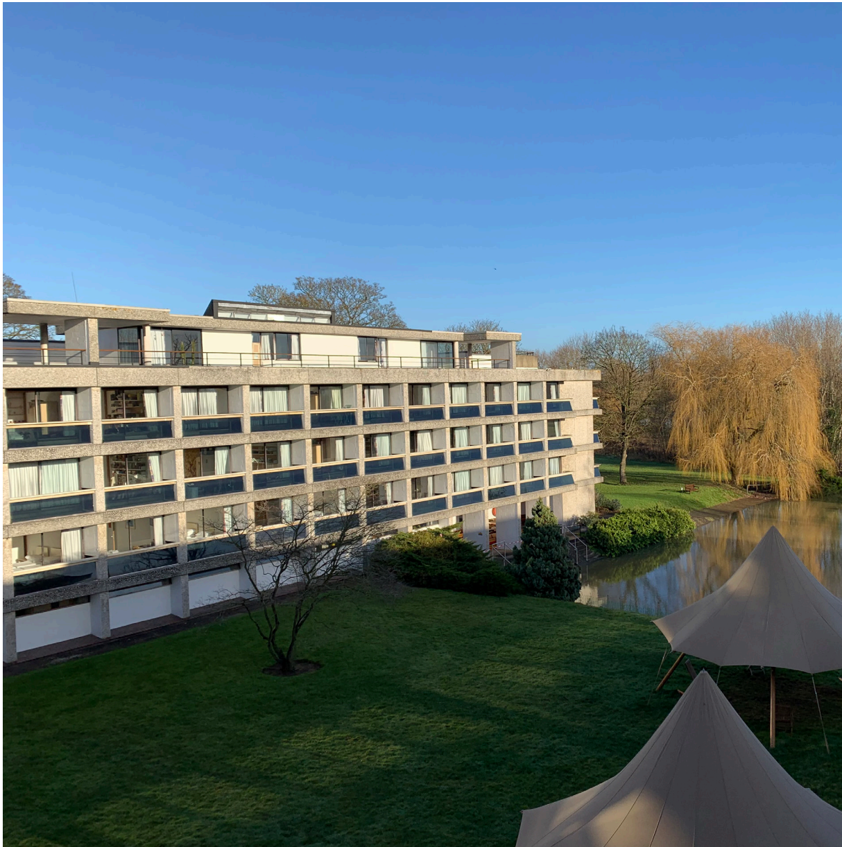
Fig 2. View of C Block
