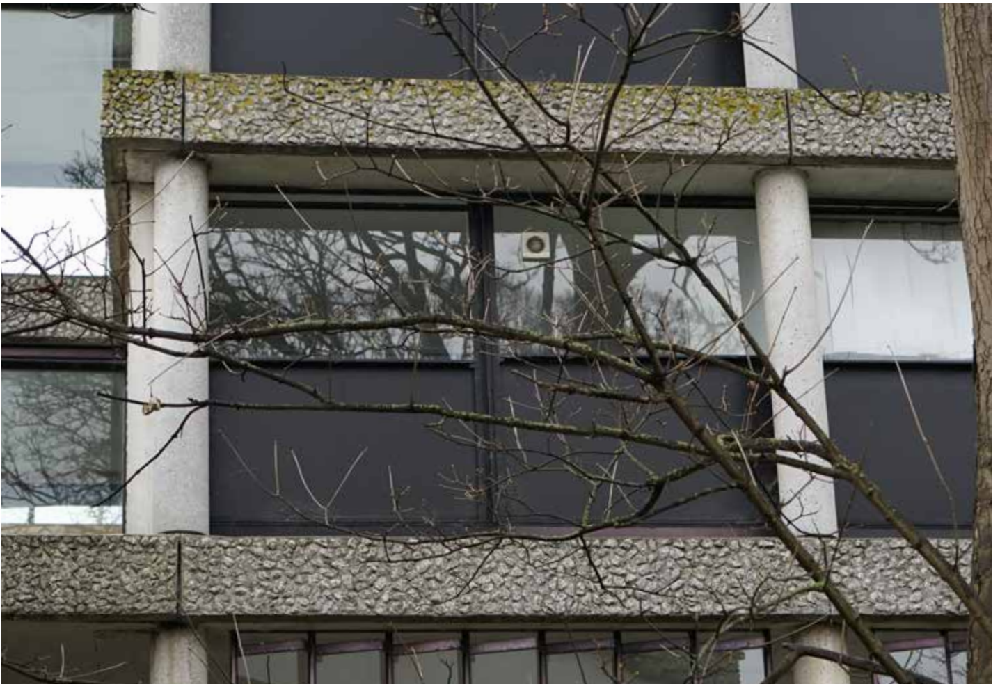
Full height vertical sliders, lower original Powell and Moya panels of black to shield kitchen or bathroom units at second and third floors.
