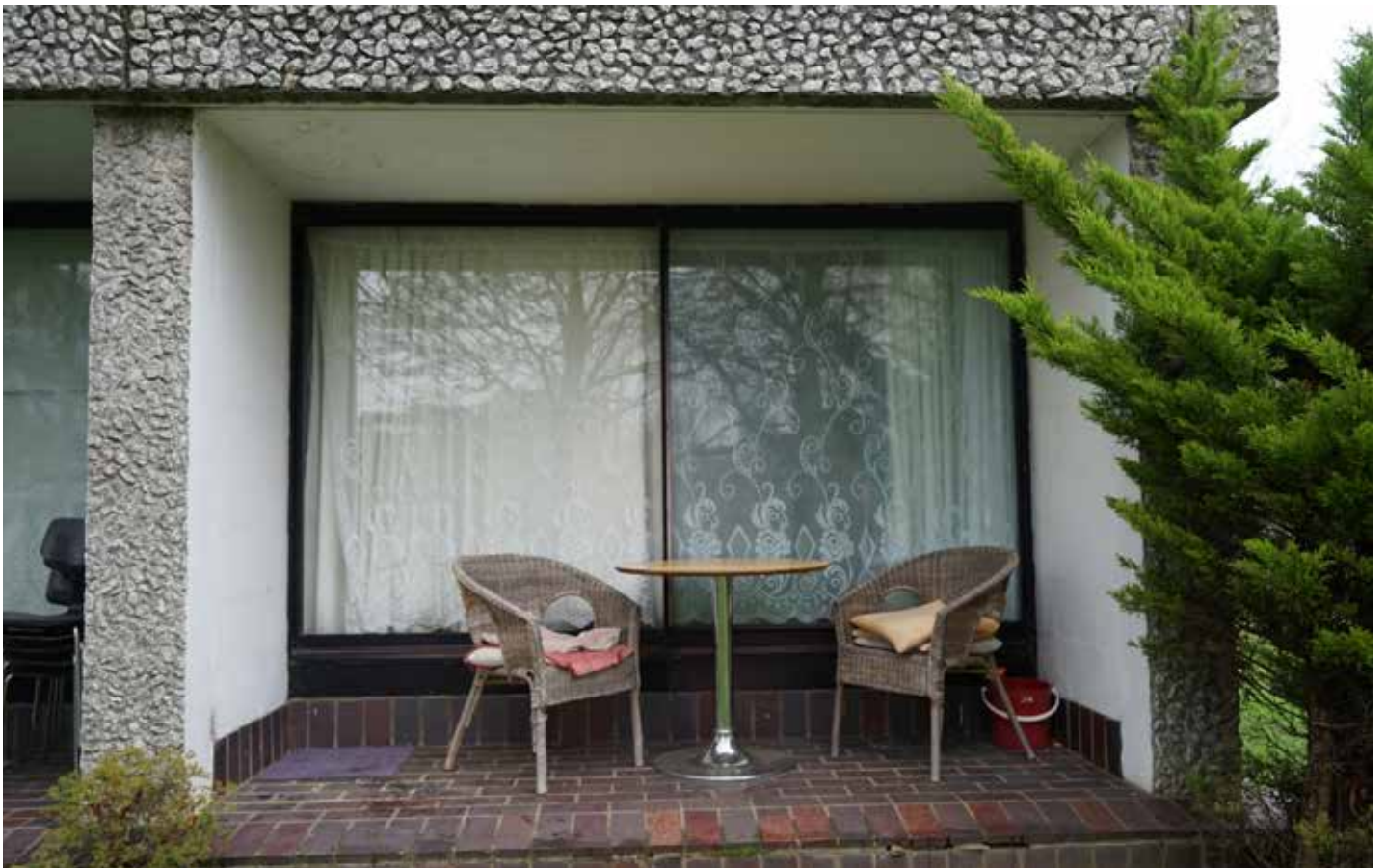
Full height, bay width horizontal sliding panes forming doors to quad and balconies at all levels.
