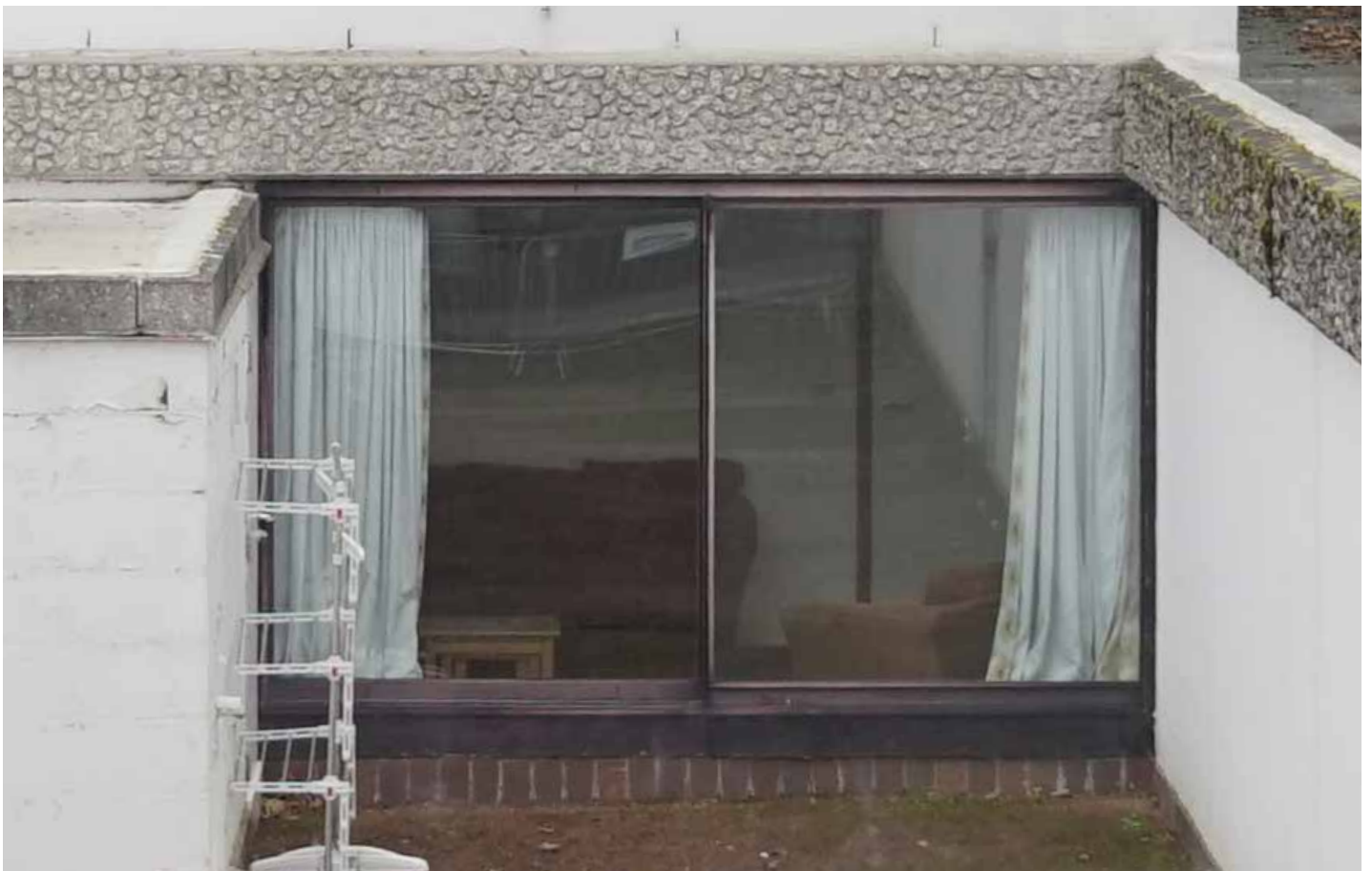
G Block – Living rooms H Block – Living rooms
