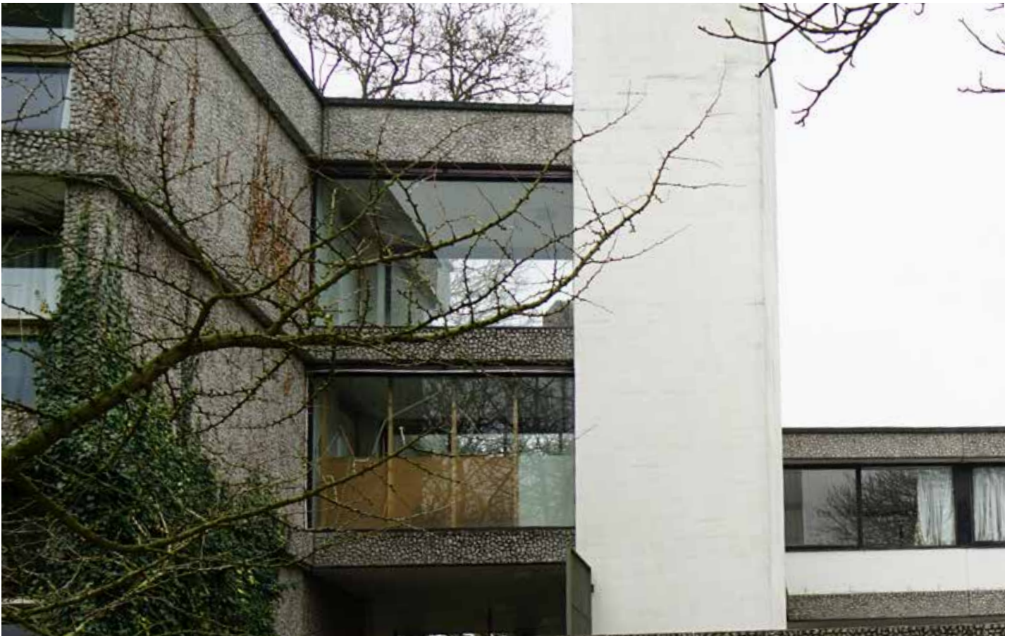
Full height bay width fixed pane at second and third floors, connecting to elevator shafts.
