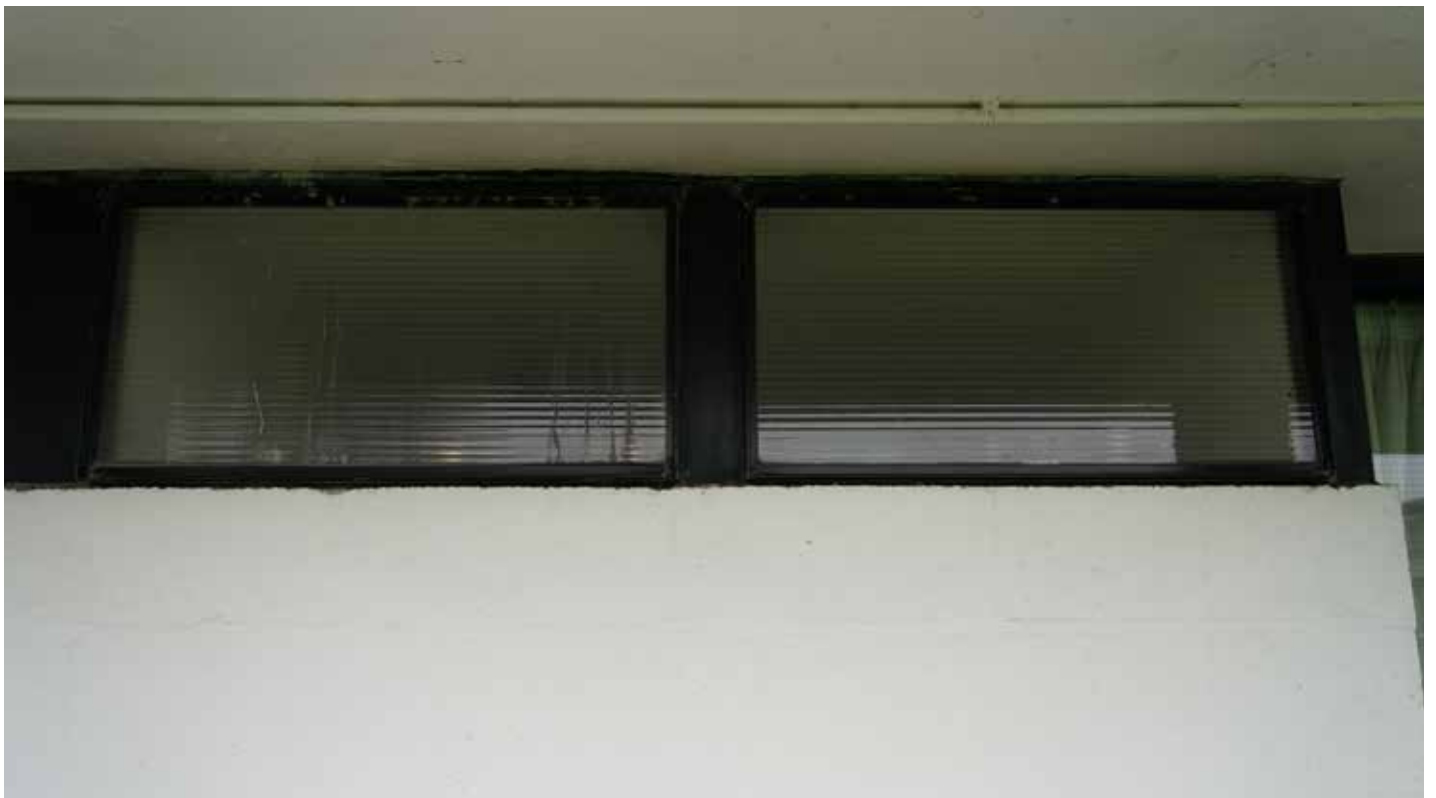
Half bay width top hung openings at ground level serving toilet/bathrooms
