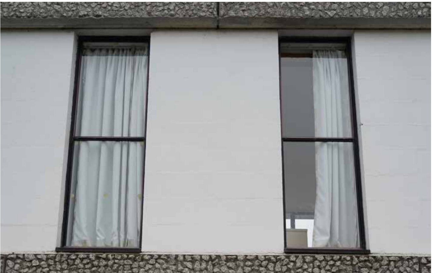
Single vertical slider above walkthrough, overlooking promenade.
