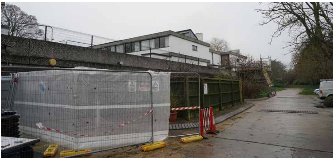
H Block – First floor overlooking the northern promenade
