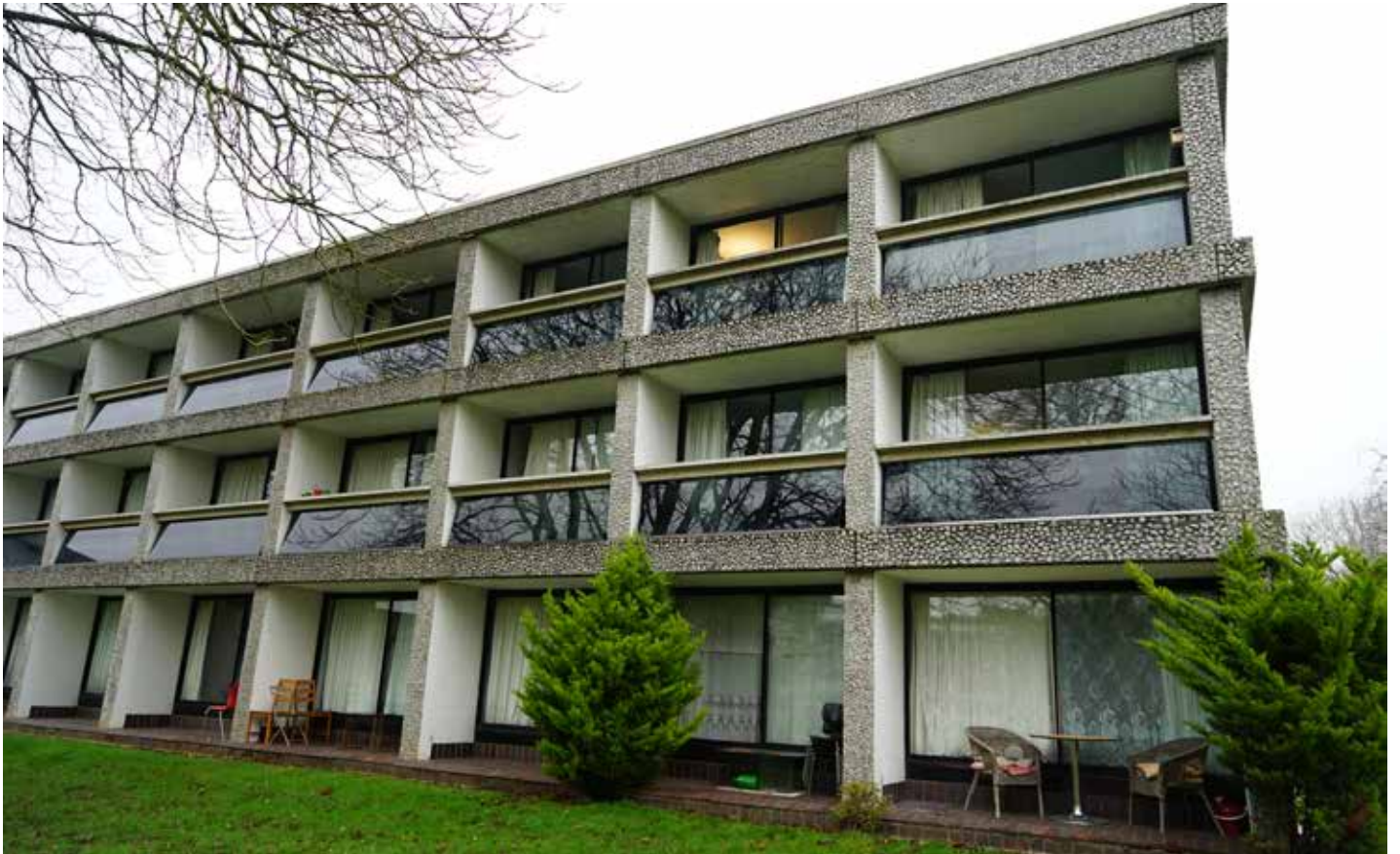
Full height, bay width horizontal sliding panes forming doors to quad and balconies at all levels.
