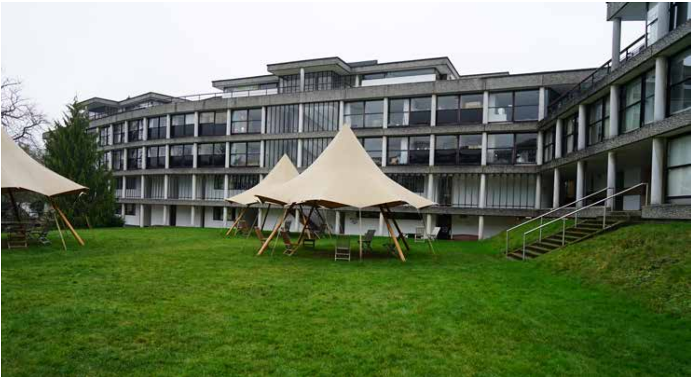
C Block – 1st and 2nd floor communal spaces
