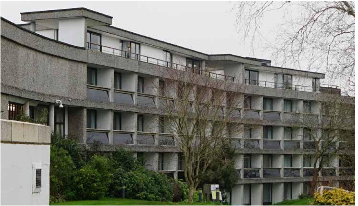
C Block – Single study bedspaces, one-bed flats living rooms and bedrooms, penthouse wrapped around corner.
