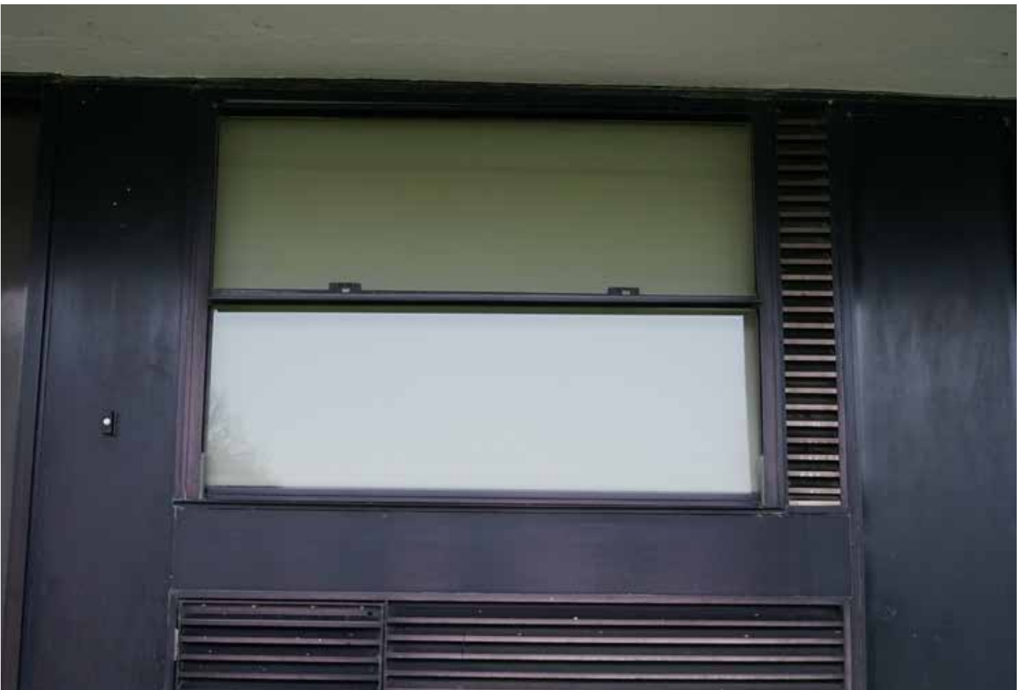
Half height vertical sliders with aluminium fixed louvres on the ground floor. Beneath them bay width aluminium louvred panels with opening panel to serve kitchen refuse bins.
