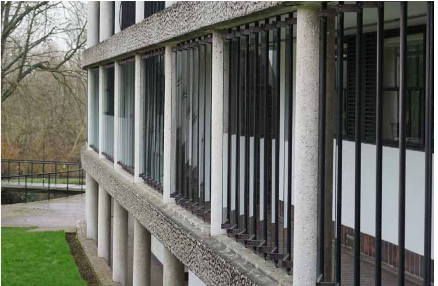
Full height panes in louvred fixed aluminium frames
