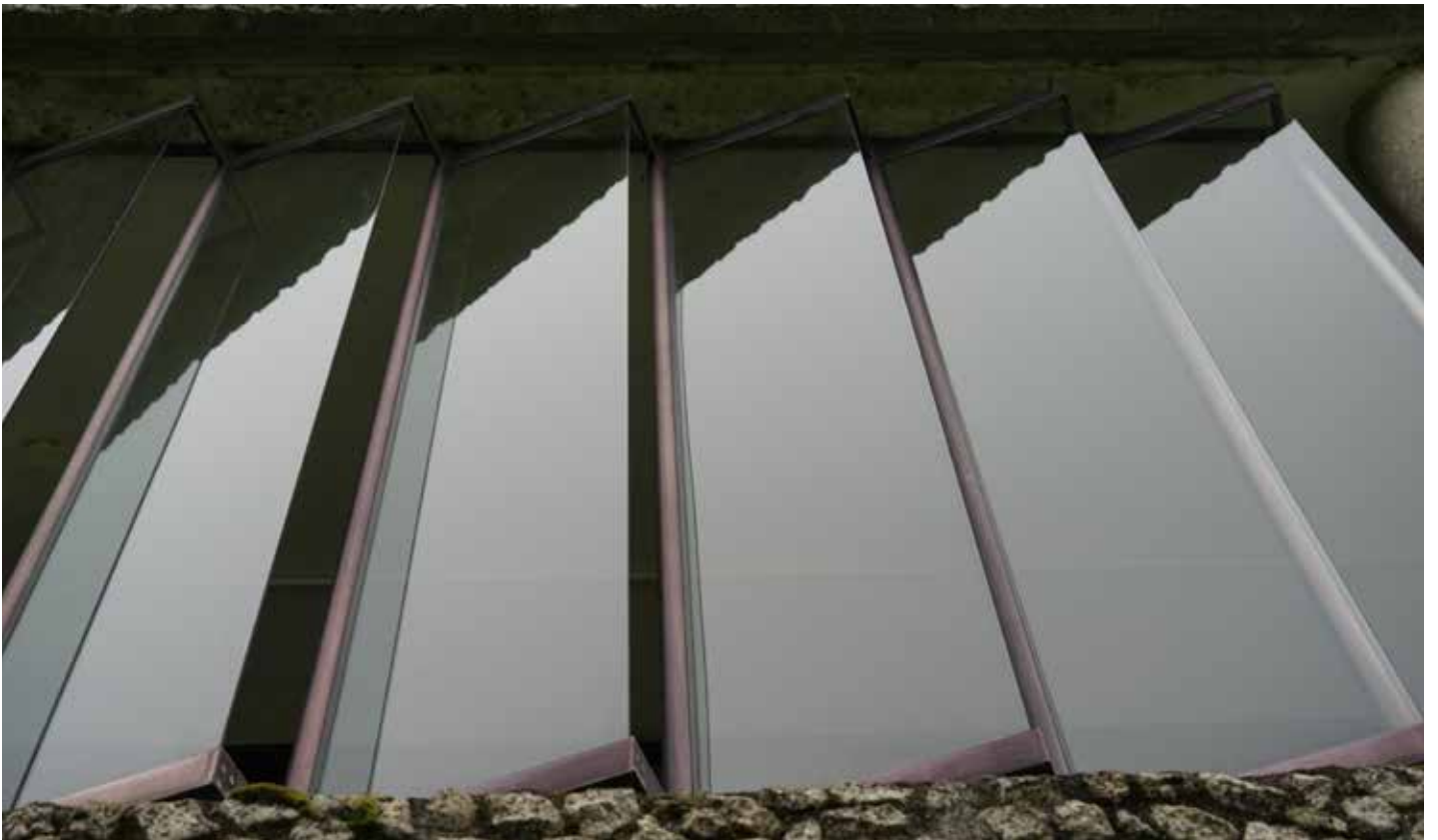
Half height vertical sliders with aluminium fixed louvres on the ground floor. Beneath them bay width aluminium louvred panels with opening panel to serve kitchen refuse bins.
