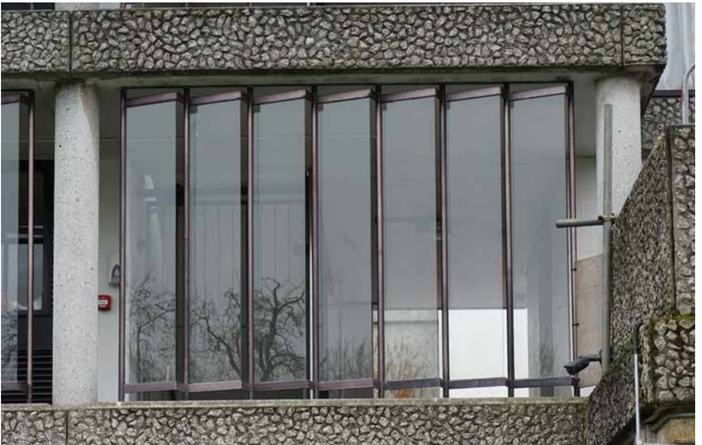
Full height fixed panels in louvred aluminium frames at first and second floors offering protection of corridor
