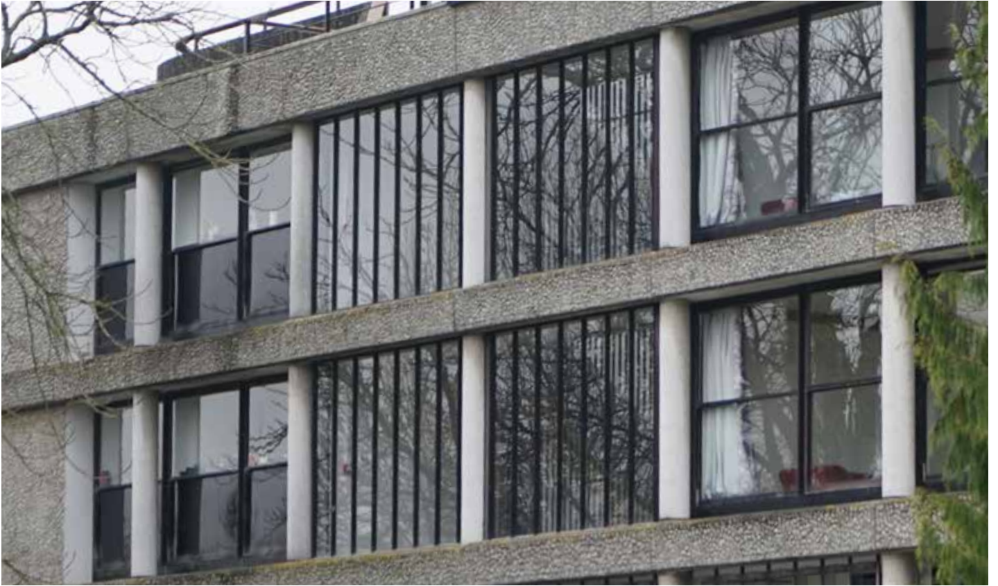
Full height rectangular pane in aluminium frames
