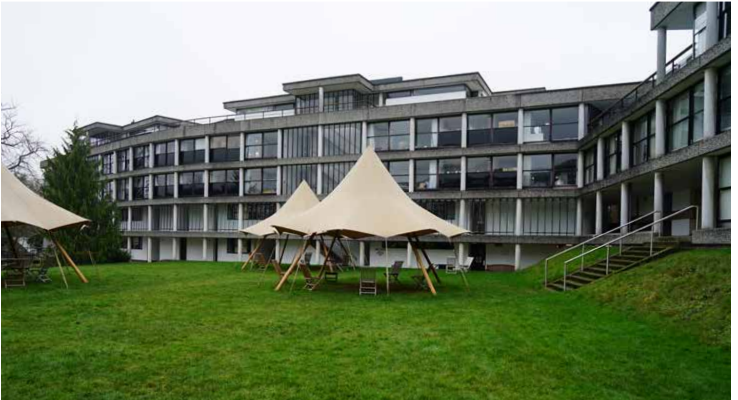
Full height vertical sliders, lower panes of kitchen or bathrooms painted black on the reverse to shield units.
