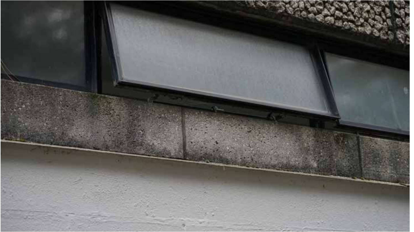
Top hung large pane opening at south east corner
