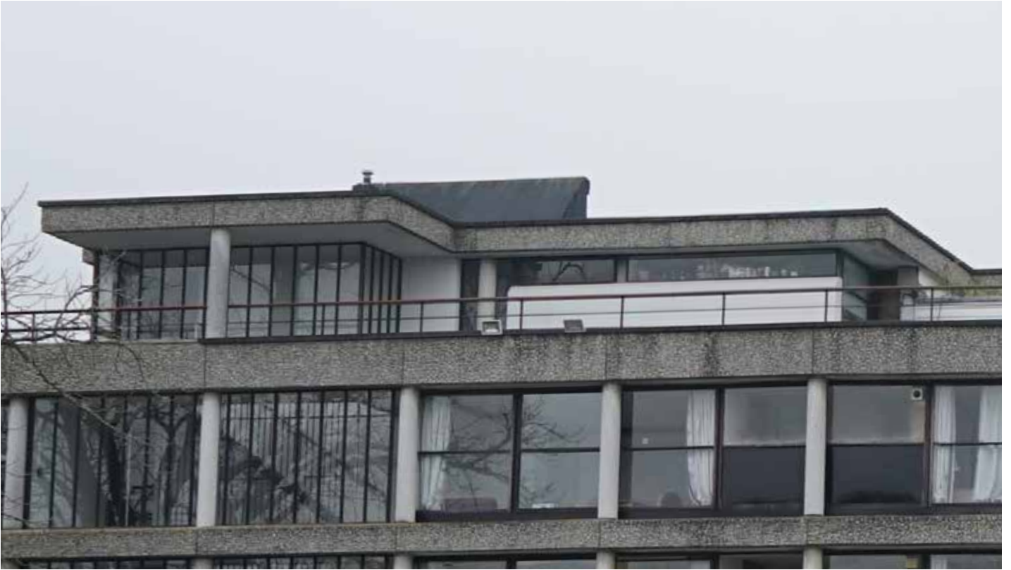
Double bay width top hung opening at penthouse level.
