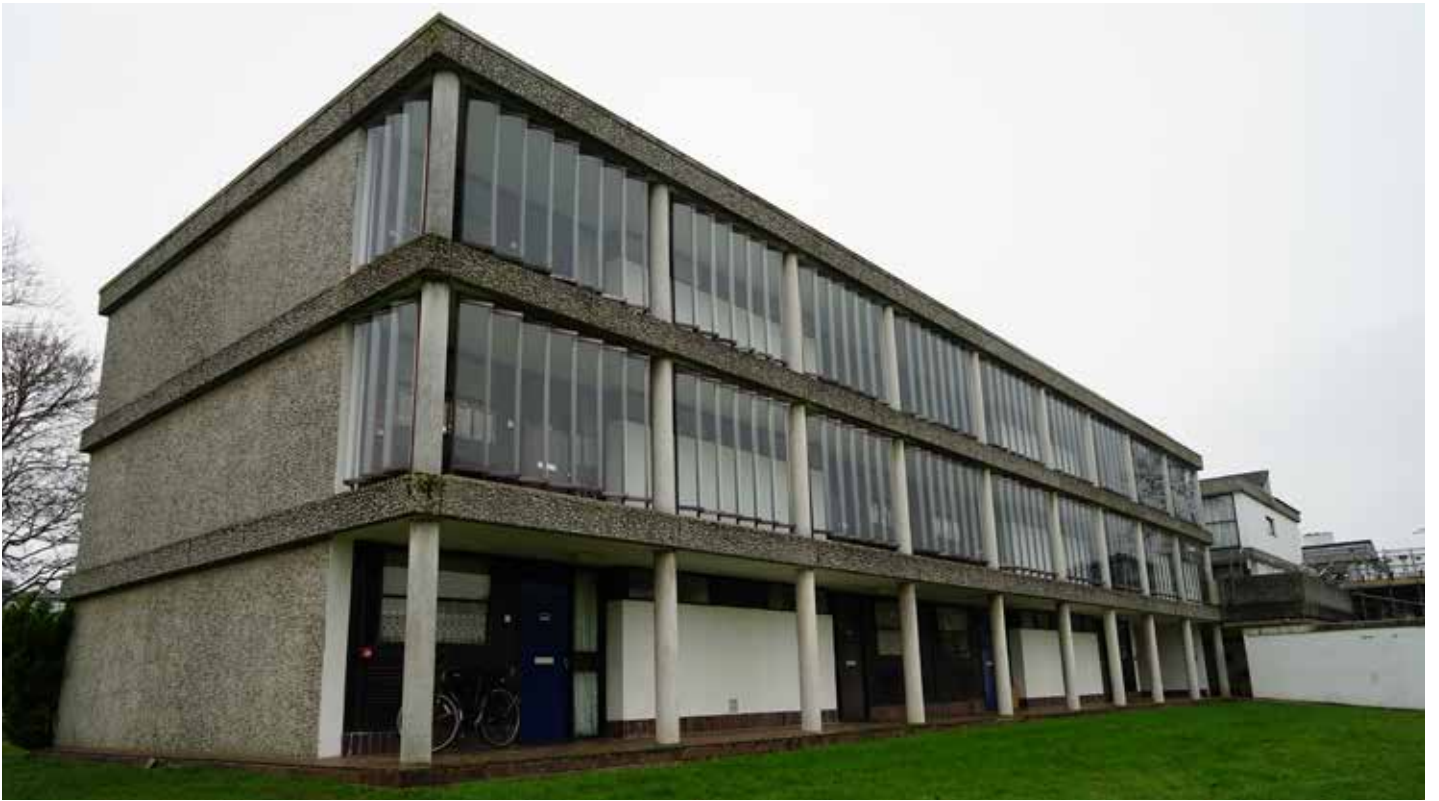
Full height fixed panels in louvred aluminium frames at first and second floors offering protection of corridor
