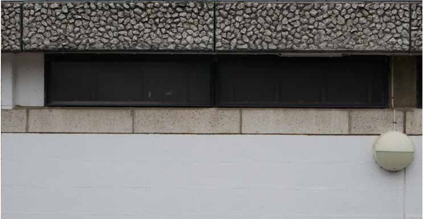
Half bay width top hung single pane openings with mitred protruding L bracket
