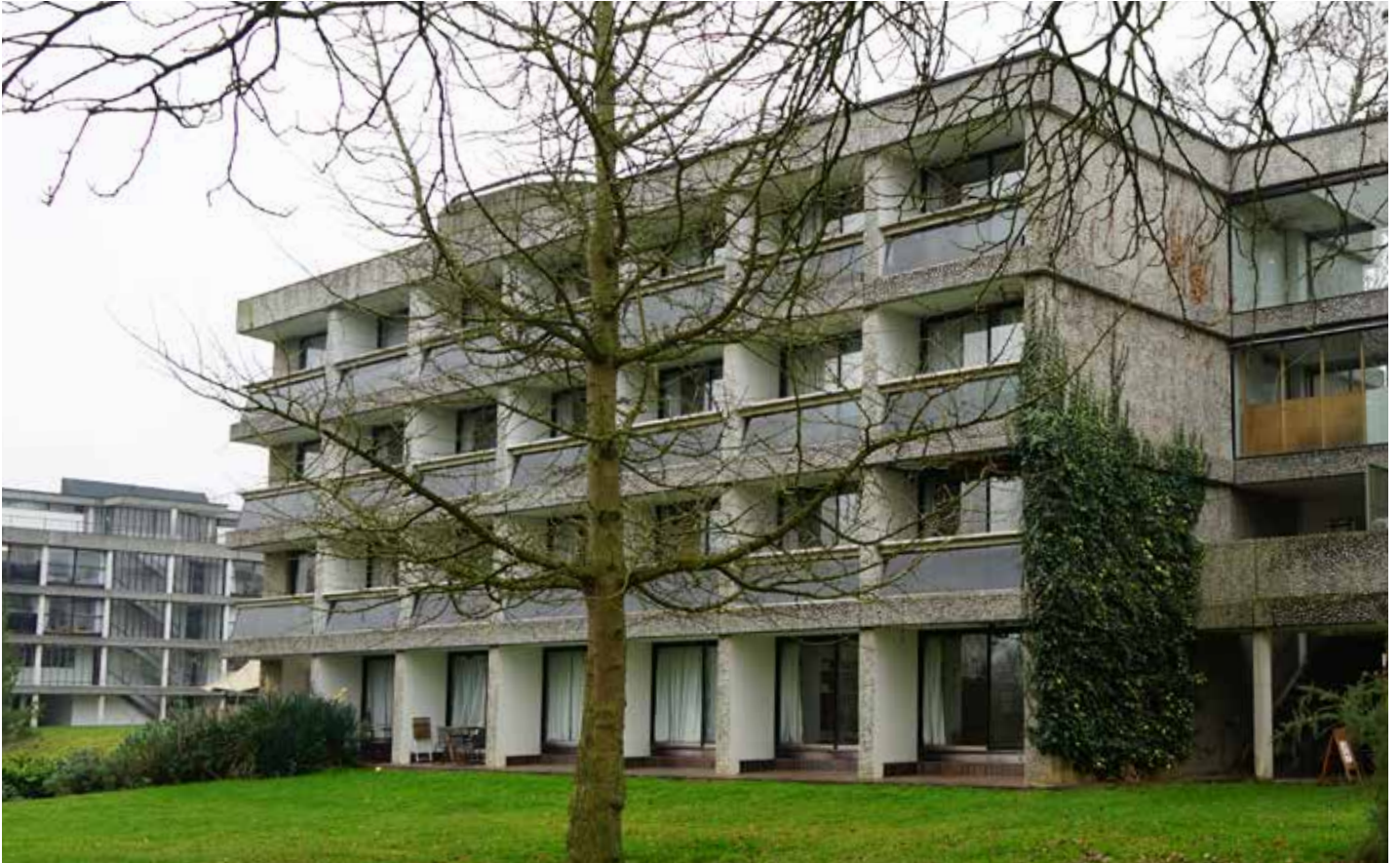
Full height horizontal sliding double doors on balconies at all levels of east elevation
