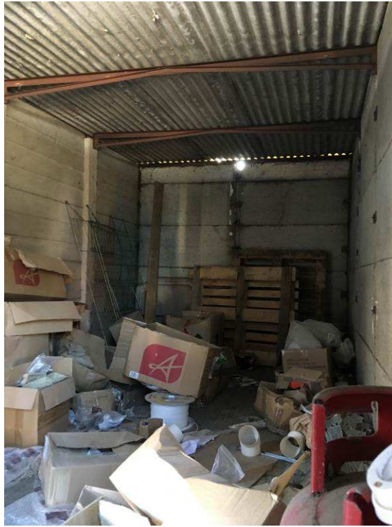
Plate 3 – Internal view of one of the garages.
