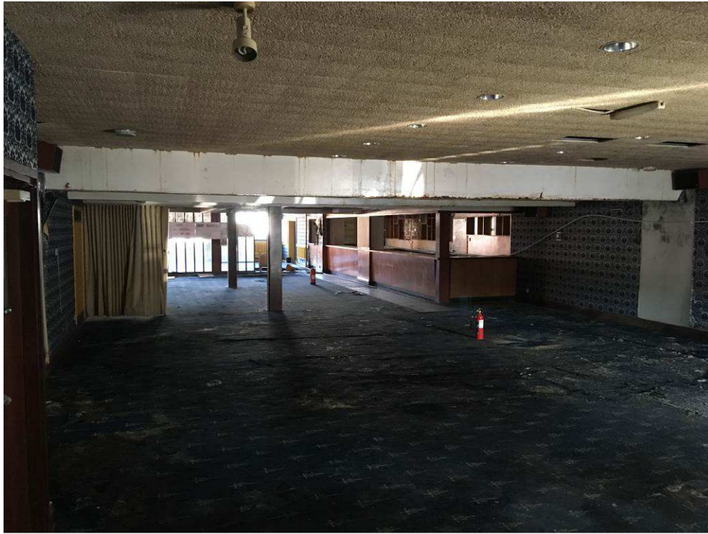
Plate 9 – Internal view of southern section of Cowley Conservative Club, looking west.
