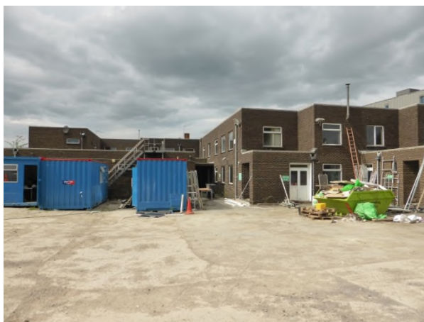
Figure 24: Rear elevation of the 1970s extensions
