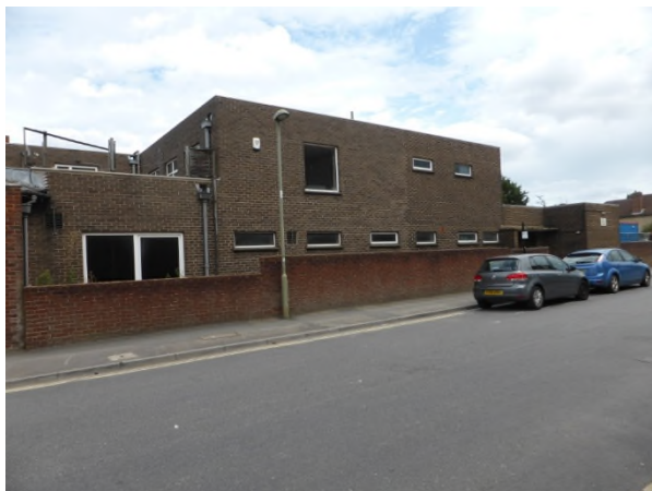
Figure 21: Early 1960s single storey entrance and 2-storey extension viewed from St Lukes Road (centre and left of the image)
