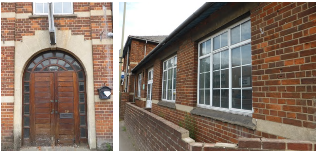
Figures 9 and 10: Main entrance with stone dressings and a later door (left) and stone bands, sills, lintels and double glazed windows on the front elevation (right)
