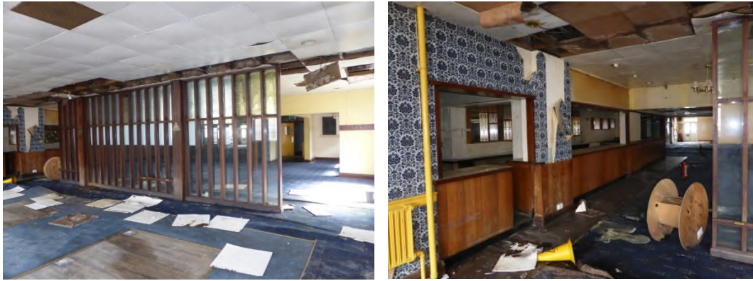
Figures 29 and 30: Glazed wooden screen in the extended Lounge (left) and bar to the extended Lounge (right)
