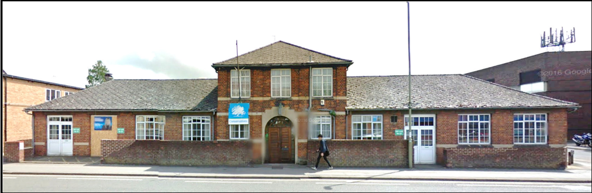
Figure 6. The west façade of the Conservative Club at No 19 (Google Earth).
