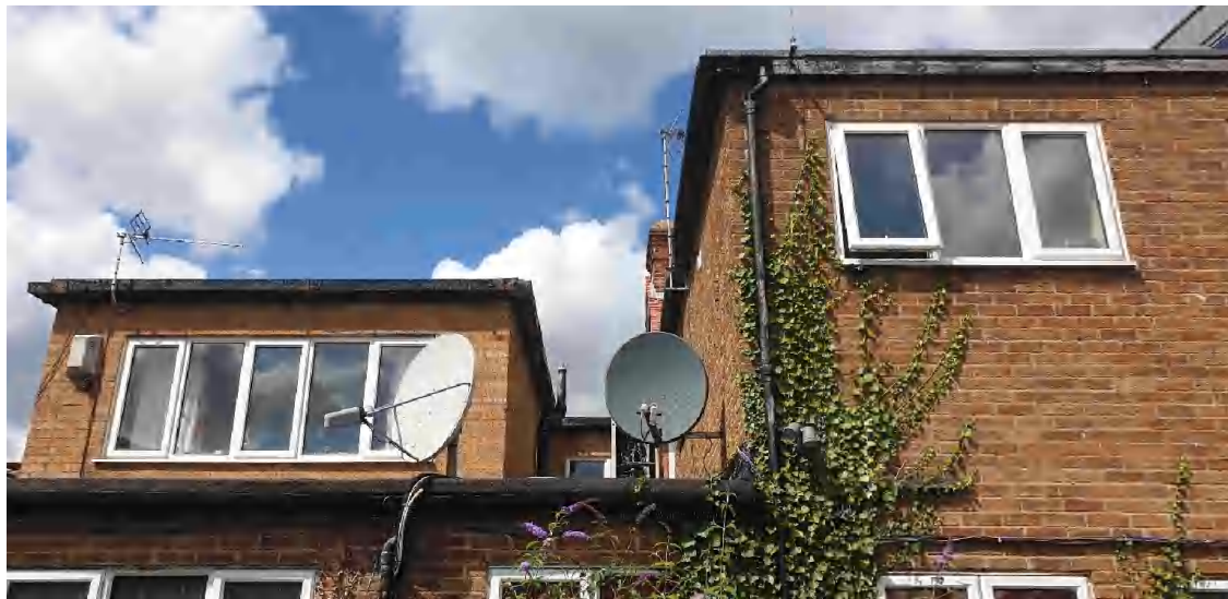
Photographs showing rear of no's 17/17b. The newly constructed Between Towns Court can be seen in the upper photograph.
