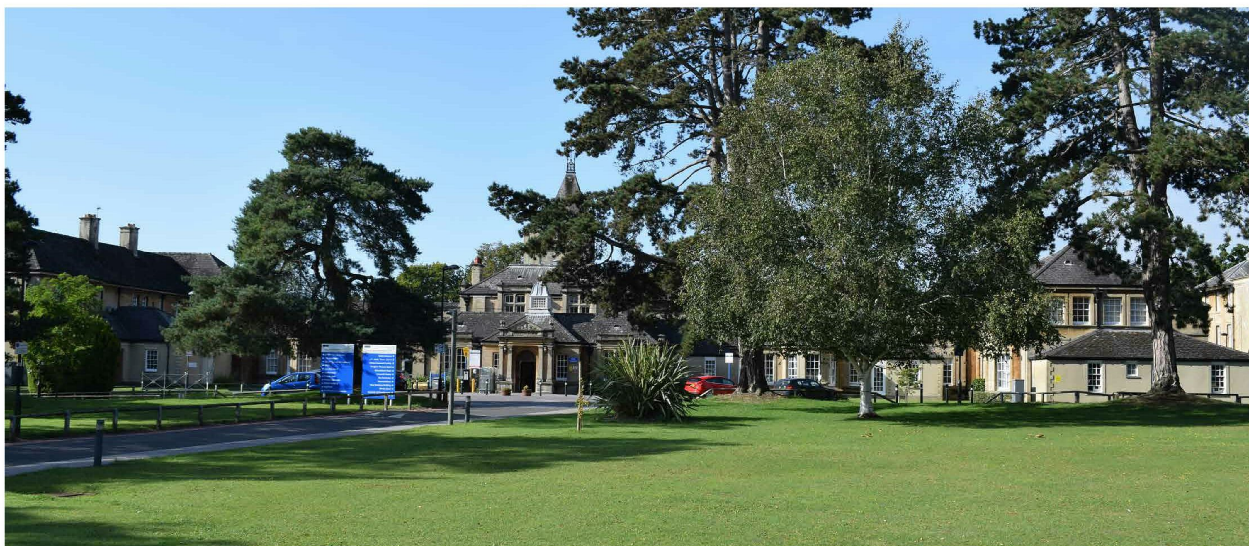
Current front entrance to the Warneford Hospital, in landscape setting with specimen trees
