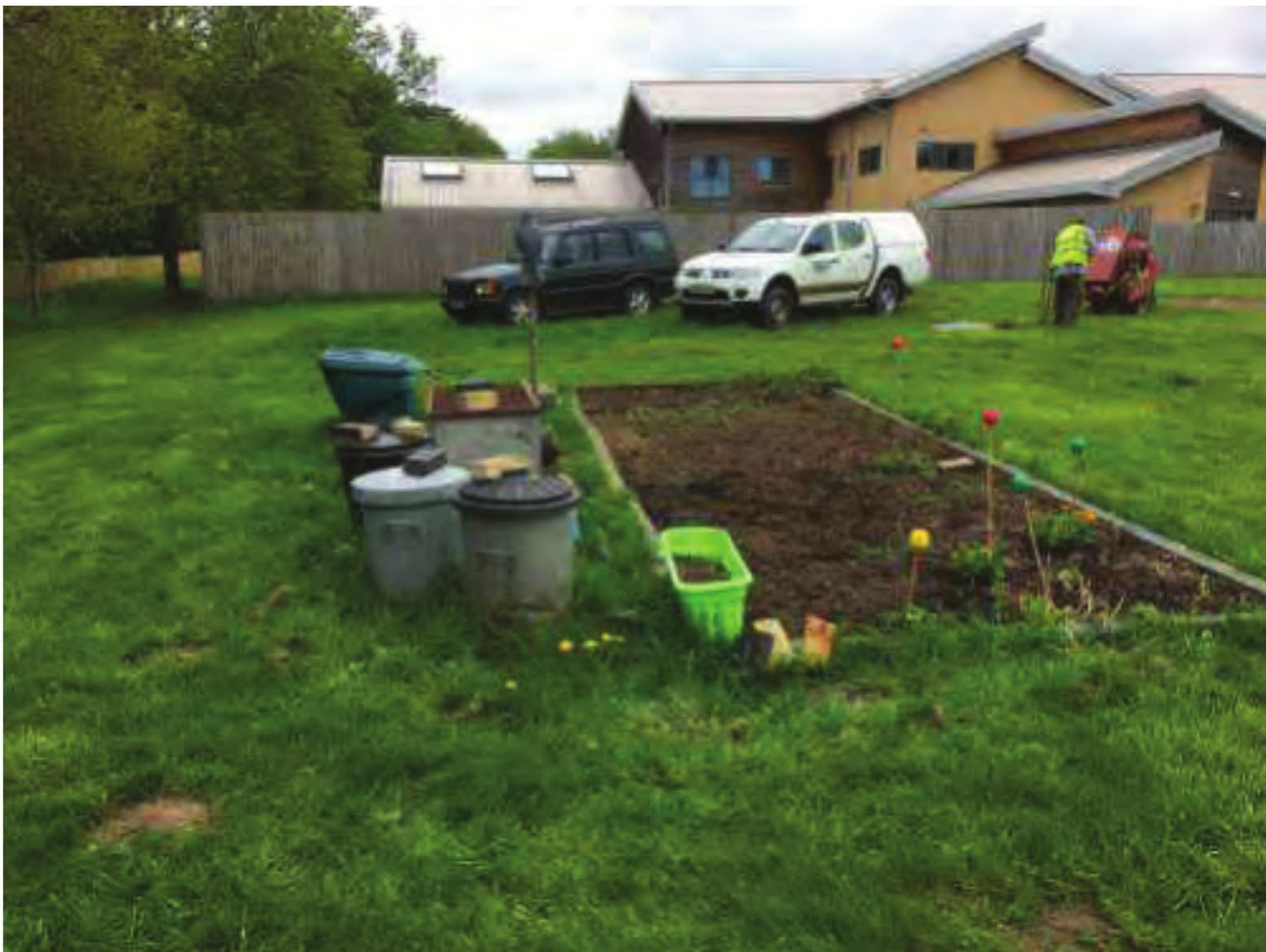
Site area from east
