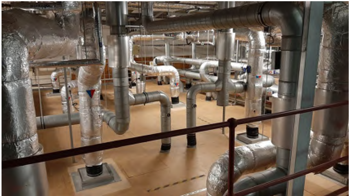
Plate 4 – Showing internal air conditioning ducting
