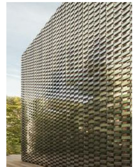
4 Ceramic Baguettes Decorative Rainscreen on Concrete Wall
