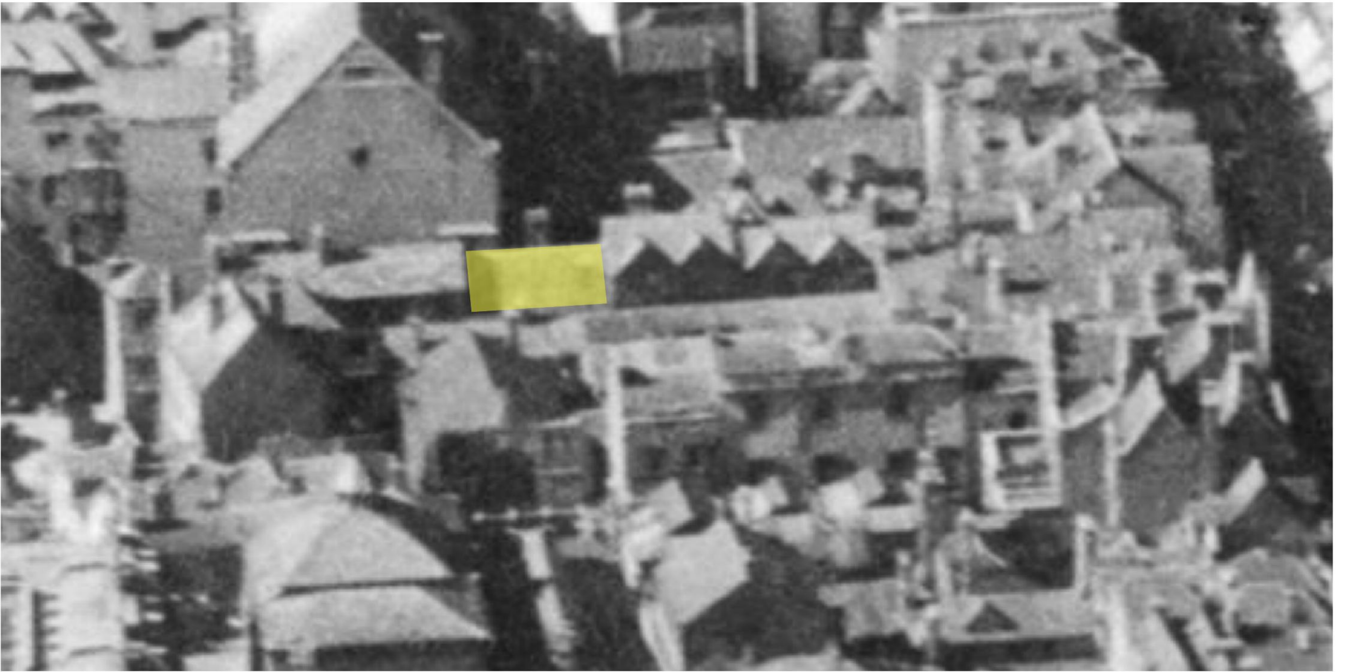
1949 aerial image from the east showing the roof of the Wheatsheaf PH and adjoining roofscape. The yellow dot is the area of roof proposed to be raised.
