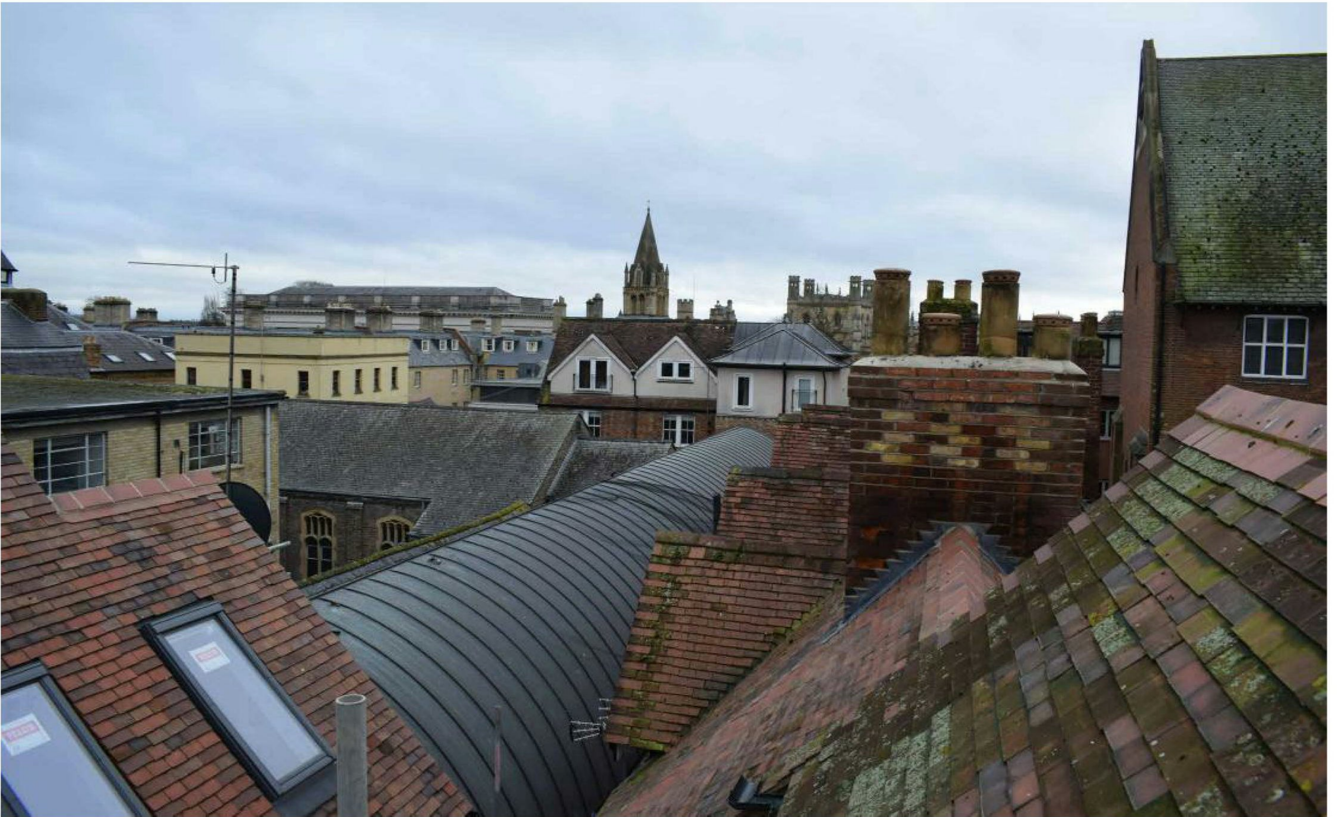
View of variety of adjoining roofs looking south
