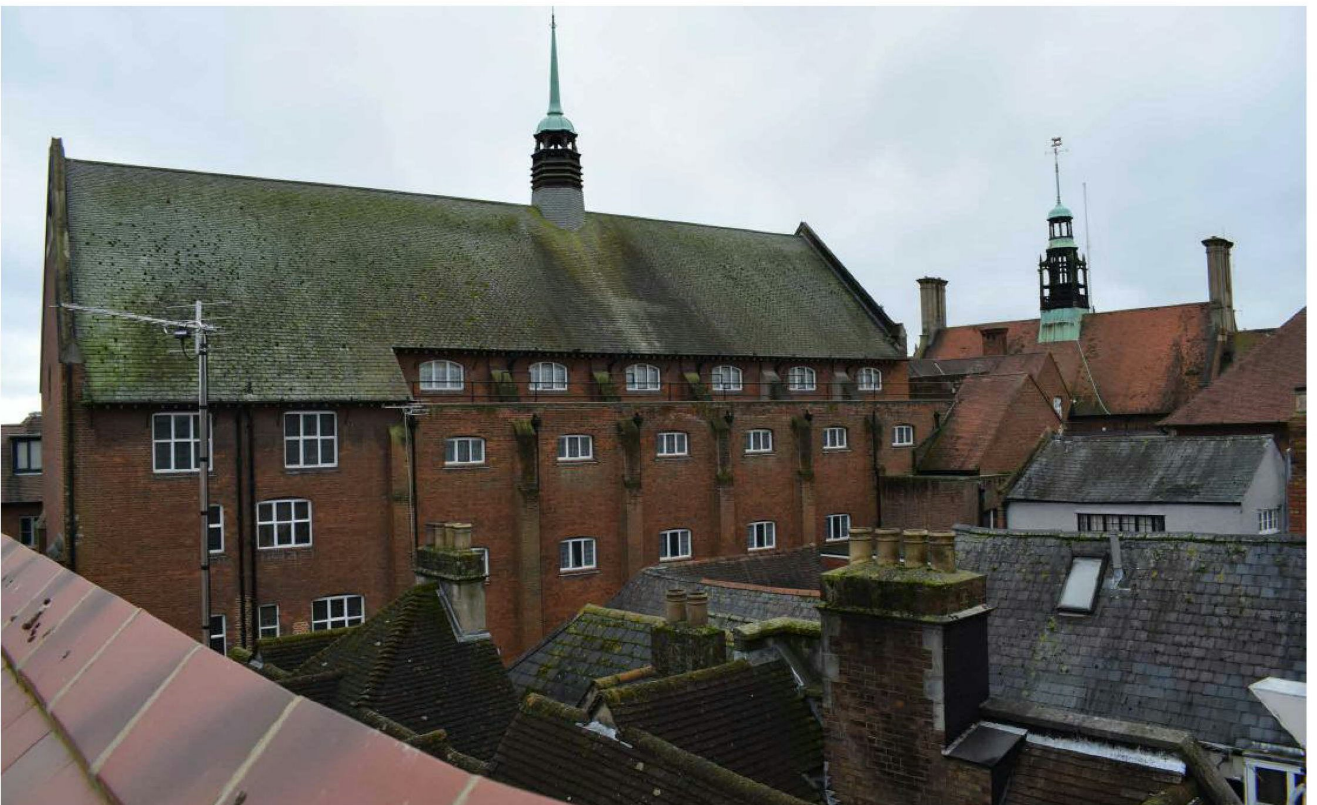
View of adjoining roofs to the south west
