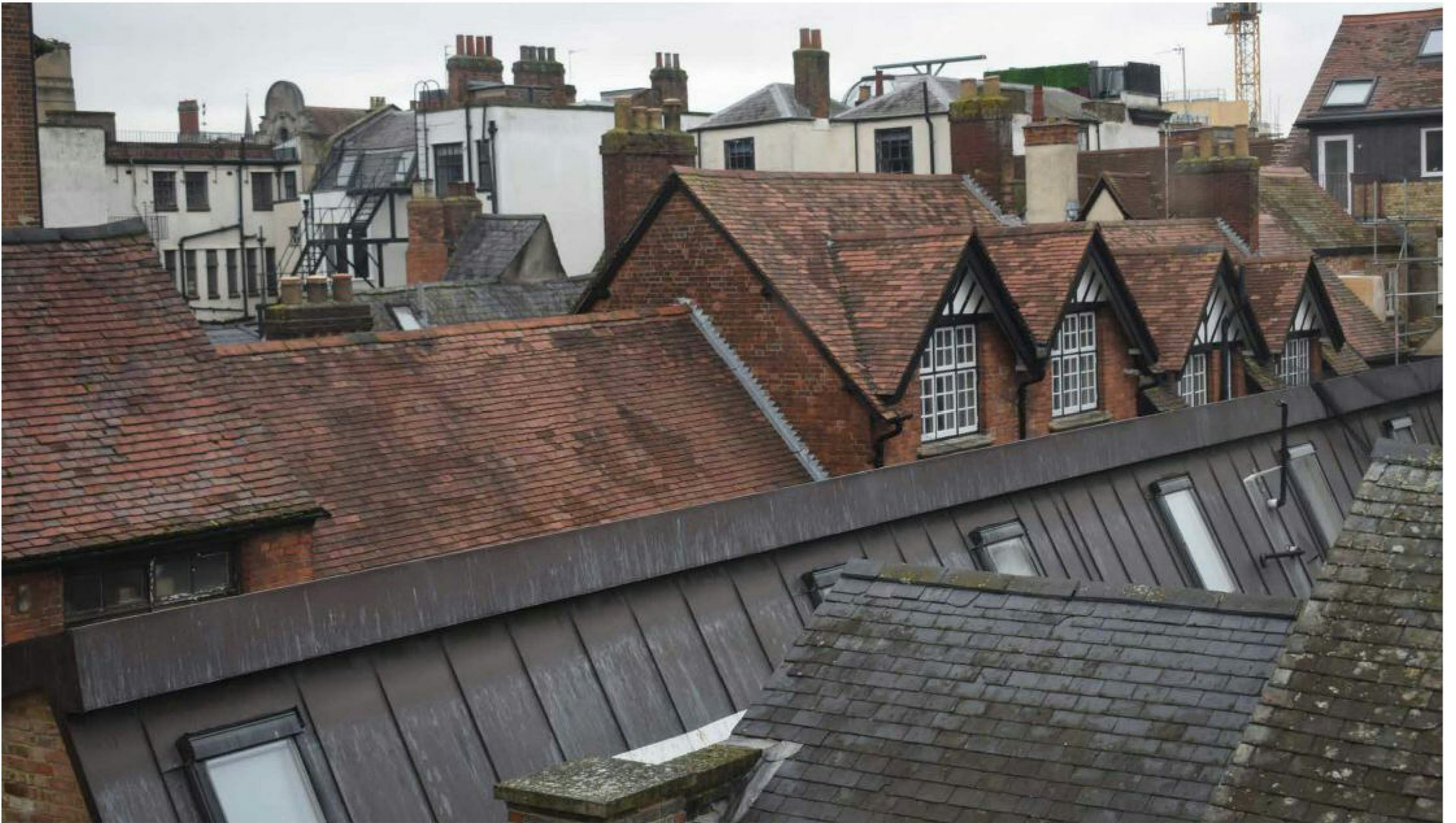
View of adjoining roofs looking north-west towards the High Street
