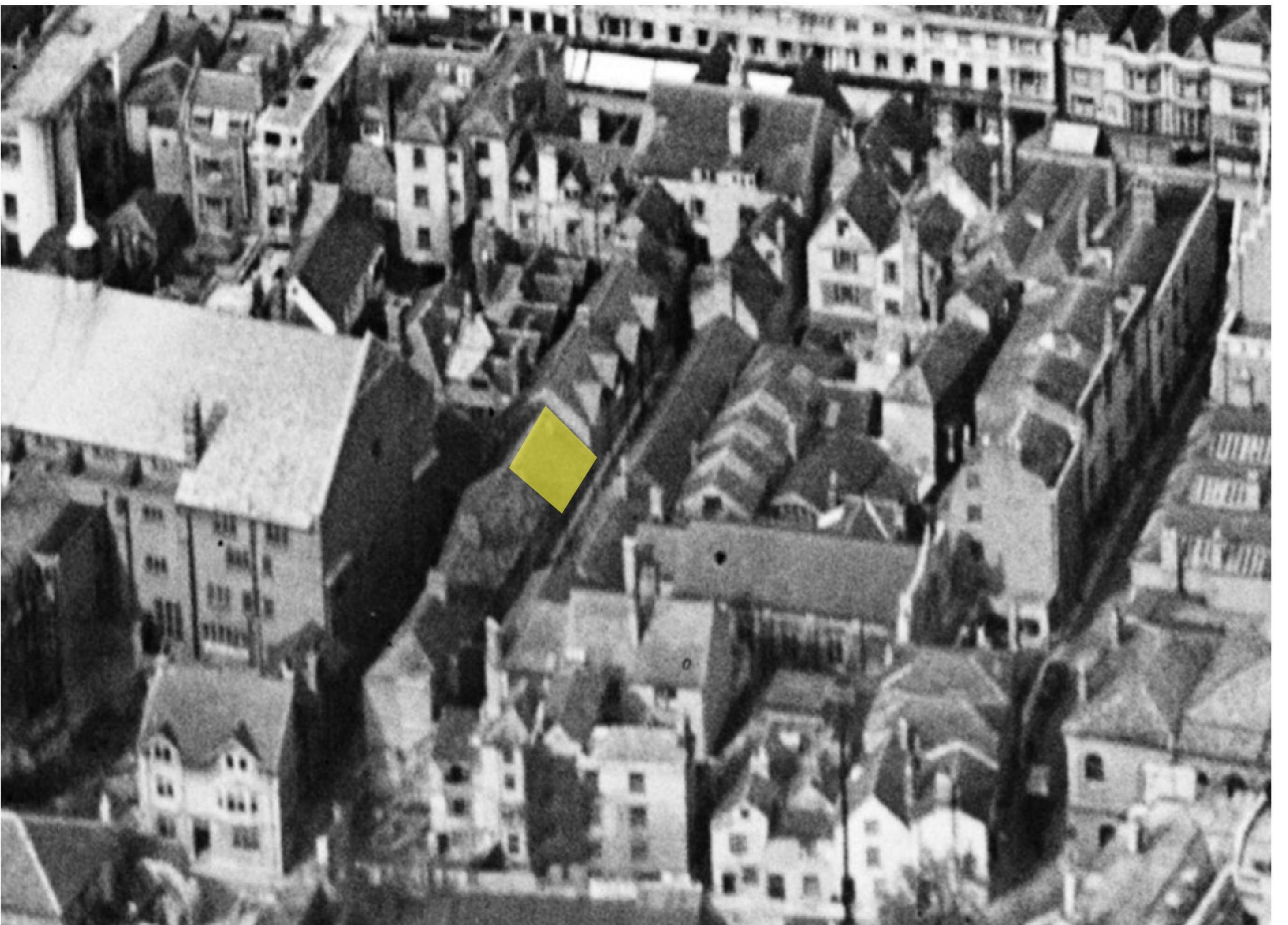
1937 aerial image showing the roof of the Wheatsheaf from the south-east and adjoining roofscape. The yellow dot is the area of roof proposed to be raised.
