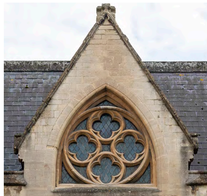
Clerestory windows in first floor of the library
