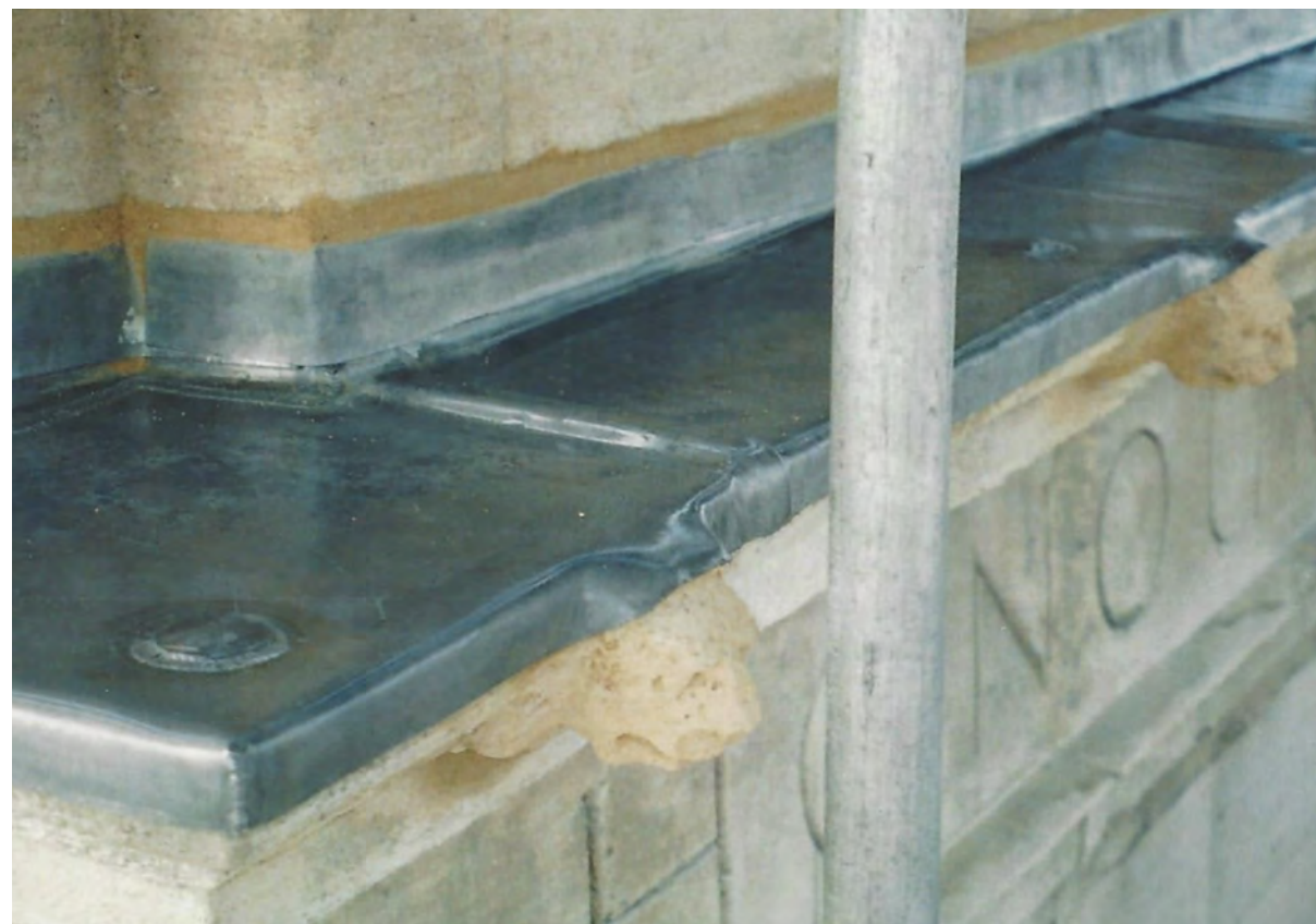
Example Lead / Stone Interface Detail
