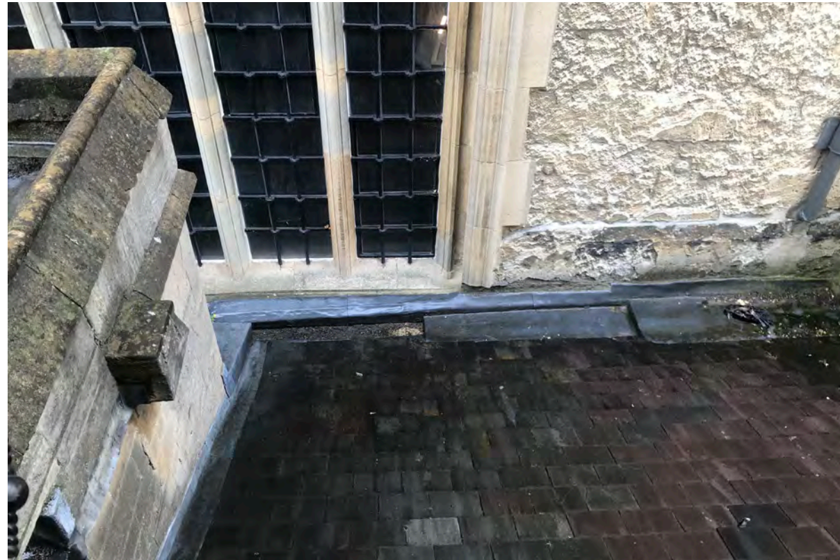
Existing condition showing leadwork abutting bodleian cill
