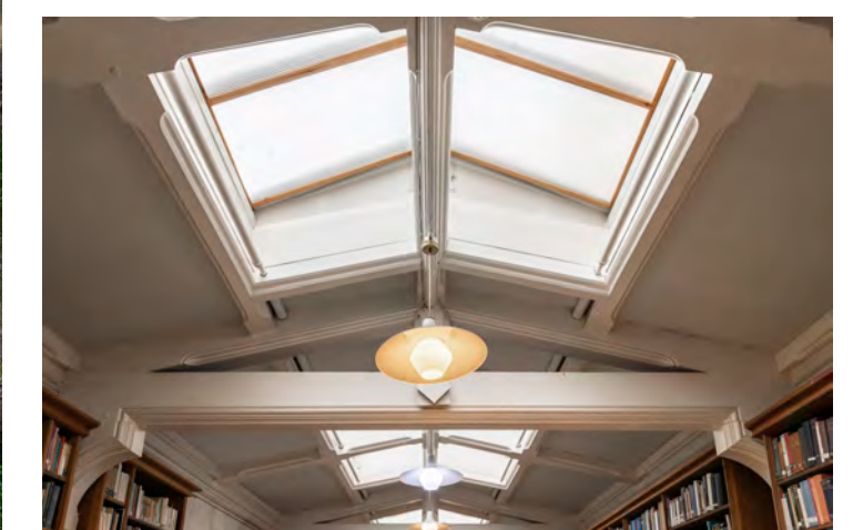
Interior photographs showing the roof-lights.
