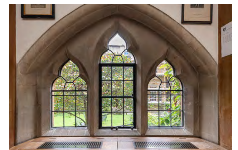
Existing Annexe West Windows, Obscured by Mezzanine
