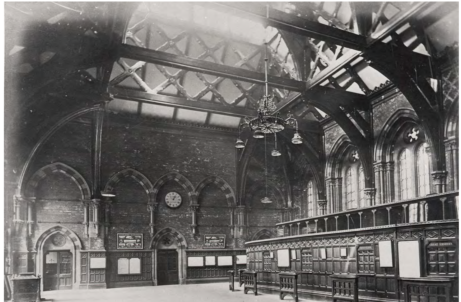
Clerestory windows at St Pancras ticket hall by George Gilbert Scott
