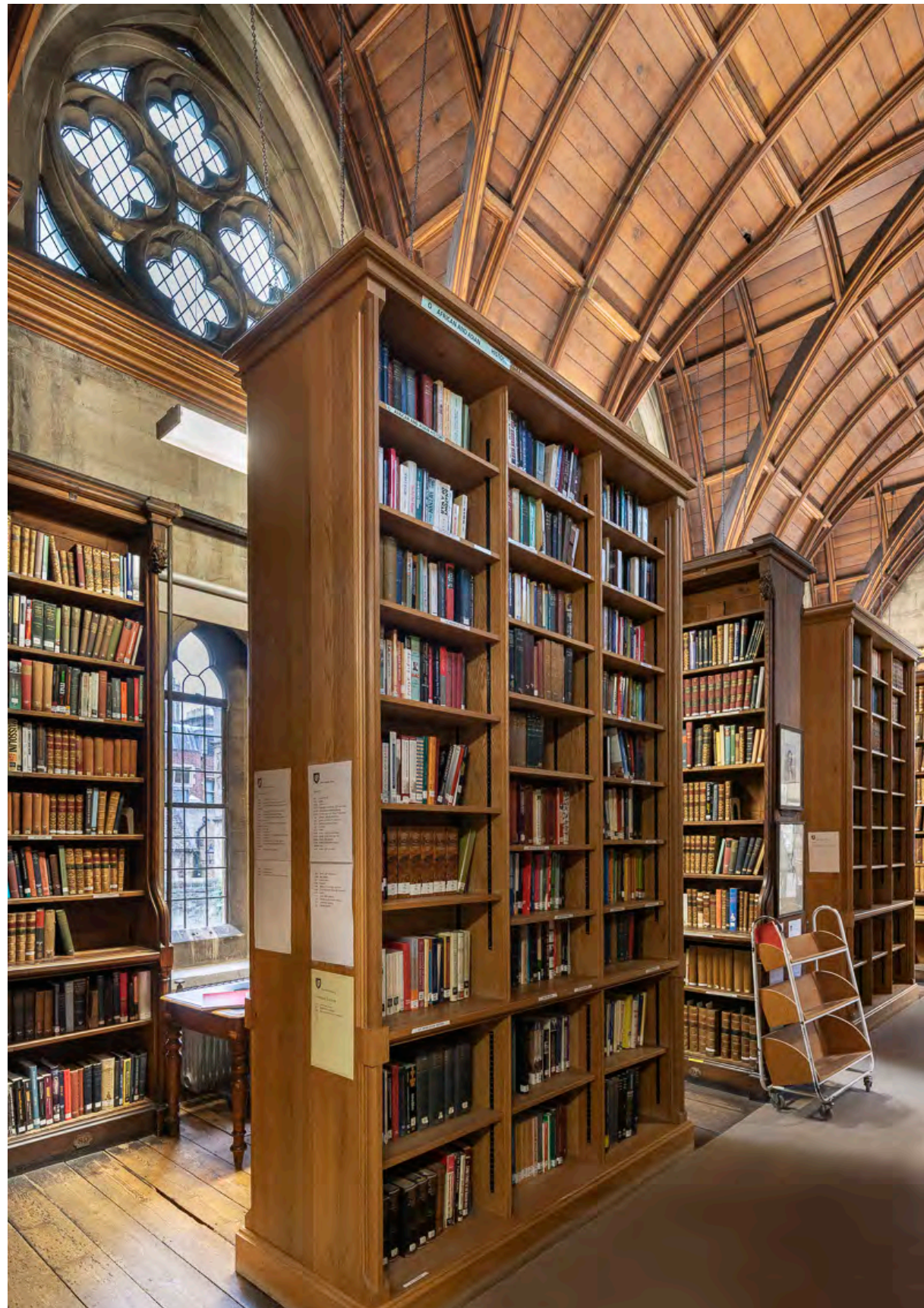
Clerestory windows in first floor of the library
