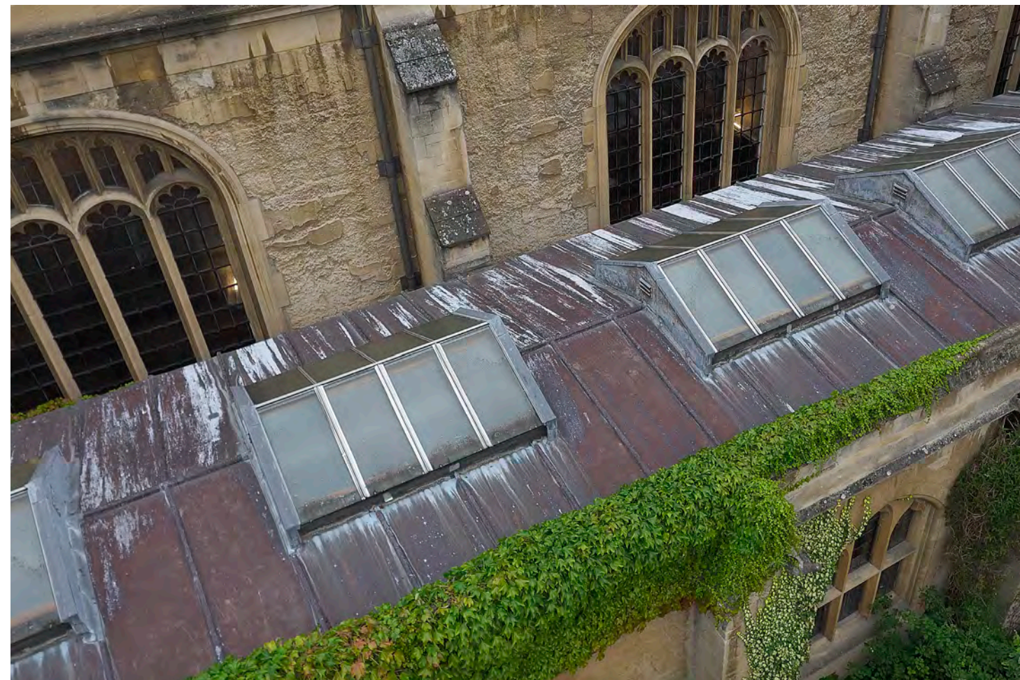
Aerial view of existing roof-lights installed in 1957
