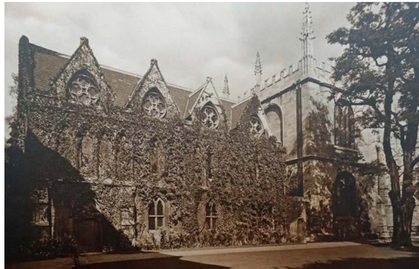
Plate 13. c.1930 photograph showing the front (south) elevation of the Library when it was covered in ivy (Exeter College Archive)
