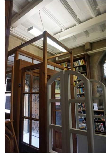
Plate 40 The modern and retracting glazed lobby around the west entrance to the Library, room G1, 2019 (Donald Insall Associates)
