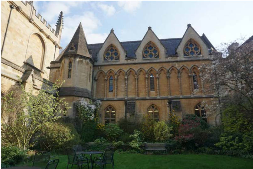
Plate 29 The rear (north) elevation of the main Library showing the corner turret and conical stone roof, 2019 (Donald Insall Associates)
