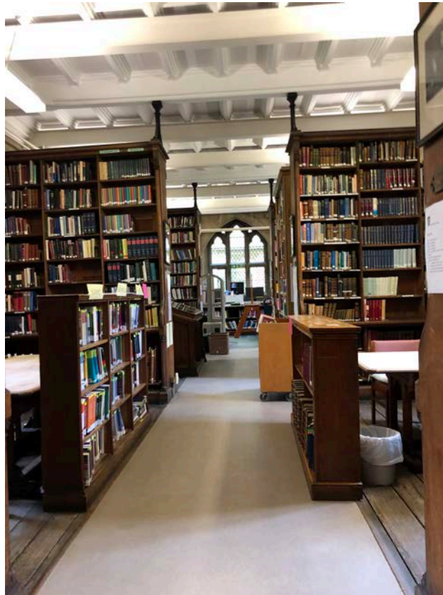
Plate 35 The ground floor of the main Library in room G1. This photograph shows the modern lino, 1898 steel girders, the original bookshelves and the original beamed ceiling, 2019 (Donald Insall Associates)
