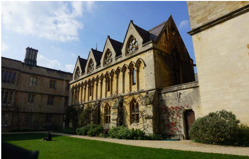
Plate 28 The side (east) elevation of the main Library including the original low stone wall between the Library and the Bodleian, 2019 (Donald Insall Associates)
