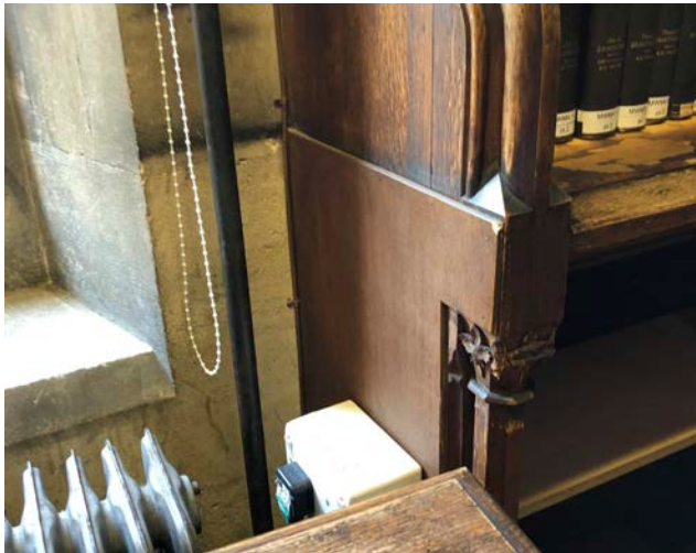
Plate 54 Detail of the modern plywood fixed to the side of the bookcases, room F1, 2019 (Donald Insall Associates)
