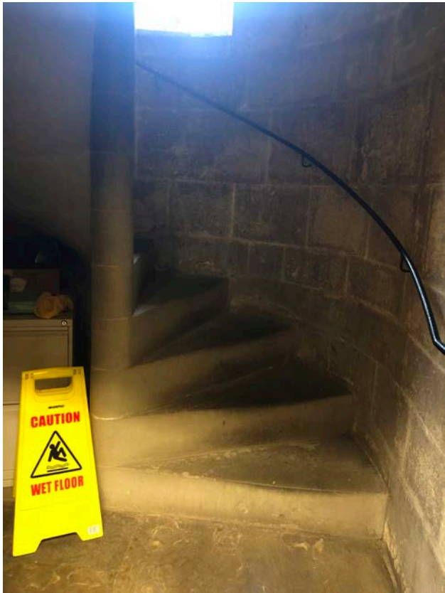
Plate 34 The original spiral-stone staircase in ST1, 2019 (Donald Insall Associates)
