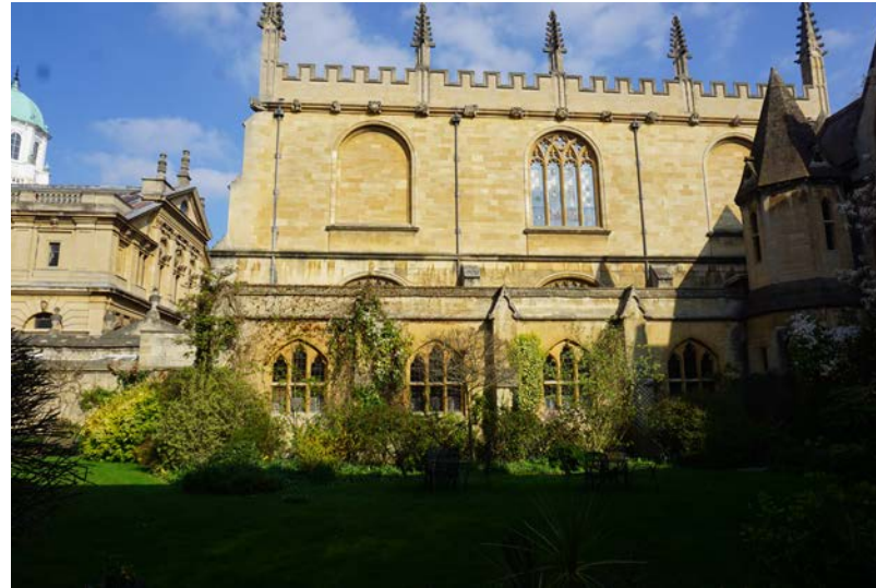
Plate 30 The front (west) elevation of the Annex, 2019 (Donald Insall Associates)
