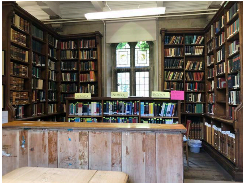
Plate 41 The modern lights, roller blinds and heating pipes running above the bookshelves, room G1, 2019 (Donald Insall Associates)
