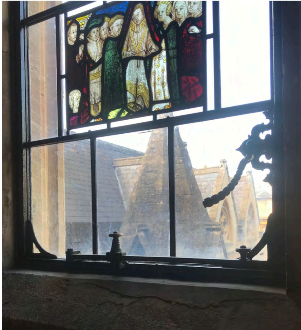
01. First Floor Central Window - Existing
