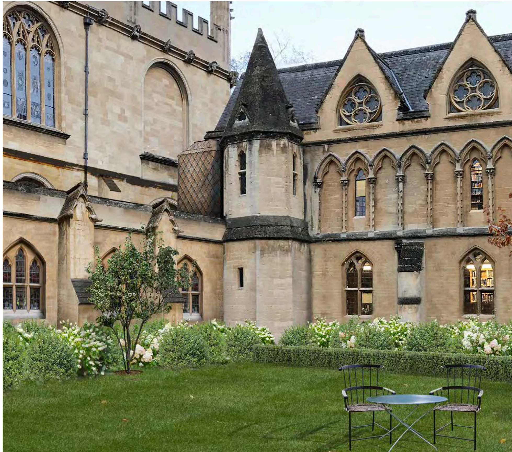
View of lift overrun from Rector's Garden
