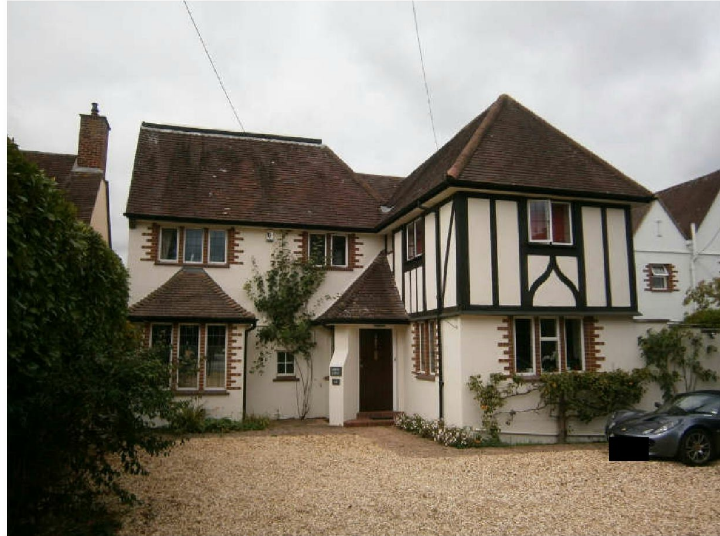
Image 3: Existing front (east) entrance
