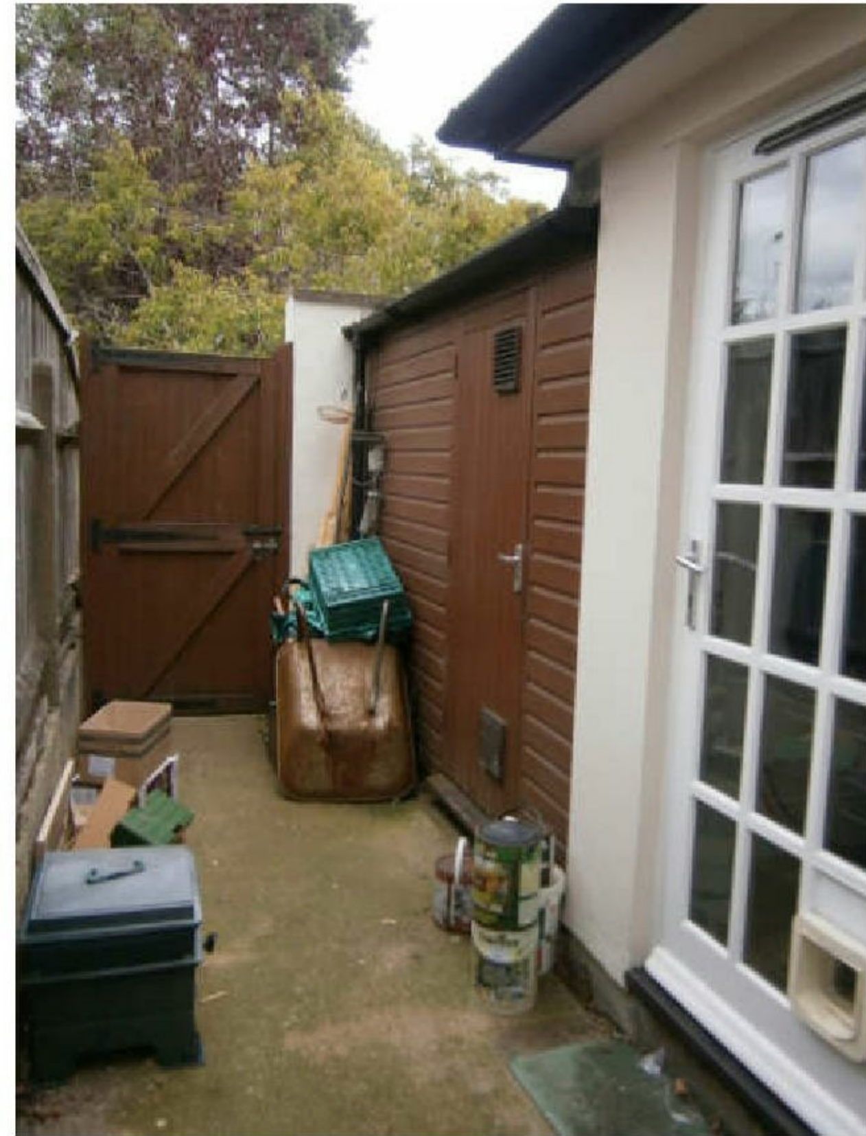
Image 7: View of existing single storey side extension and store behind frontage wall
