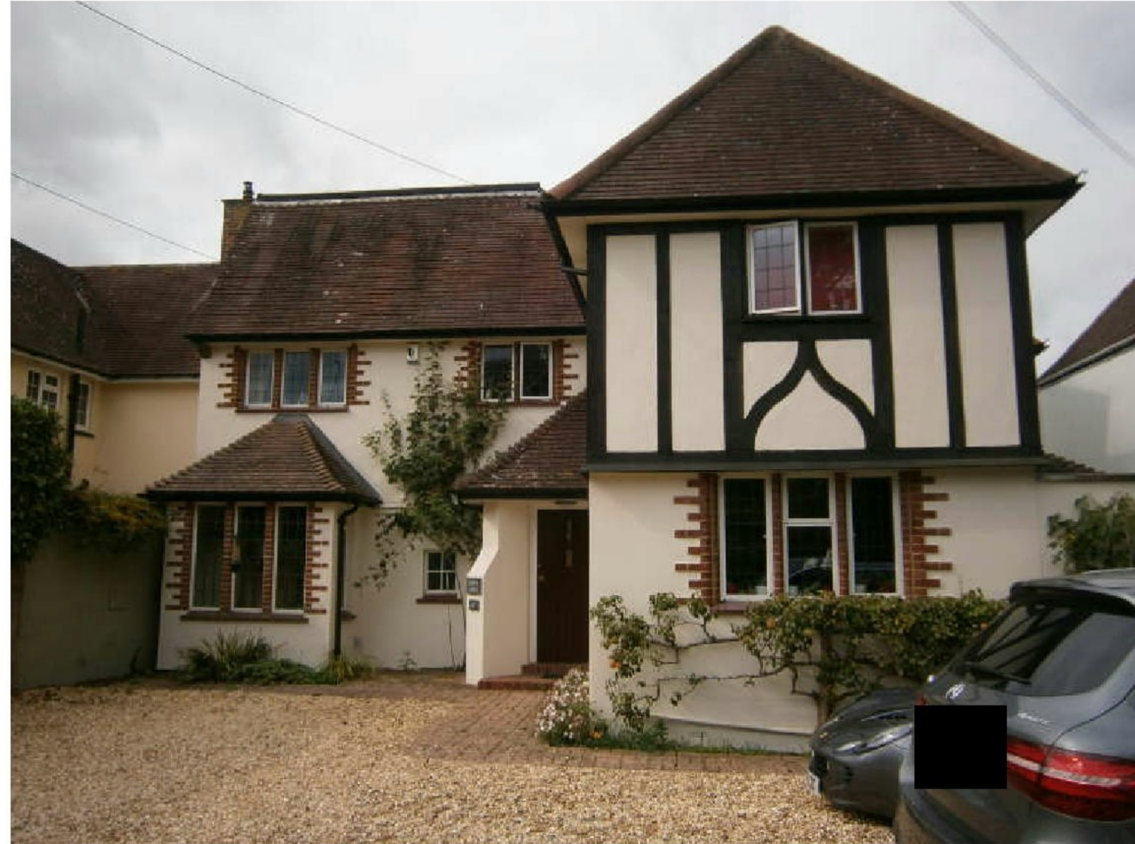
Image 5: Close-up of existing front (east) elevation
