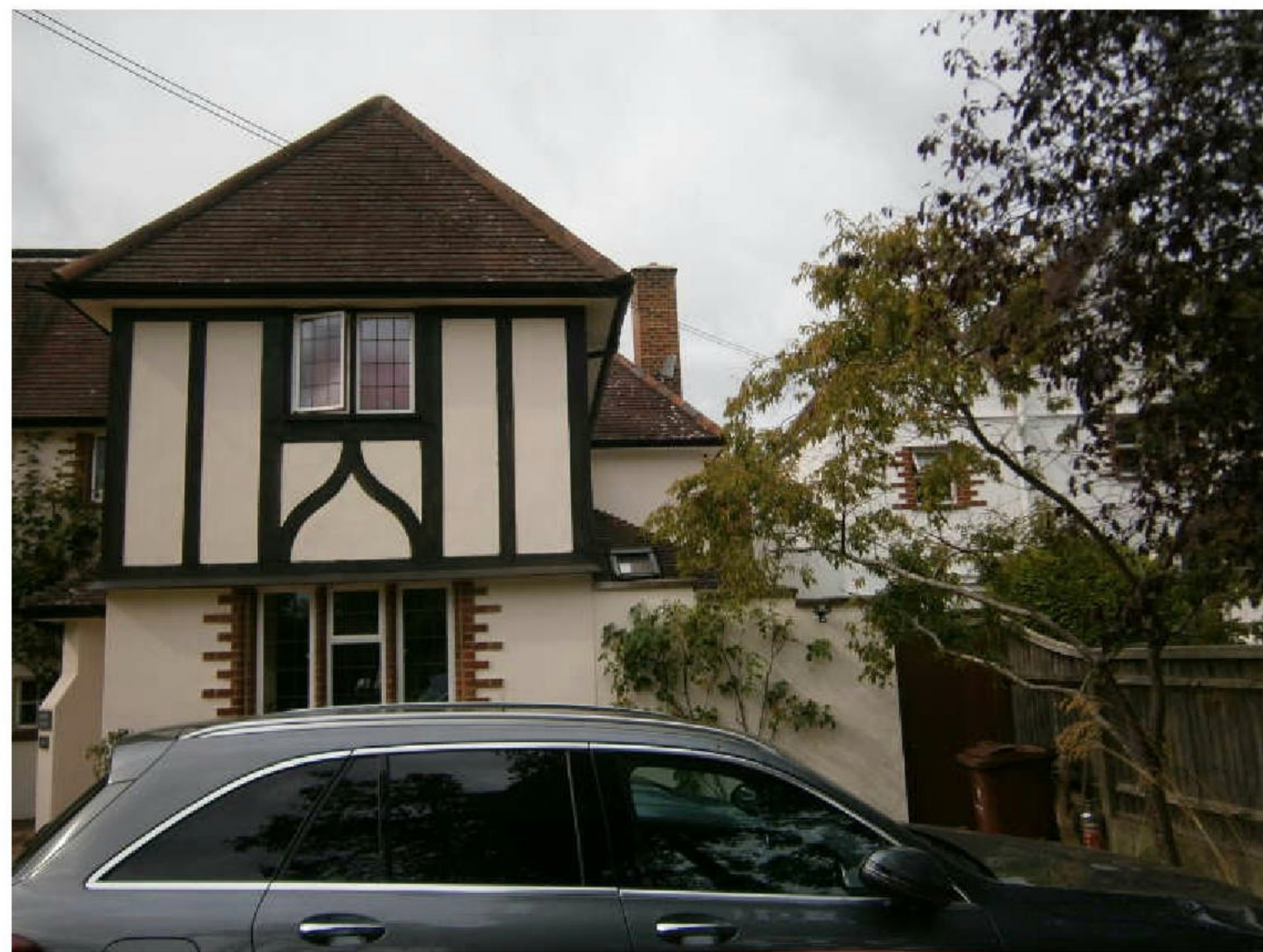
Image 6: Close-up of proposed location for part two storey and part first floor side extension
