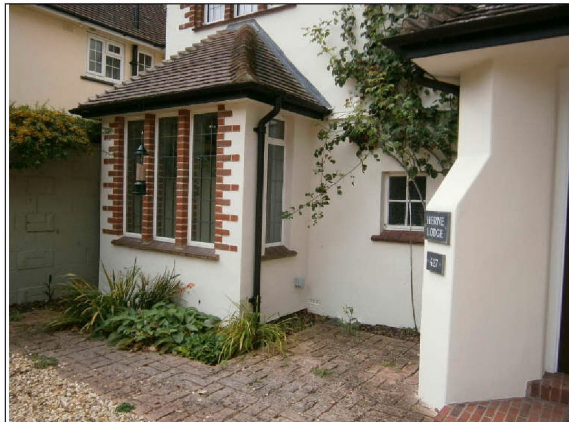
Image 8: Close-up of existing bay window
