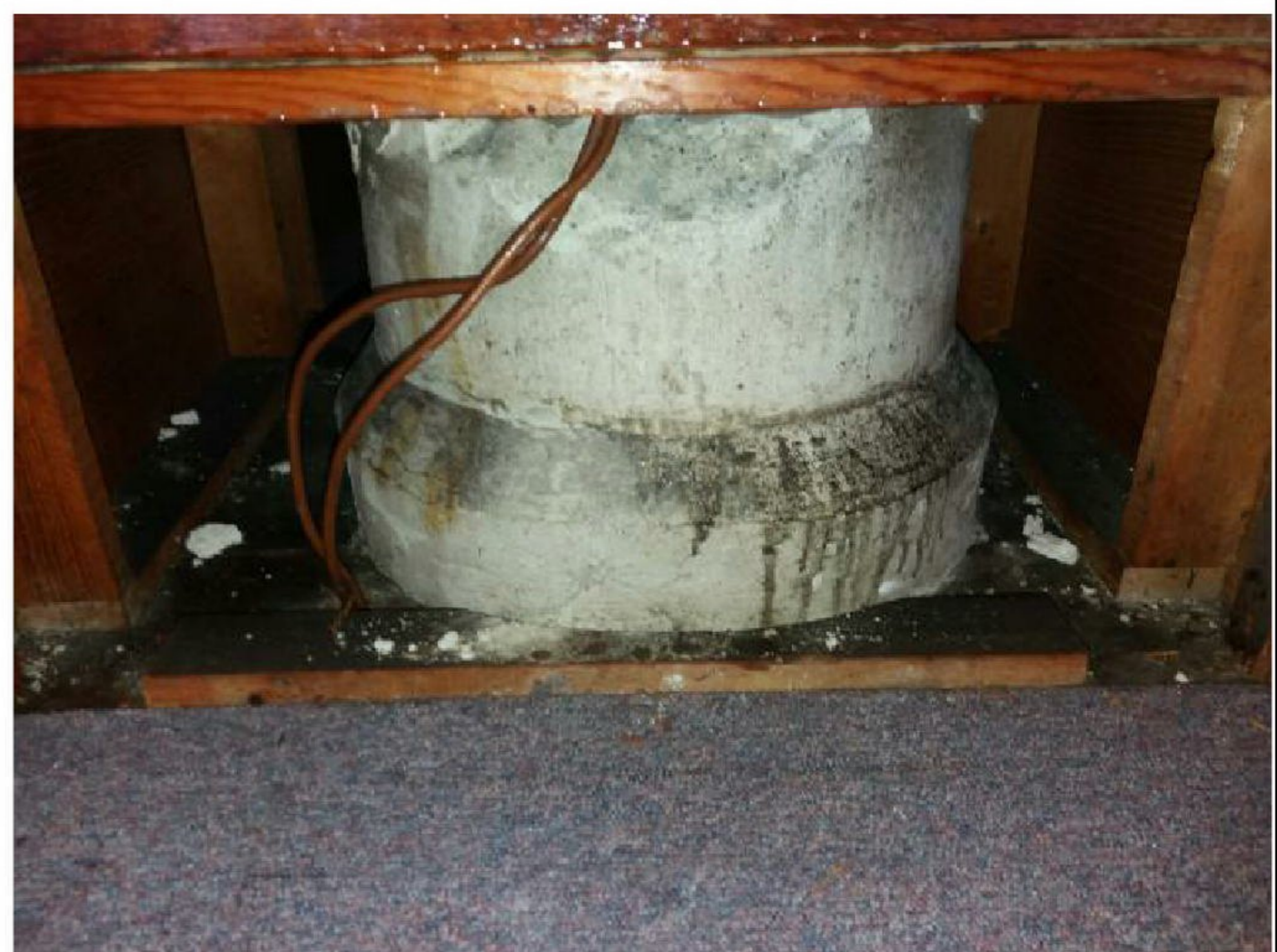
Base of column via removed access panelling
