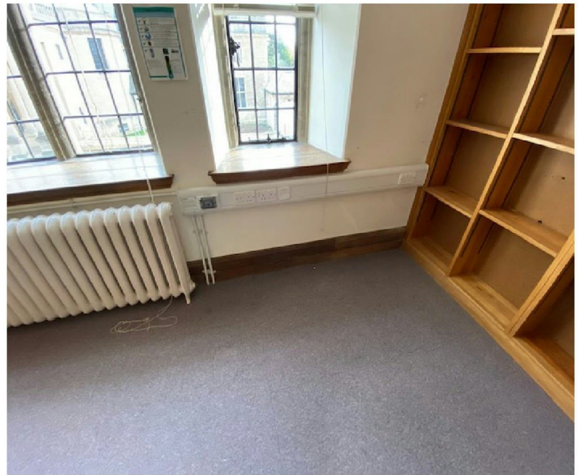
Area 1 window detail
