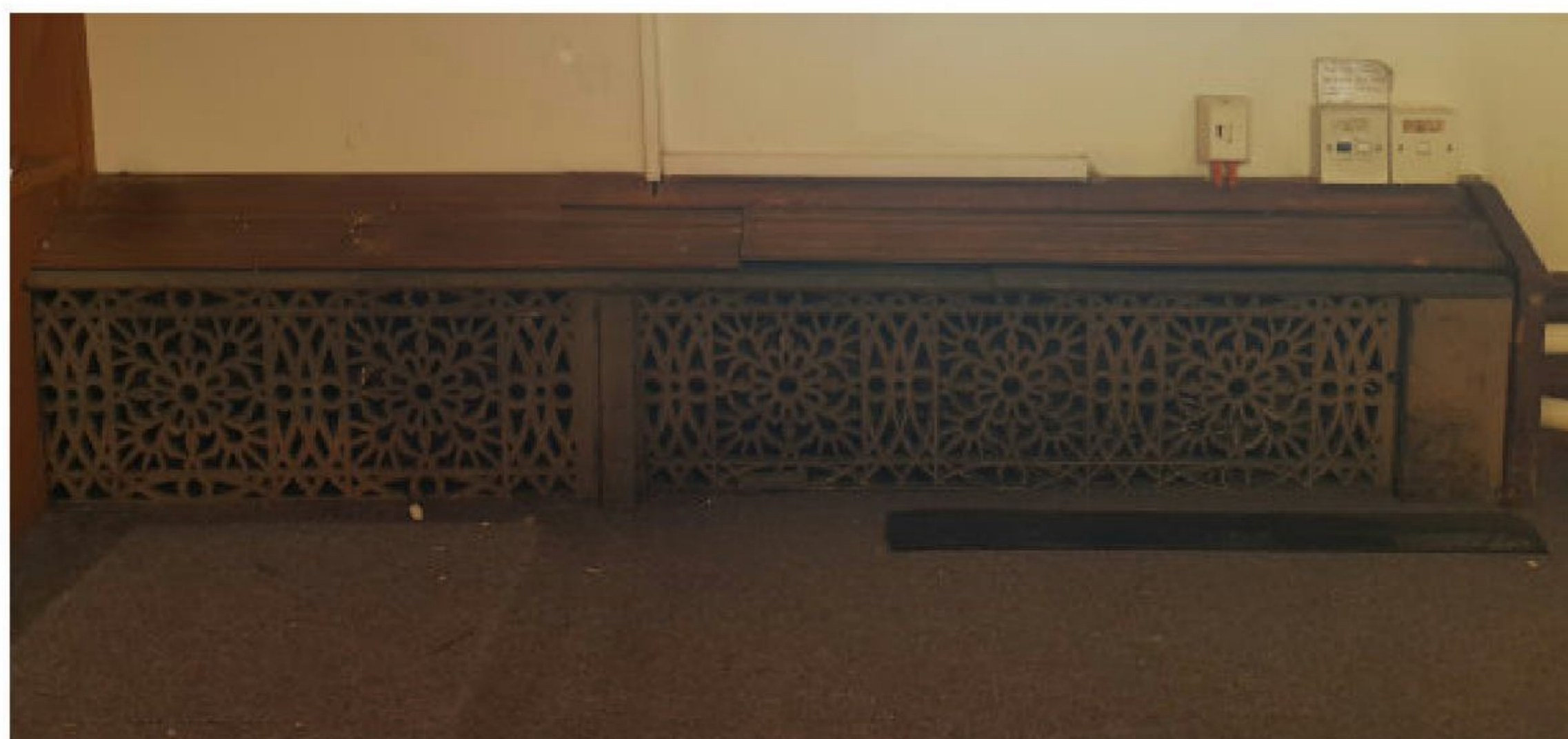
View 9 - decorative metal grille and adjacent joinery at skirting level
