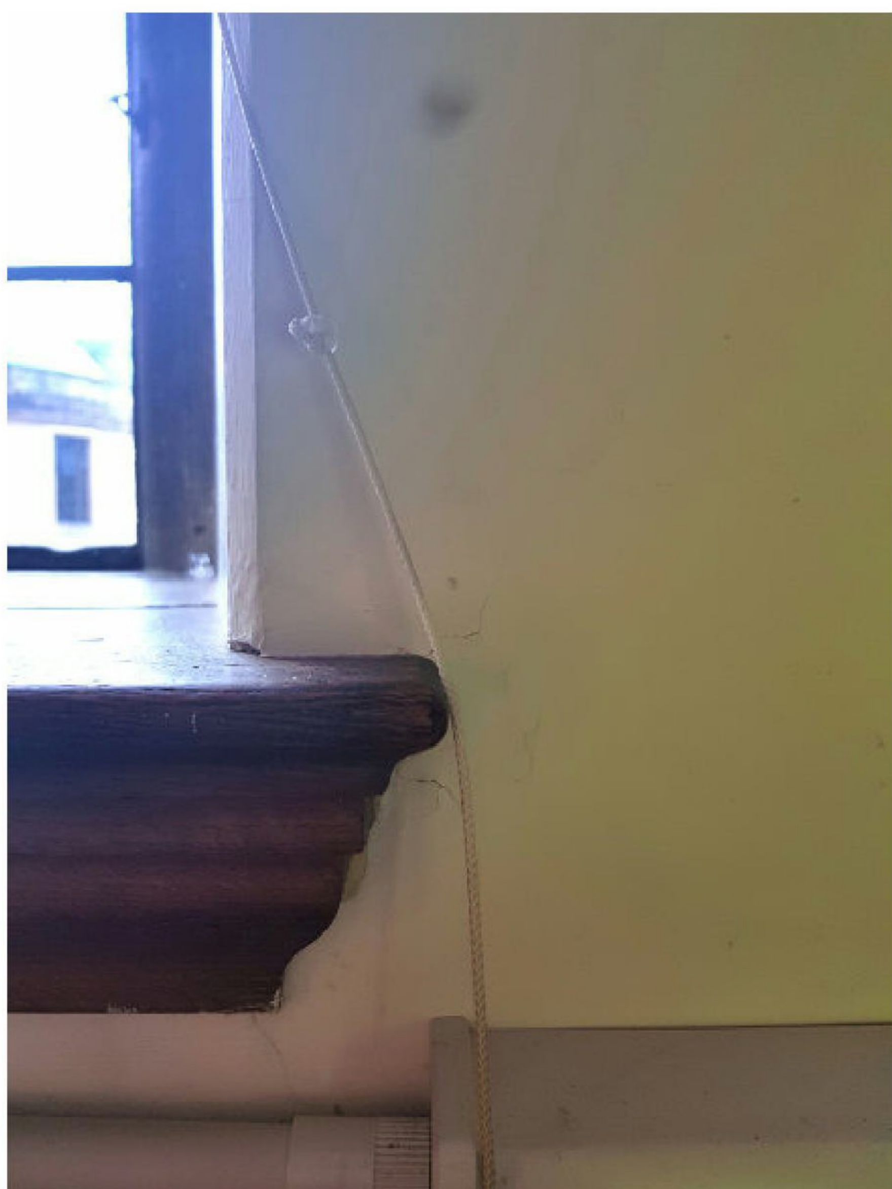
View 11 - window sill, profile
