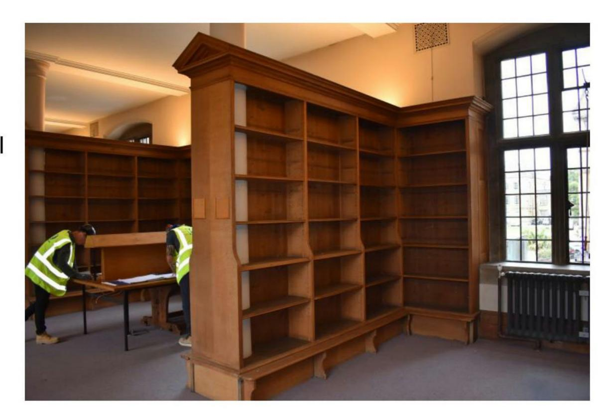
The bookcases are generally in good condition although areas of damage are visible where modifications have been made to the bookcases over time. Investigations have been undertaken on site to understand the construction of the bookcase and how they could be dismantled to enable modification as required for the proposed scheme.
