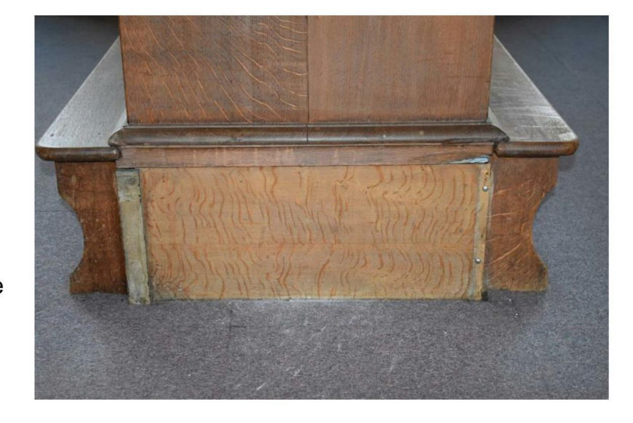
With the panel removed you have access to the void space under the bookcase. Note plaster column penetrates through the base of the bookcase and floor. Plaster casing which contains ACM's has been damaged to allow installation of lighting to the top of each bookcase.
