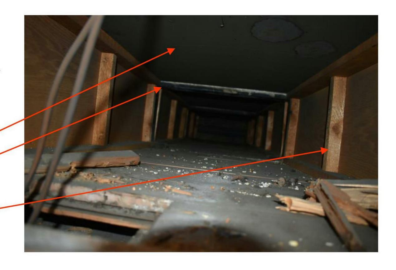
Foot of ironwork support strap – these are screw fixed to the floor boards.
