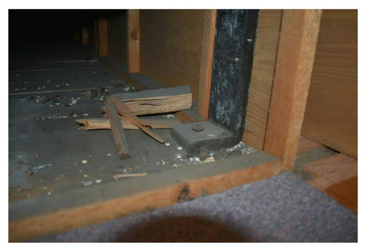
Plinth step is pinned to the plinth panel and can be removed by easing away from the bookcase as a single item. Each of the support legs is also pinned to the step itself. With the step removed it is possible to remove the remainder of the plinth panels which are pinned to the support framework. (Note these panels are faced plywood 4mm thick and require care to remove without damage.).
