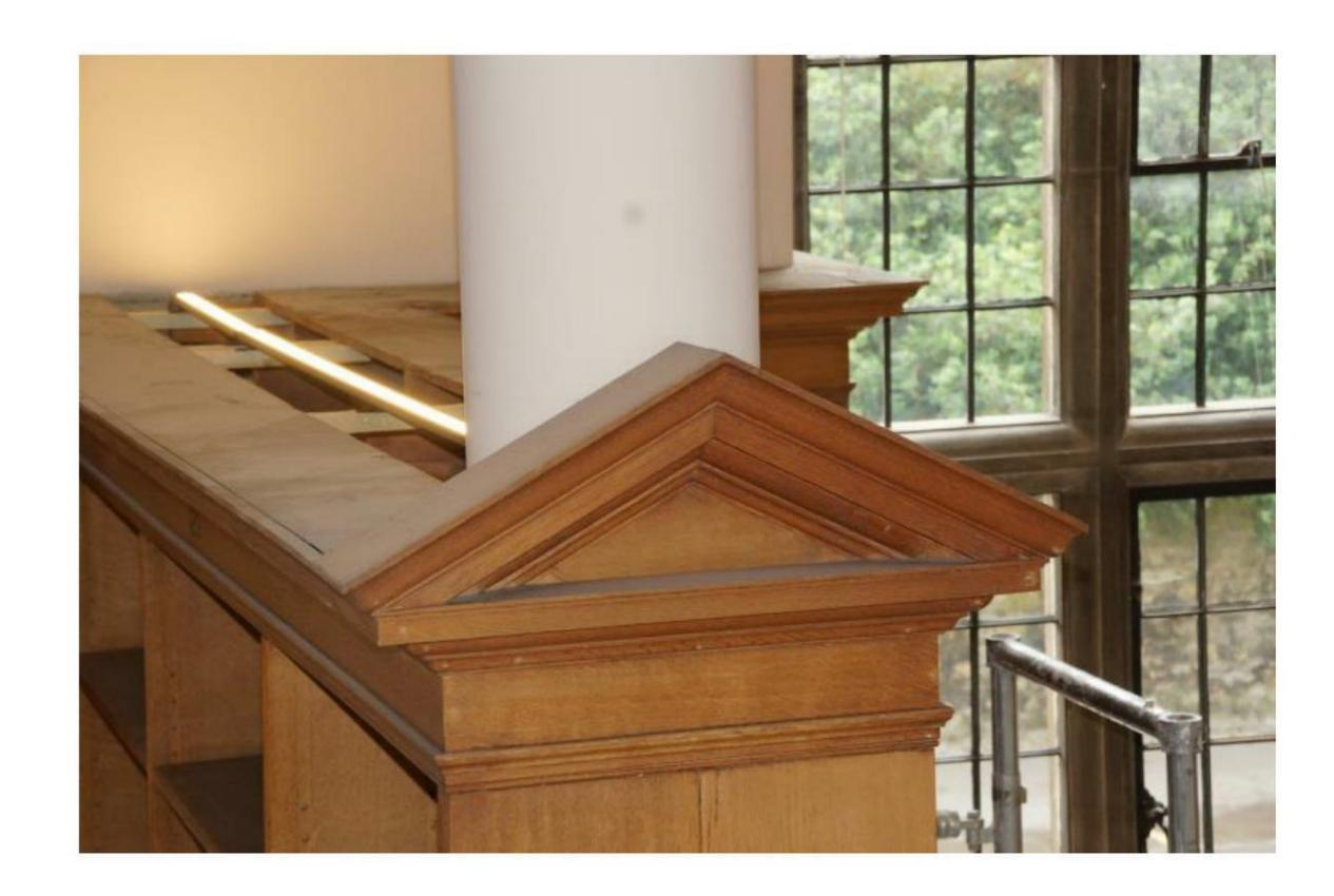
With the covers removed it is possible to the wooden coving to the pediment end and sides of the bookcase. The bottom edge of these slot into a groove in the bookcase top moulding piece. It is both nailed and glued in place.
