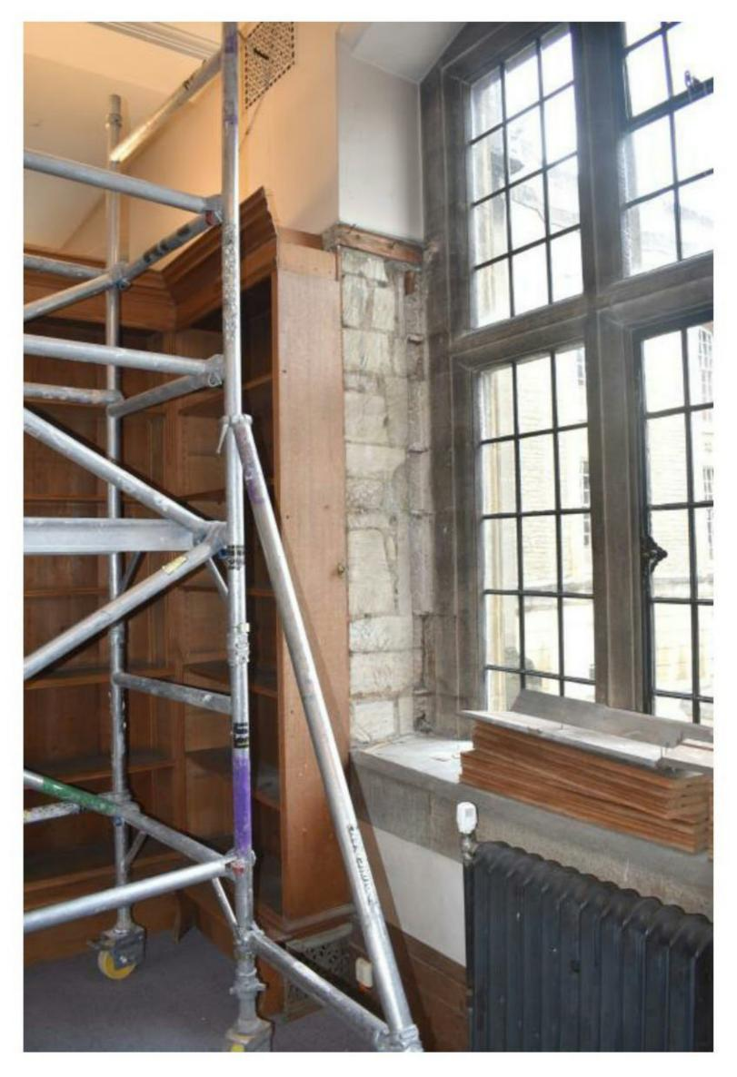
Coving removed from window to external corner of bookcase (pinned and glued at mitre) which allows release of the reveal panel from the grounds and rotated from the bookcase rebate.
