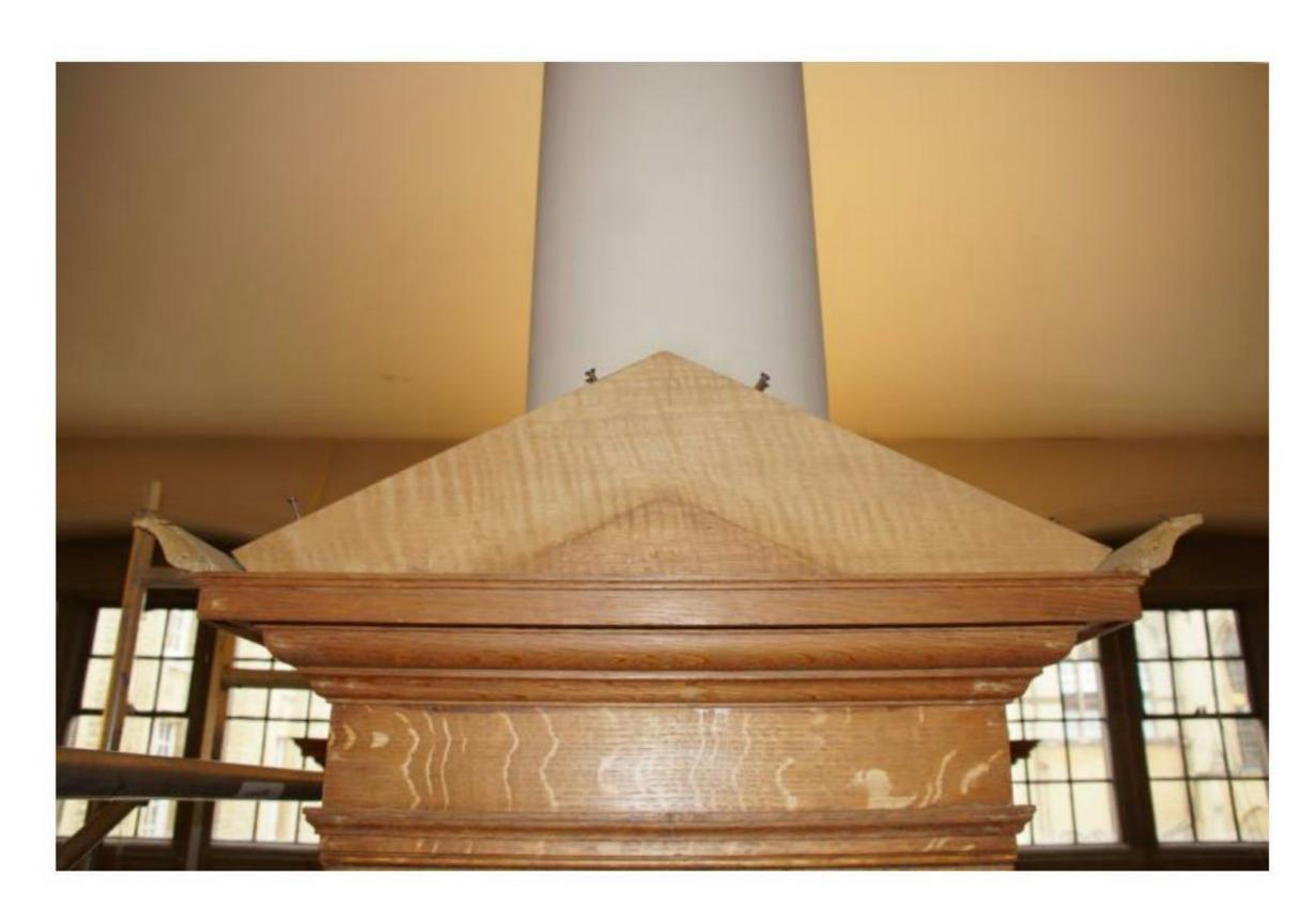
Once the coving has been removed the top moulding can be removed. This is secured by nails into the bookcase end and partition edges.
