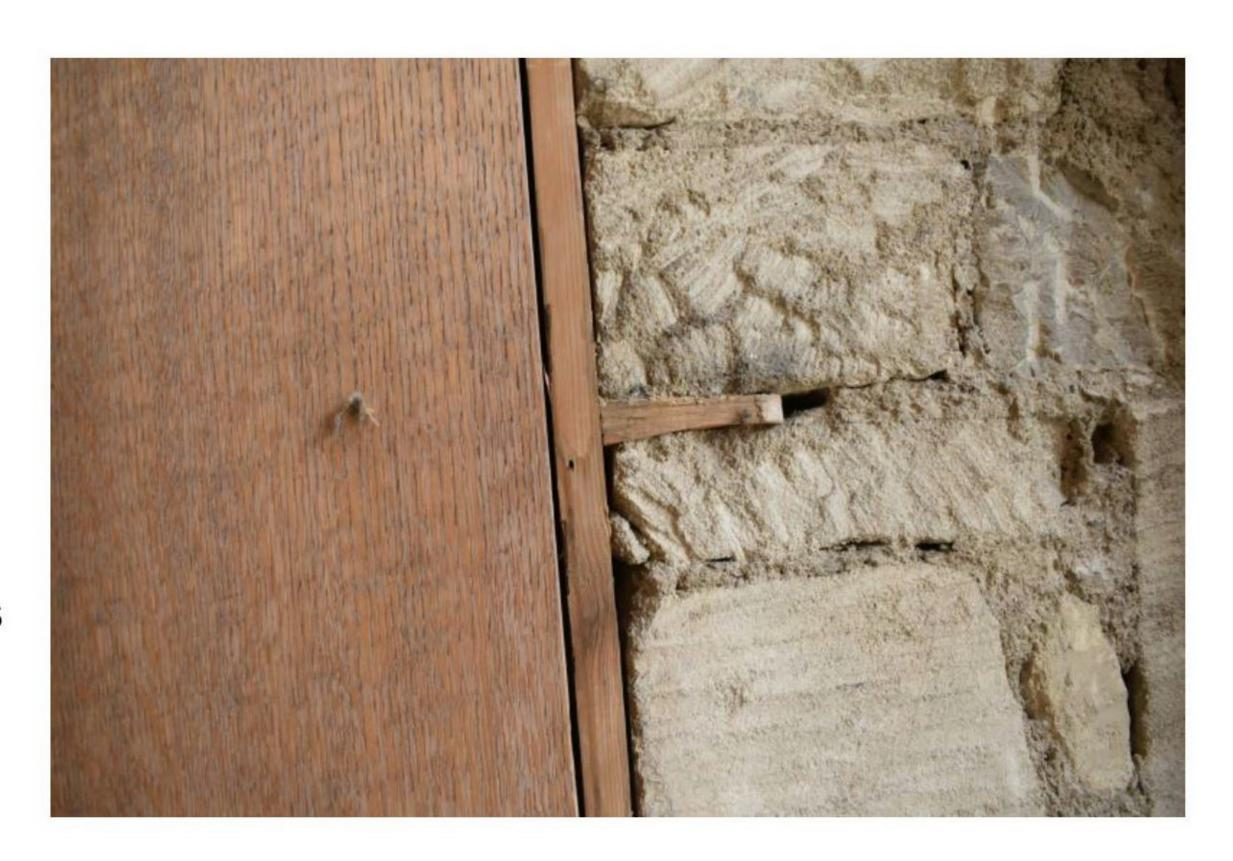
The wall mounted bookcases have been fixed in position prior to the projecting element which has a rebated joint into the end casing upright.
