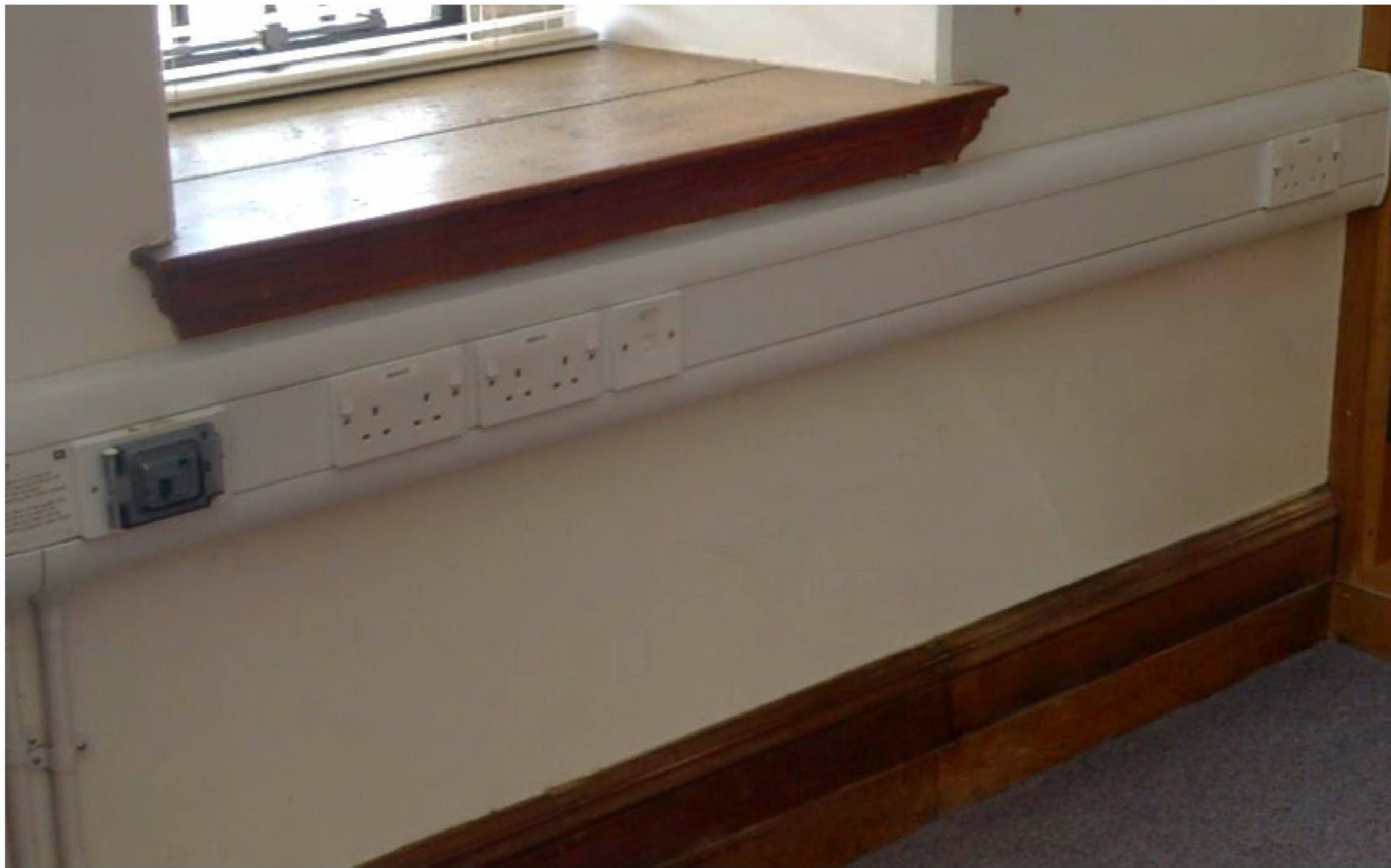
Timber windowsills, chamfered detailing to reveal and skirting
