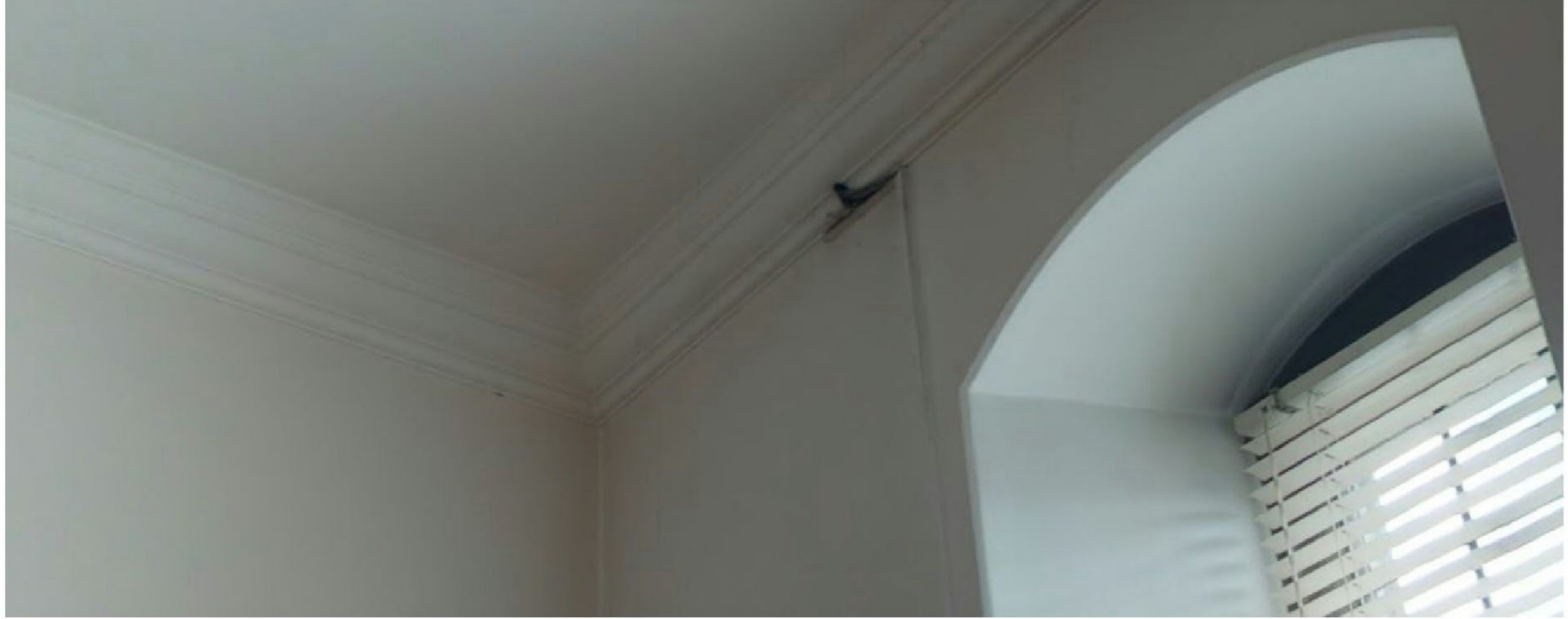
Moulded cornice, shallow arch-headed window reveal and chamfered edge
