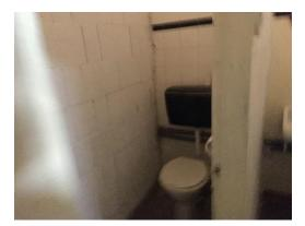
General view of existing WC block. Nonoriginal block wall and sanitaryware to be removed and existing utilities connections to be re-used.
