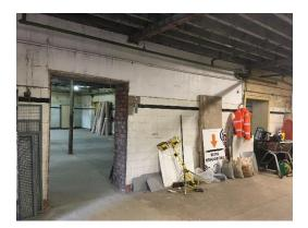
General view of dividing structural wall between building B and C. Proposal to enlarge both openings. Retain remaining ceramic tiles and protect with board lining.
