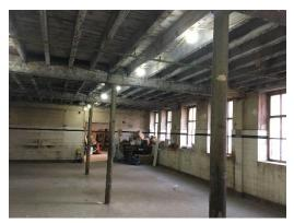
General reverse view of internal North elevation wall (drawing T09 Section A-B). Proposal to strip back non-original plaster above tiles to reveal original brick work. Clean and retain ceramic tiles. Original steel columns to be retained and decorated.
