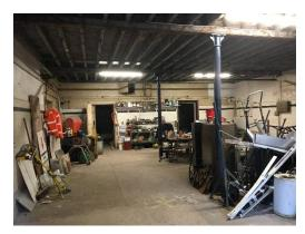
General internal view of the ground floor of application subject building C. Note level concrete floor slab to be retained and patch repaired as necessary.
