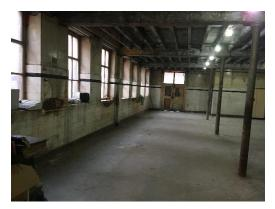
General view of internal North elevation wall (drawing T09 Section A-A). Proposal to strip back non-original plaster above tiles to reveal original brick work. Clean and retain ceramic tiles. Original steel columns to be retained and decorated. Original door (D2) to be retained and overhauled.
