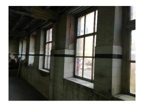
General close-up view of internal North elevation wall (drawing T09 Section A-A). Proposal to strip back non-original plaster above tiles to reveal original brick work. Windows to be retained and overhauled.
