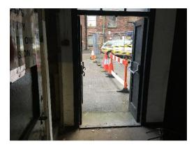
Internal view of Door D3 to be retained, overhauled and converted to an accessible personnel door
