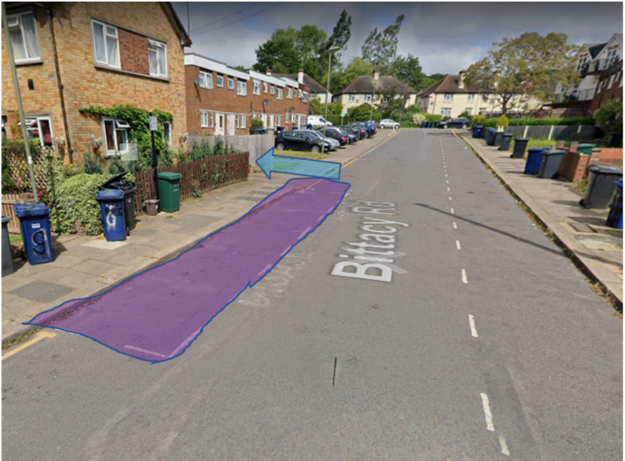
Indicative proposed area for parking suspensions & roadside compound to be installed. Blue arrow indicates start of day to day pedestrian walkway.
