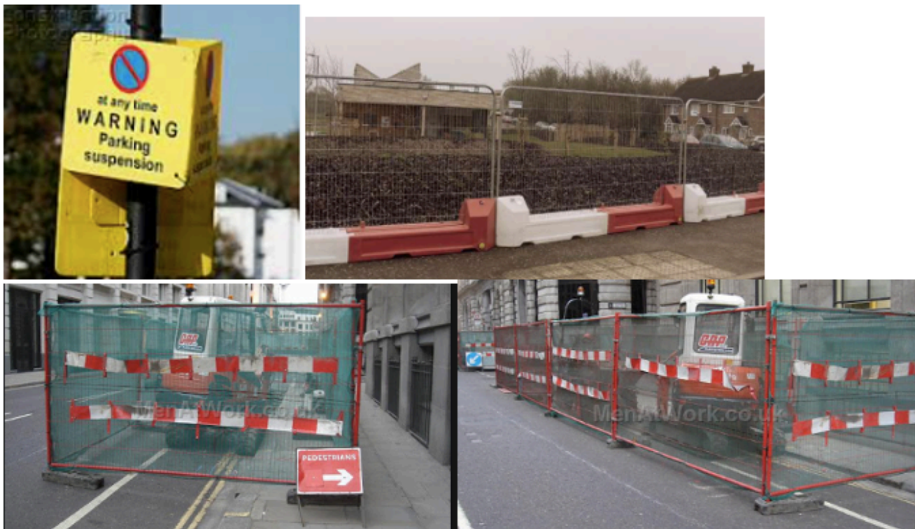
Indicative images of example roadside compound arrangements.
