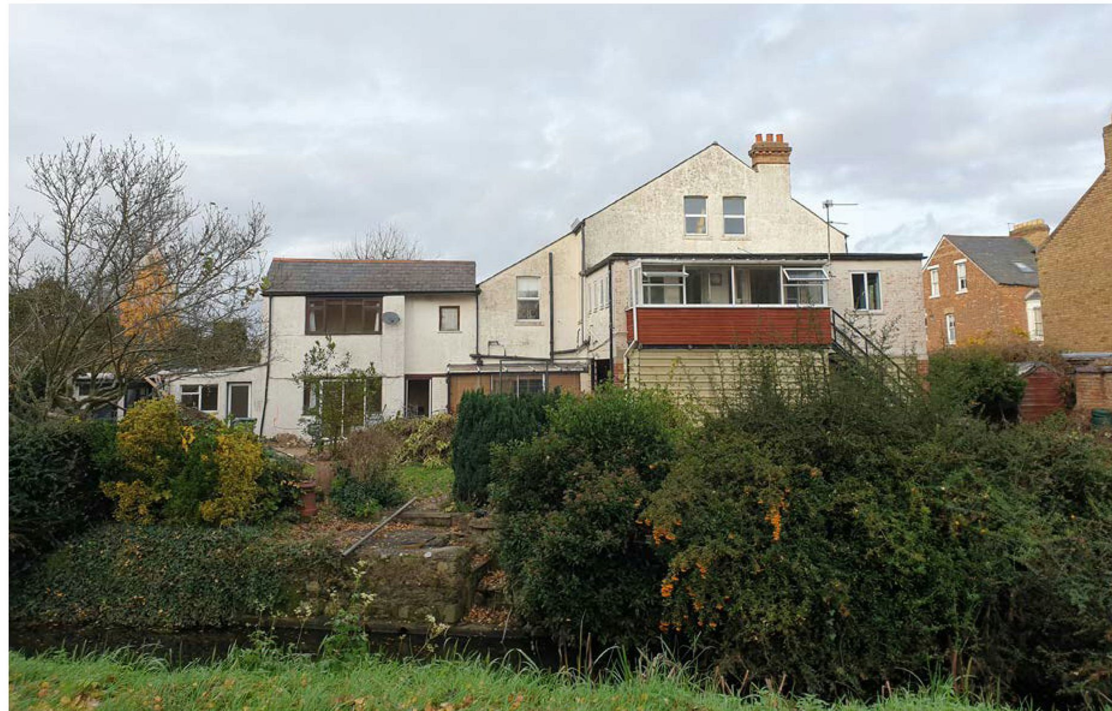
Above; North Elevation of 90 Chilswell Road from Hinksey Park
