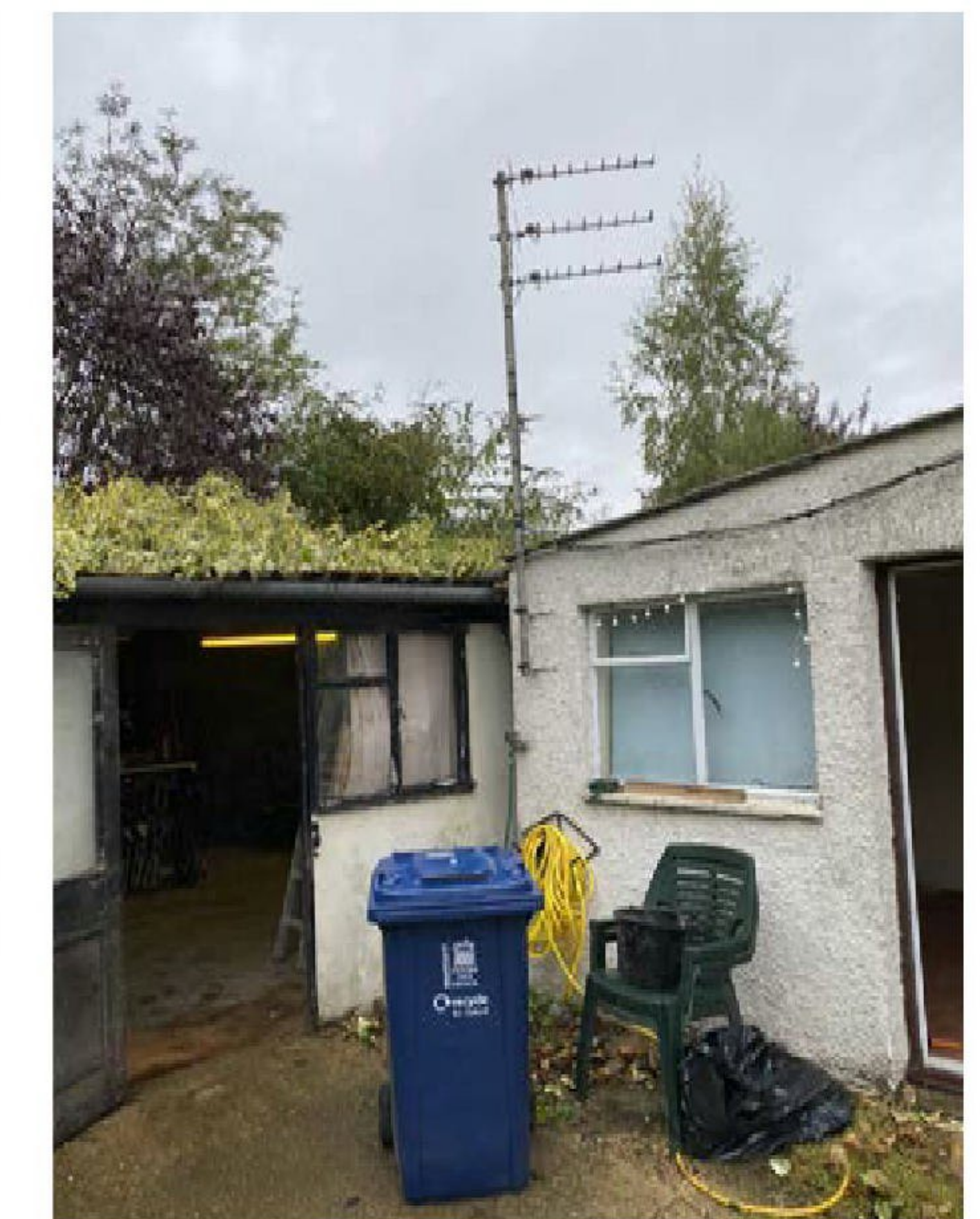
Above; Current location of bin storage at rear of property.
