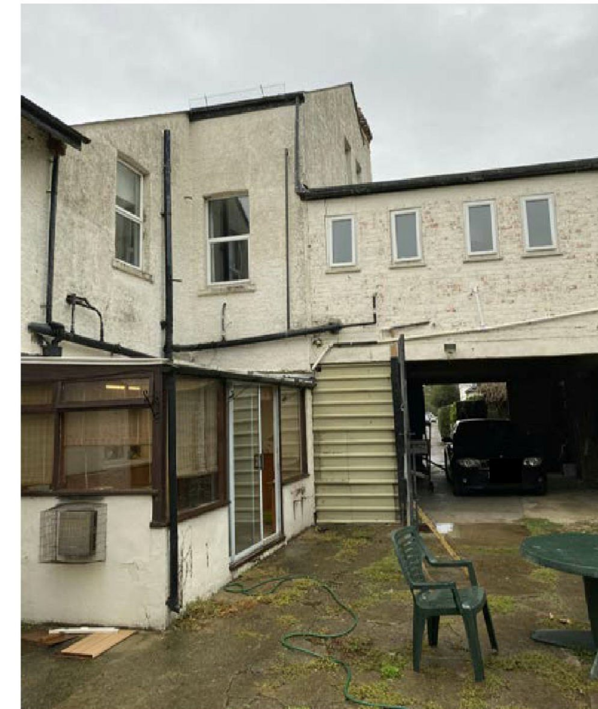
Above; Rear elevation showing previous extensions
