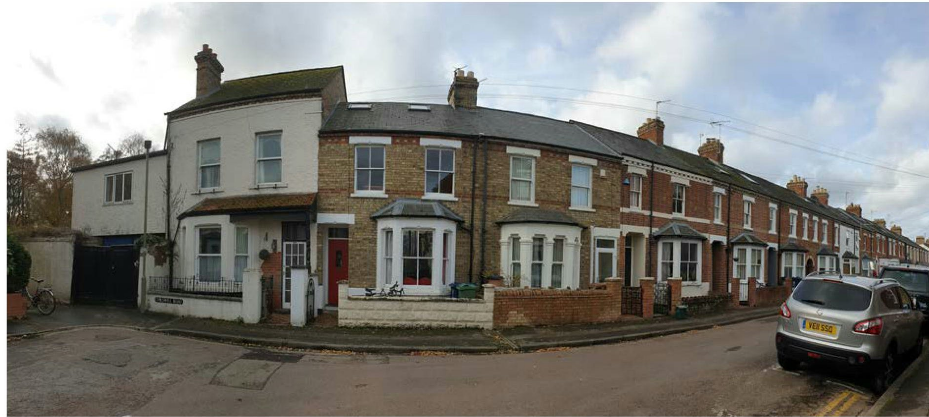
Above; Front elevation of 90 Chilswell Road within streetscape
