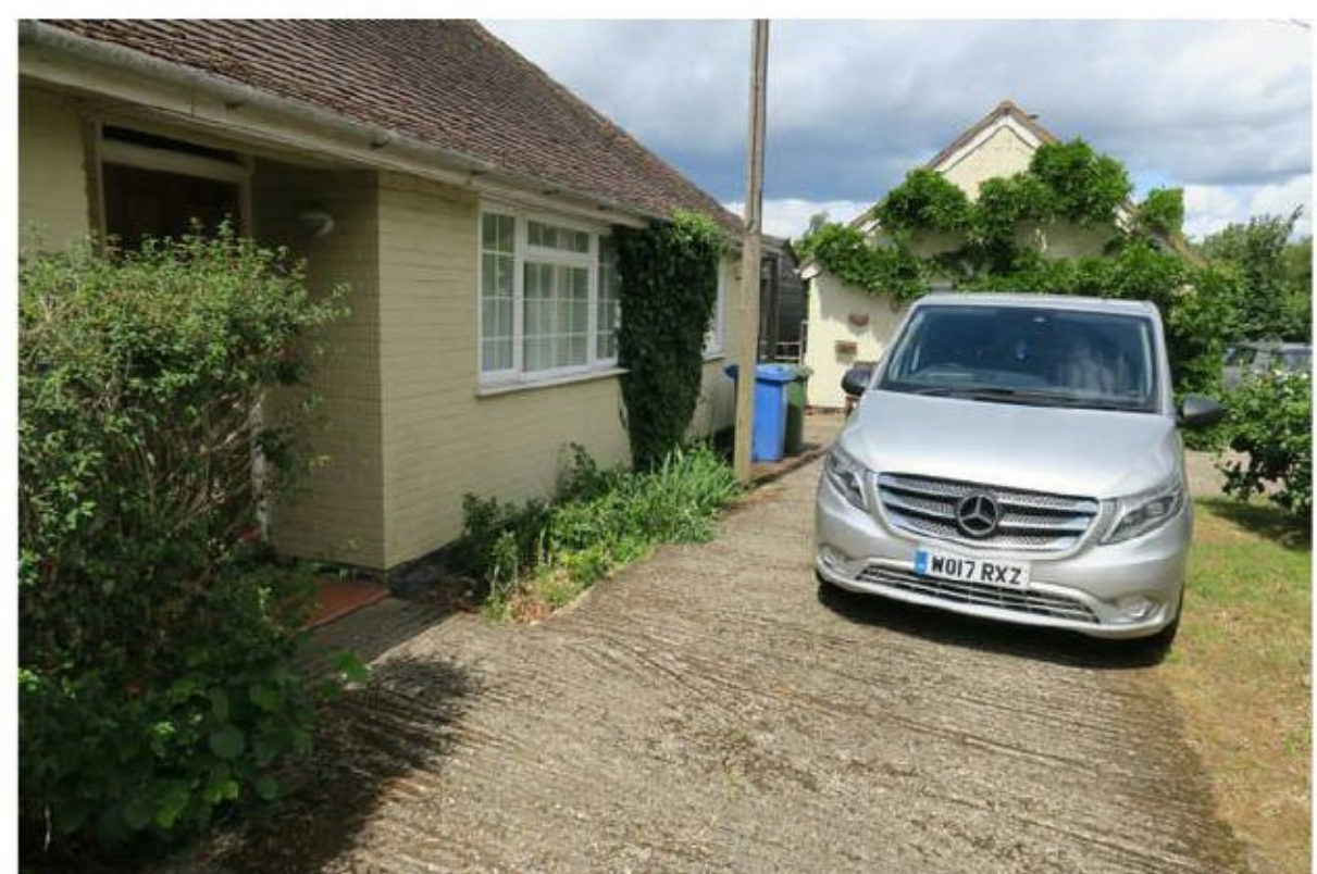
Photograph 18. Tarmac parking area to east of the Cottage.
