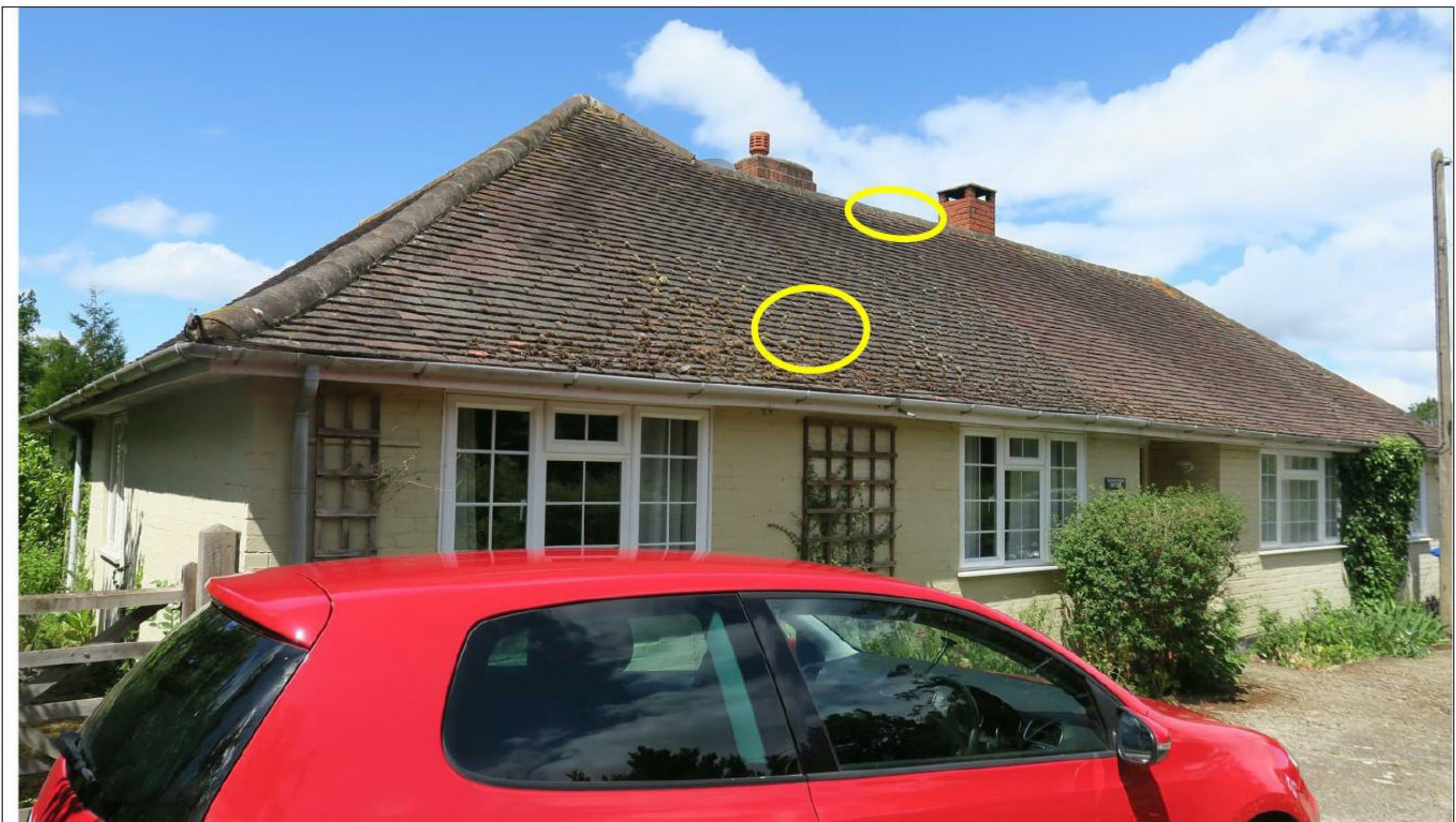
Figure 4. Yellow circles depict the approximate locations of common pipistrelle emergences from the Cottage's eastern roof pitch on the 30/06/20.
