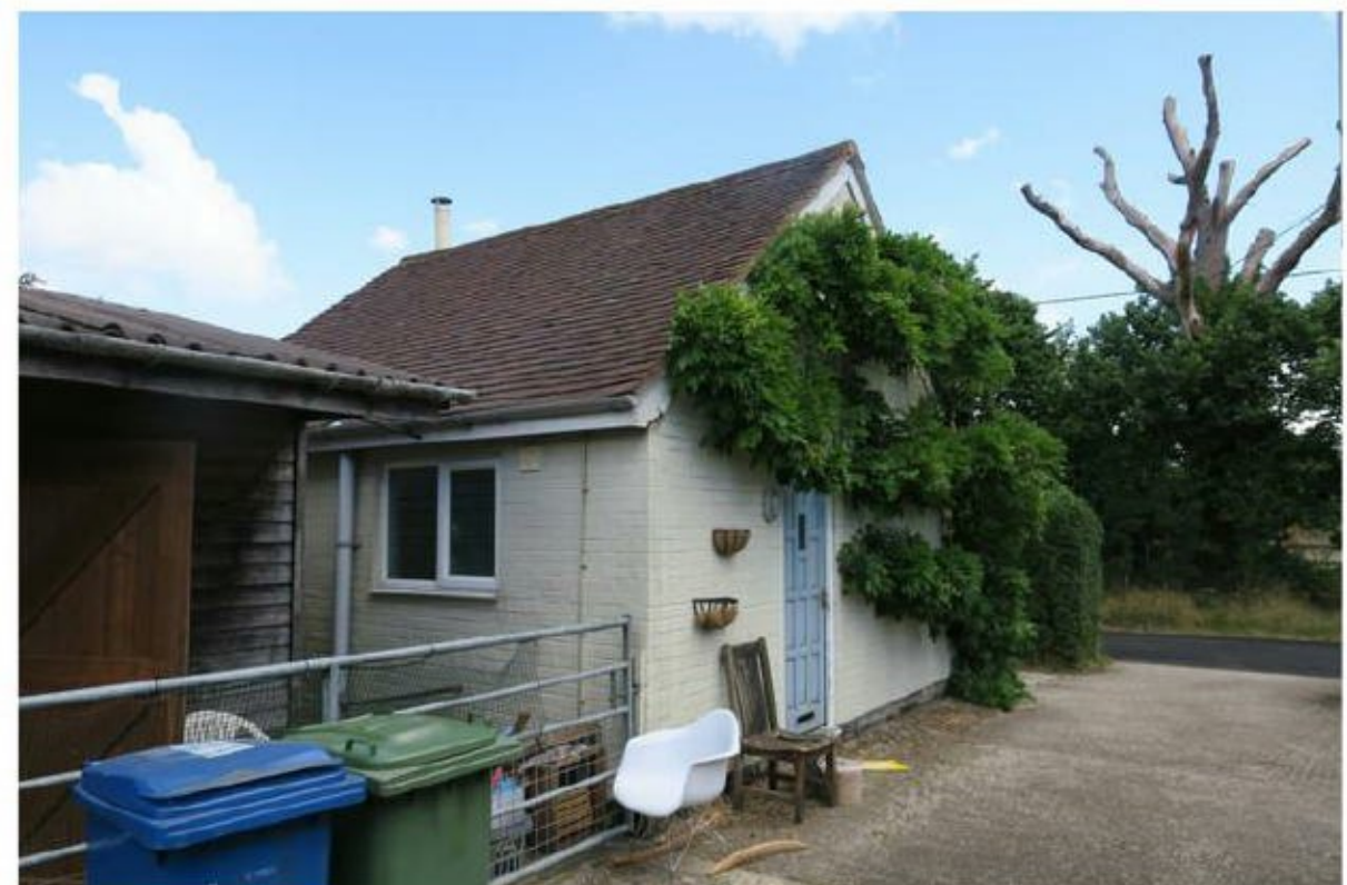
Photograph 6. The Annex viewed from the south-west.
