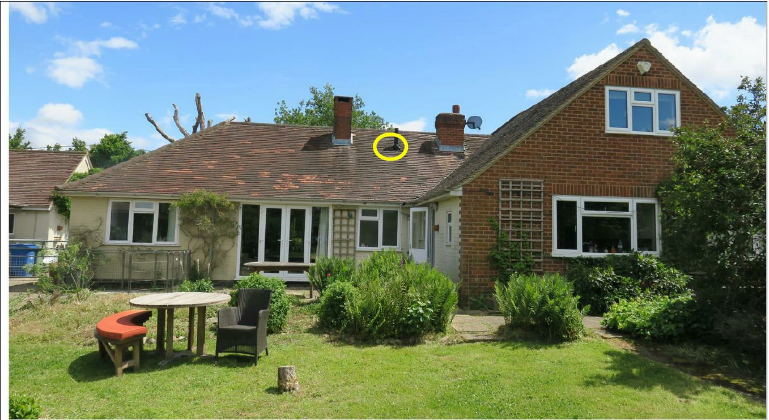
Figure 5. Yellow circle depicts the approximate location of common pipistrelle emergence from the Cottage's western roof pitch on the 30/06/20.
