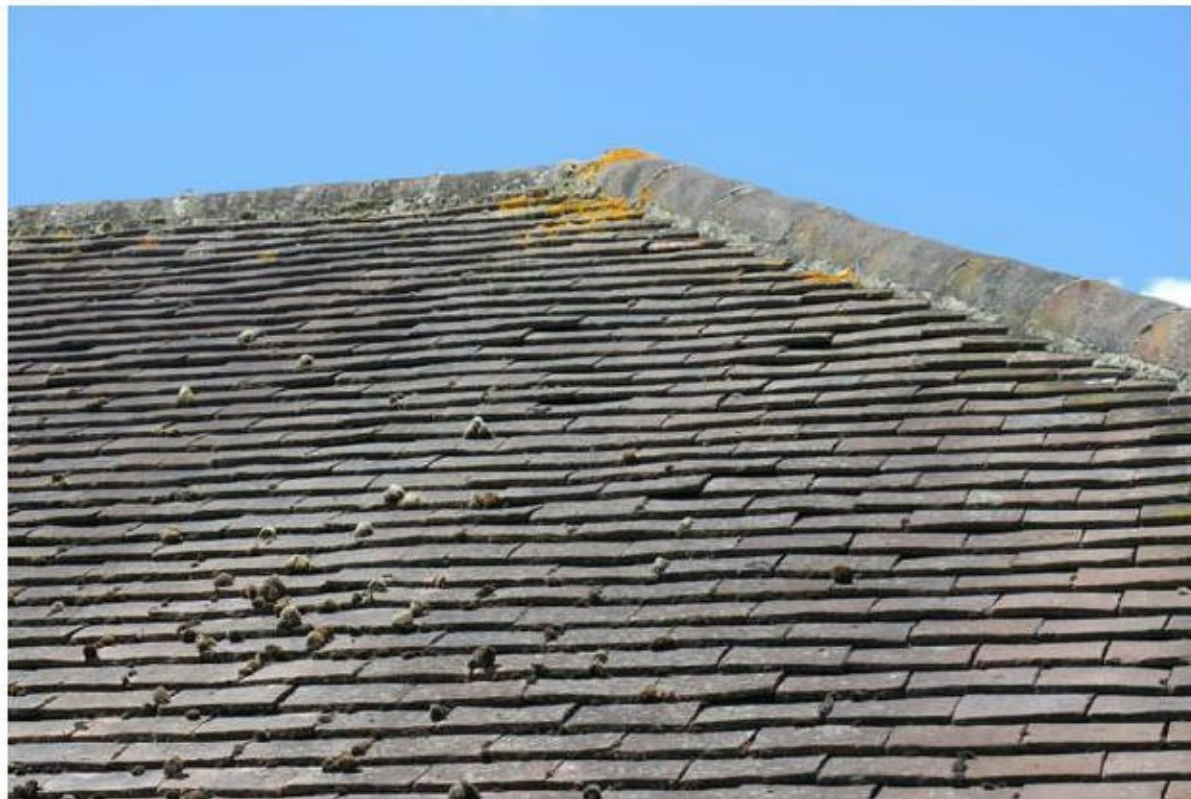
Photograph 3. Tiled surface on eastern roof pitch of the Cottage.
