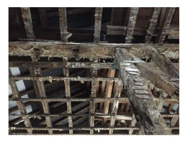
This has reached to the ceiling battens in places, but we intend to retain most of the roof structure. However, the timber partitions, which had already been much damaged by later cut-outs for new doorways, have failed completely. They were of small dimension and had been moved across the room to a position where they have been unable to support the roof above. We shall need to reinstate structural support without altering the dimensions of the rooms.
