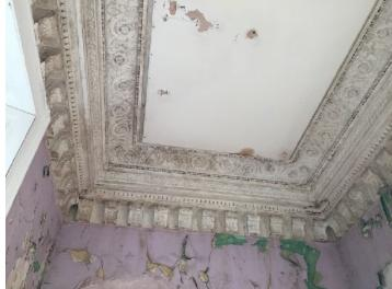
The ceiling central section of plasterboard will need to be removed once the cornice has been propped with the intention of saving most if not all from falling. The floor structure above has been badly damaged by water and dry rot but we are looking at mechanically fixing the cornice back to the walls - all of which are stone or brick.
