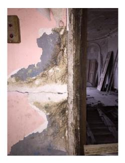
The linking corridor of these two rooms has also suffered. Fortunately none of the ceilings is ornate and the running mould cornices will be easy to repair and replicate.
