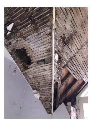
There are various areas of plaster fall, and due to removal of supporting walls, there is a major structural issue in this area which we shall resolve by use of cantilevering steels (invisible when in situ).
