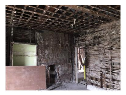
The plaster has already been removed from the partition to lighten its load and to allow the damp within to disperse.
