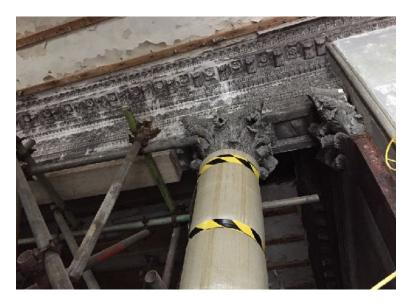
Above: the roof to the rear is collapsing and is now supported on 2-storey scaffolding.
