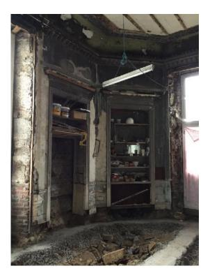
Behind the bookcases, dry rot has been rampant, and on removing the architraves, mycelia can be seen wending their way through the back of the plaster to attack the plaster laths.
