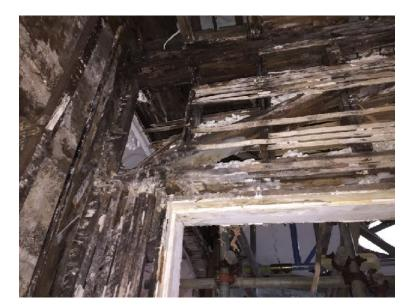
Dry rot has been active here also and the affected timbers will need to be destroyed by incineration.
