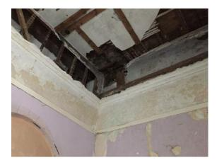
As in every other room, this north facing room has suffered from water ingress from above. The floor surface in the bathroom above is of marble on a lead tray so the water has been cascading down the walls, the weight leading to the failure of the ceiling structure, which has collapsed.
