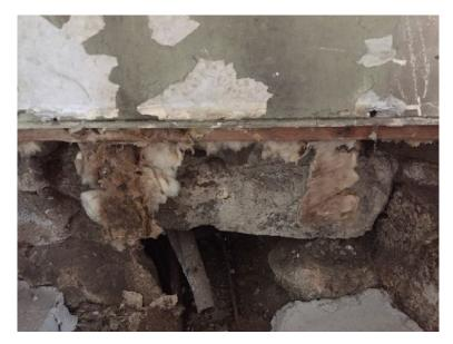
We need to remove the lath and plaster to expose the wall to assist its drying out
