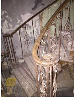
There are a number of missing balusters which are already being made up in wrought iron by Tristan Kessel. We have had several samples made, including by 3D printing, but finally we have found an artist capable of making a direct copy. The treads are oak but thin and much damaged so we are devising a scheme whereby they are the top layer of a strengthened (and invisible) tread supported by the interspersed steel posts behind.
