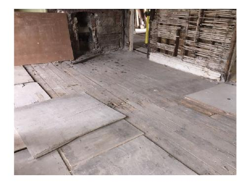
The room has serious structural problems as the flimsy partition has been moved back from its original position (presumably to widen the landing) where it was holding up the roof. Now that it is so badly damaged, it can no longer serve this function and major structural repairs are being designed. At the same time, there is at least one massive original timber in the floor void, and this will be kept as a structural member if at all possible.
