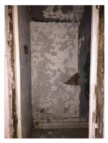
The corridor: Looking through to the corridor beyond, the cracks in the plaster are remarkable.
