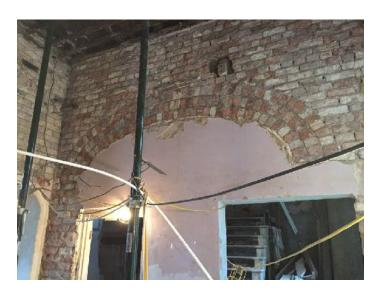
removal of damaged plaster has exposed the archaeology of the walls. Archways and various blocked doorways and interior windows can be seen, together with evidence of old fireplaces and earlier uses. Please see photographs and drawings illustrating this.
