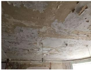
We believe that the original fireplace area (which was later used as an internal bathroom) is the original source of the historic dry rot outbreak - probably a small undetected leak over a number of years.
