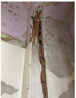
The timber trim to the alcove has been destroyed by rot; we shall reinstate with plaster, keeping the use of timber to a minimum for longevity.
