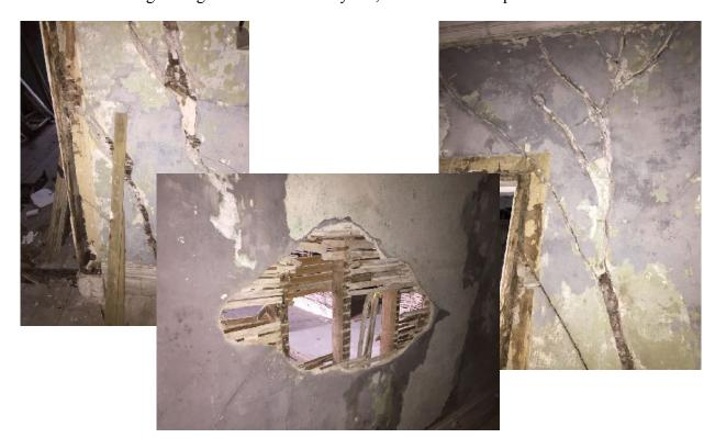
And just as remarkable, is the dry rot in the door frames. However, we have removed the architraves for repair and treatment. They have been labelled and are being stored in the house.
