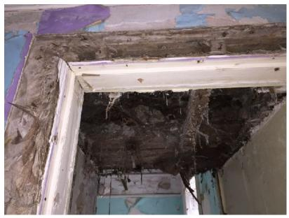
Bedroom 4, however, is the most severely affected by dry rot issues. It is situated below an old rainwater collection tank which had originally and recently been lined with lead until it was stolen along with the roof lead. This meant that most of the water hitting the roof on the whole of this wing was directed through the room (and down to the Anteroom below).
