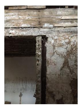
We shall need to introduce a steel framework to support the roof correctly. This means that we can continue to replace the relatively thin partitions and keep the room proportions.
