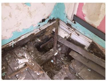
Going back in to the corridor area (previously a bathroom), it has a green and white marble tiled floor sitting in a lead tray. It is much deflected and broken, but we hope to save it to reuse in this area, perhaps by turning it over. We have also managed to retrieve matching marble slabs from this area which were used vertically. from the courtyard behind where they had been removed and smashed in an attempt to steal them. Some will be reusable and whatever we can use we shall.
