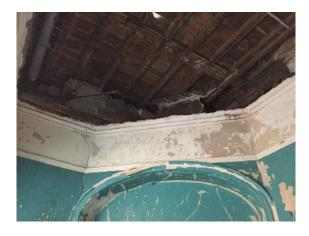
In these photographs you can see the evidence of dry rot mycelia and an earlier higher ceiling height. These traces of earlier walls still have their paint surfaces.
