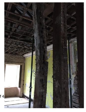
The walls themselves have deep horizontal timber fillets (to which to attach the plaster framework), all of which have rotted, and which we shall replace with brick and slate as a permanent repair.
