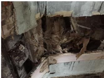
Where the door cases have been removed, the poor construction of the building can be seen. We believe this to be an early C20th change to the room during the Holman ownership.
