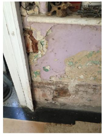
Water damaged plaster on exterior wall which will need to be repaired
