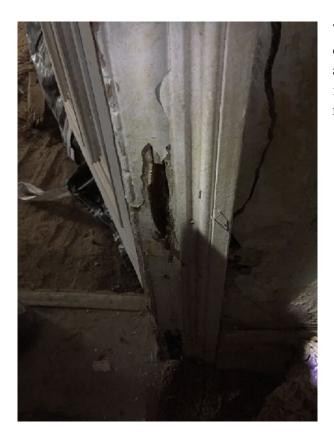
There is a single doorway in this area which opens on to the Drawing Room. Unfortunately its architrave has been damaged by rot, but the door itself and the windows in this area have been repaired and kept safely for reinstatement.
