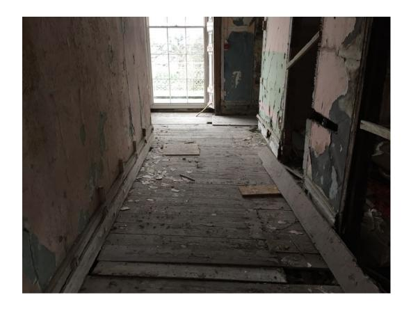
Bedroom 2 is west facing. Unfortunately its ceiling has collapsed, together with its laths, and the floor is deflected by 175mm, so major structural work is required to bring the room back in to use.
