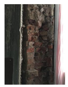
This is the area visibly most badly infested, and from where fruiting bodies were removed on a regular basis. You will see that this is probably the finest cornice in the building, albeit the most damaged.
