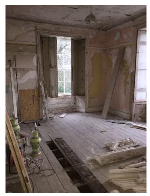
Obviously it has all been soaking wet as the parapet gutters above had been stripped of their lead over the years prior to our arrival. This has led to cracking of the ceiling plaster, damage to floor boards and the growth of mould.
