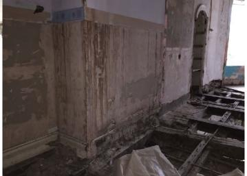
chandeliers in the ballroom below. There are also two very large original timbers at a slight angle; all are to be retained. The floor is very much deflected, however, by as much as 120mm in the hall, so we shall need carefully considered intervention to create a level floor.
