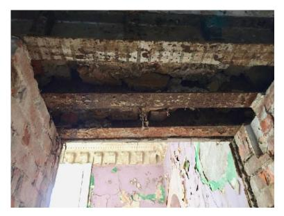
Looking at same lintel between Anteroom and Laundry, the damage to architrave can be seen clearly. The door has been repaired and stored for reinstallation but the door lining and architrave will require replacement.
