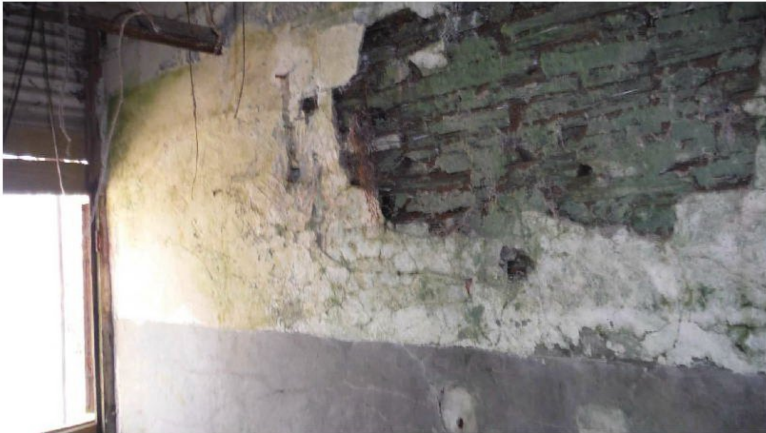
Photograph 6 Internal stone wall
