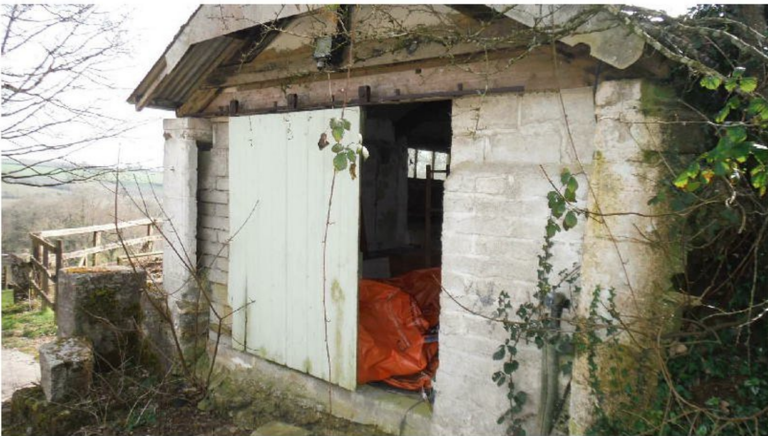
Photograph 2 North gable End
