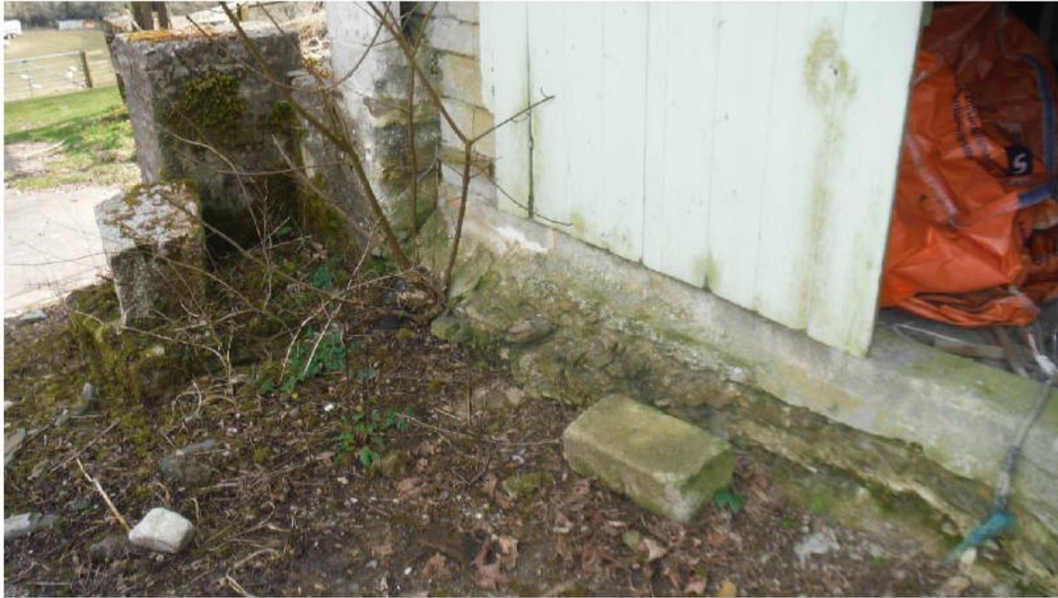
Photograph 5 Door opening to the north gable end wall
