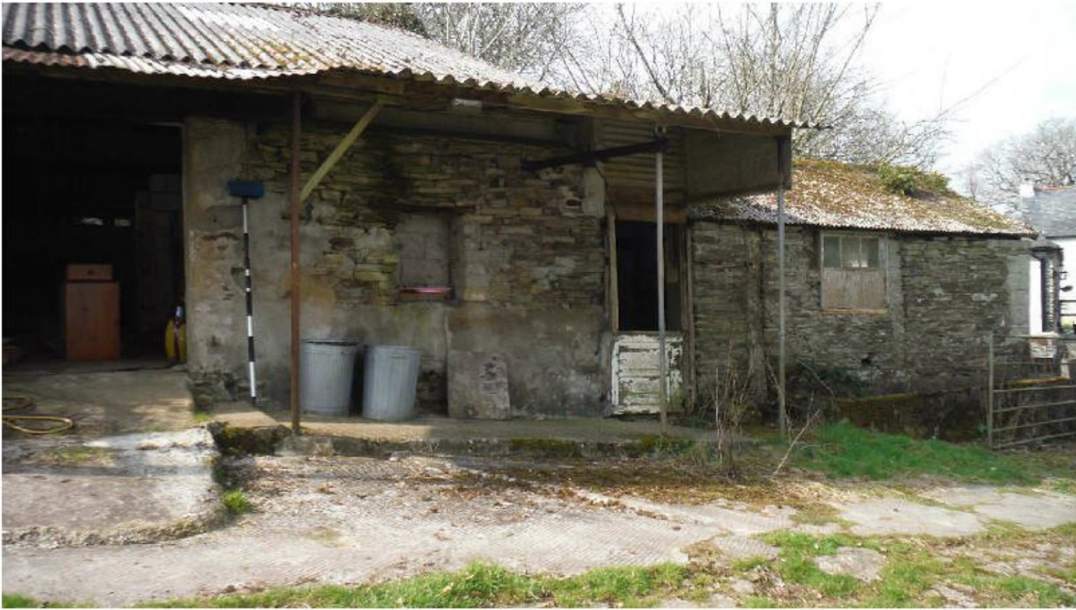
Photograph 1 Stonework walls to the East elevation
