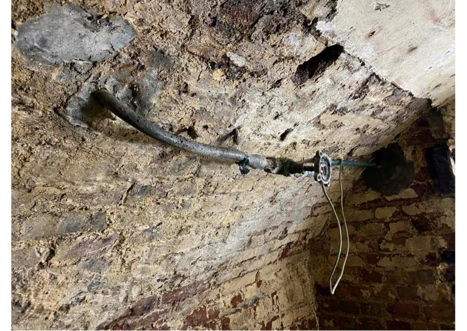
Existing water mains stop cock on vault wall to be relocated to kitchenette
