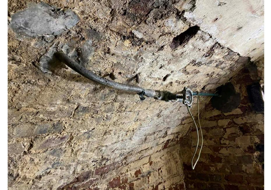
— Existing water mains stop cock on the vault wall to be relocated to the kitchenette
