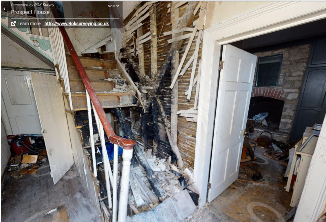
Photo 2 – Music Room - damage to floor and walls
