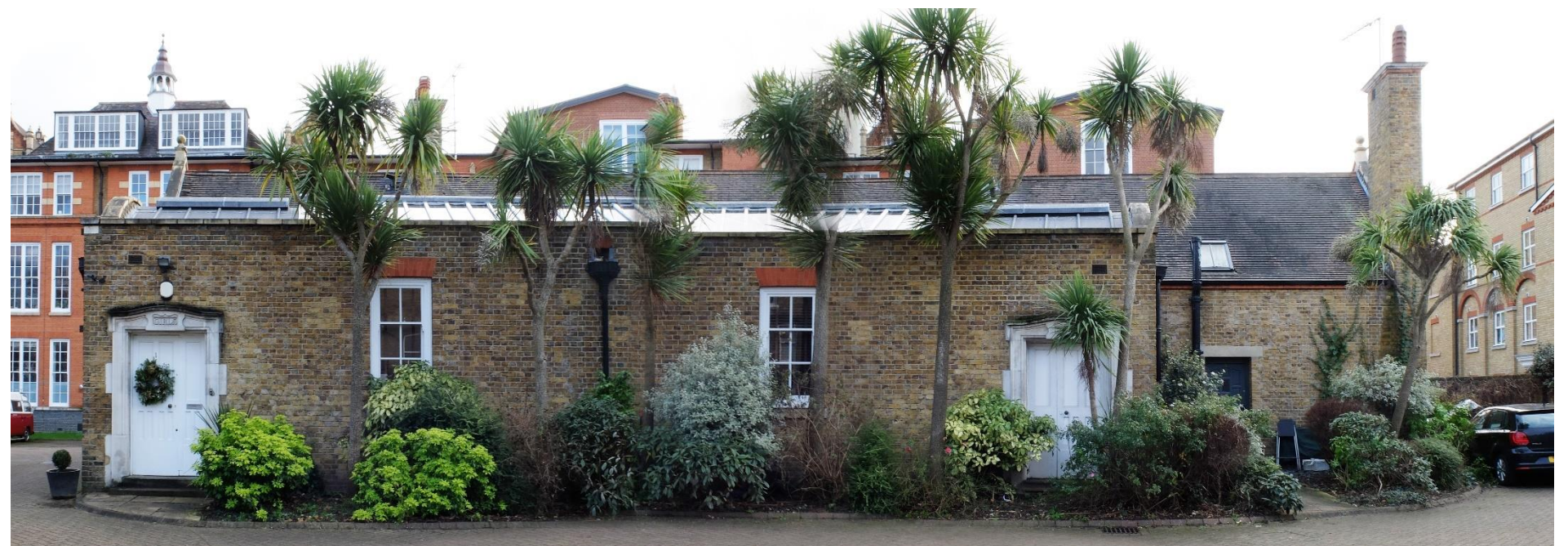
Figure 8: North elevation of kitchen building, showing house No.1
