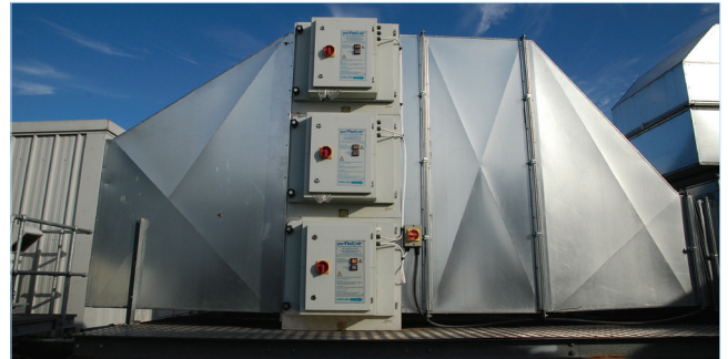
3 ESP Units Stacked in modular formation
