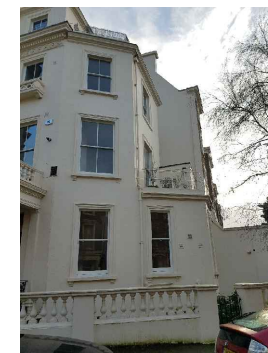
EXISTING BALUSTRADE SIDE
