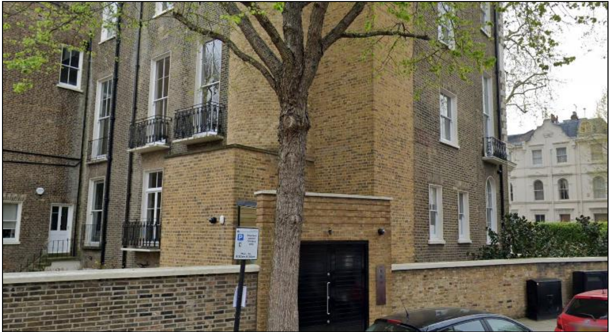
Figure 1 – Railings at No. 1 Randolph Crescent.
