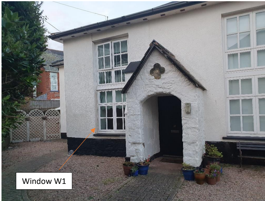
Part Front South Elevation, W1 to left
