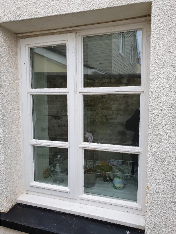
North Rear Elevation W4 ground floor
