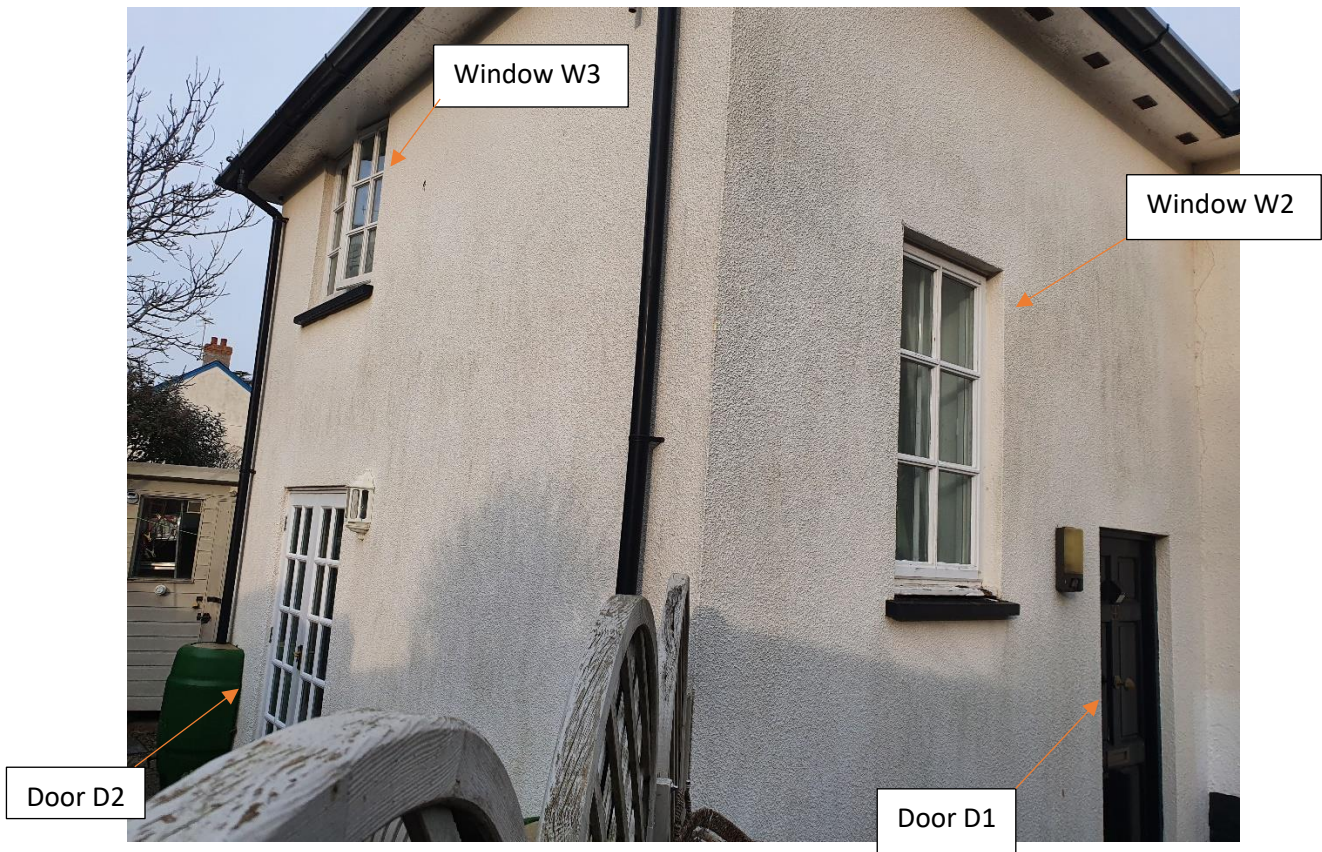
West elevation taken from south west
