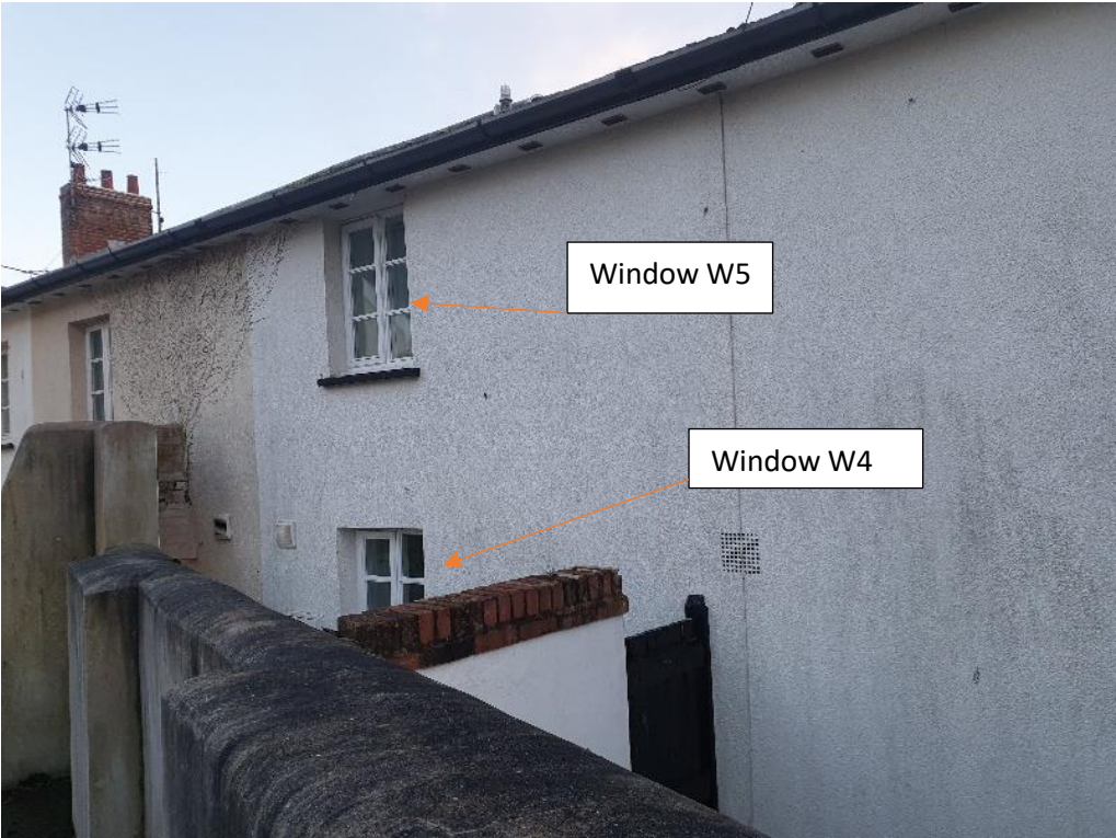
North Rear Elevation W4 ground floor and W5 first floor
