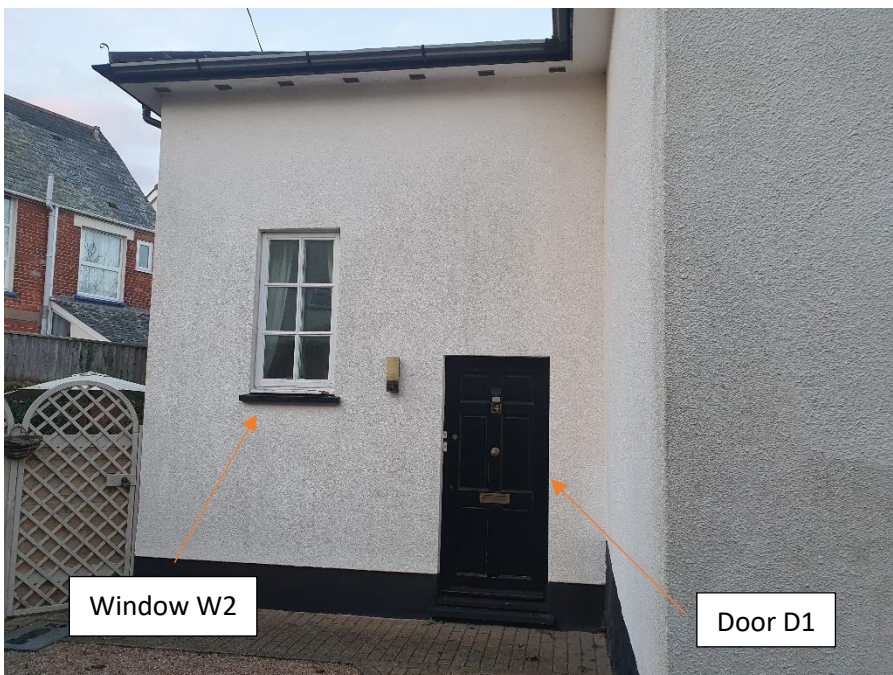
Part Front South Elevation, D1 and W2
