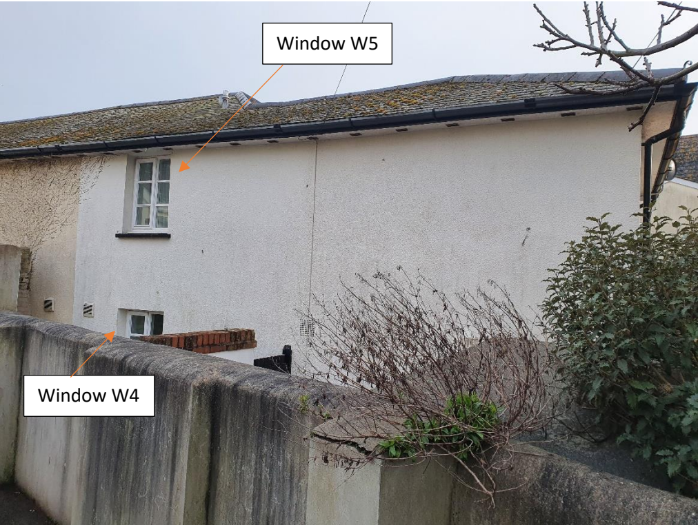
North elevation rear from lane
