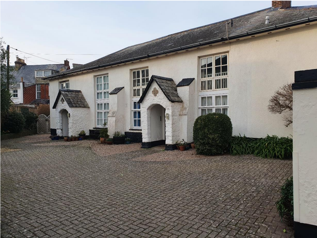
Front elevation of whole building
