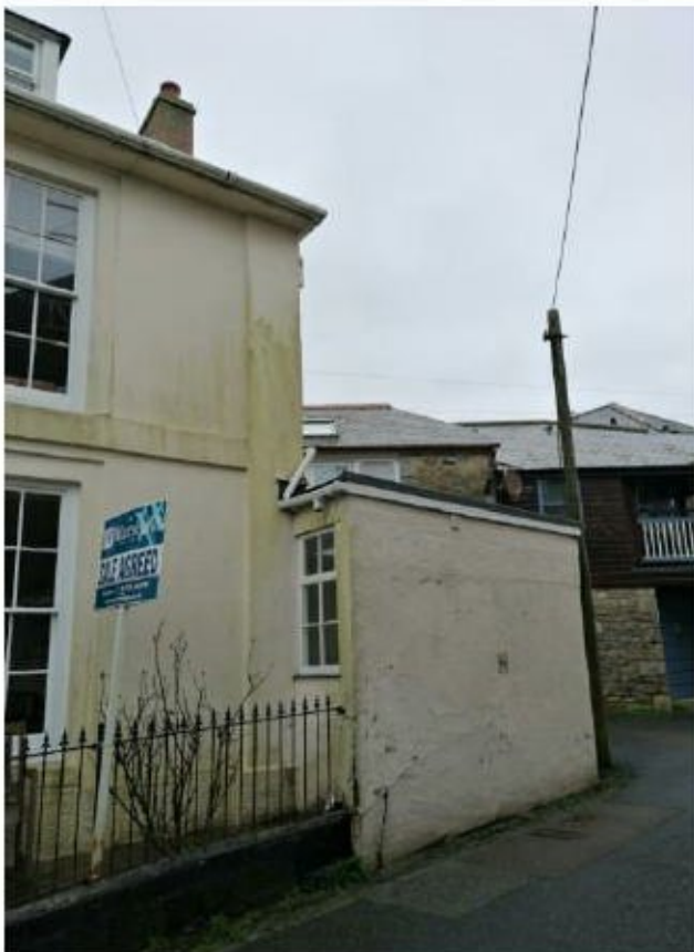
Showing kitchen window, felt flat roof & traditional railings.
