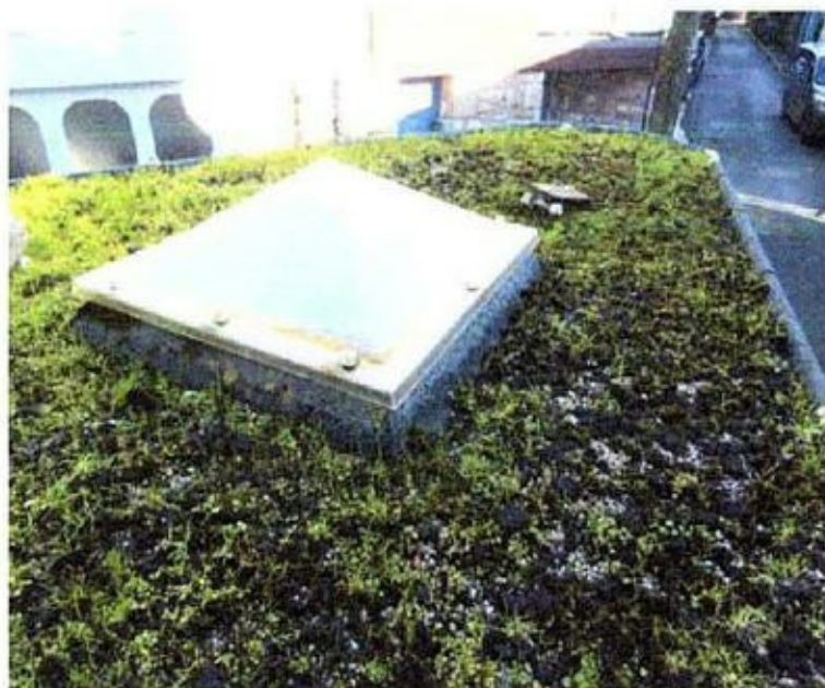
View of flat roof
