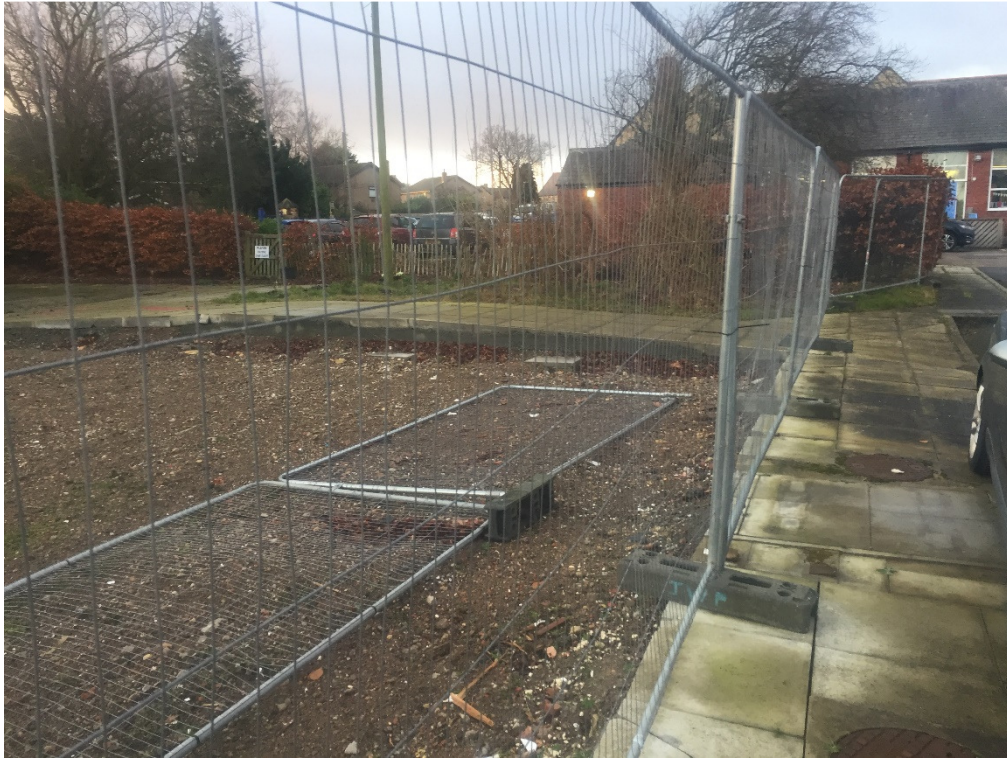
Photograph 3 – Heras fencing between car park and main site area.
