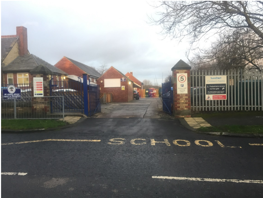
Photograph 1 – School and site entrance on Longhirst Road.
