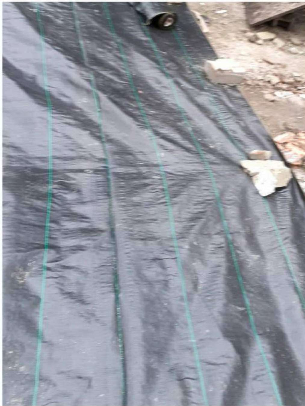
Plate 4 — Further evidence of the geotextile being laid down in the rear garden, before a layer of clean aggregate to build up the correct depth of cover before the decorative chippings were applied.
