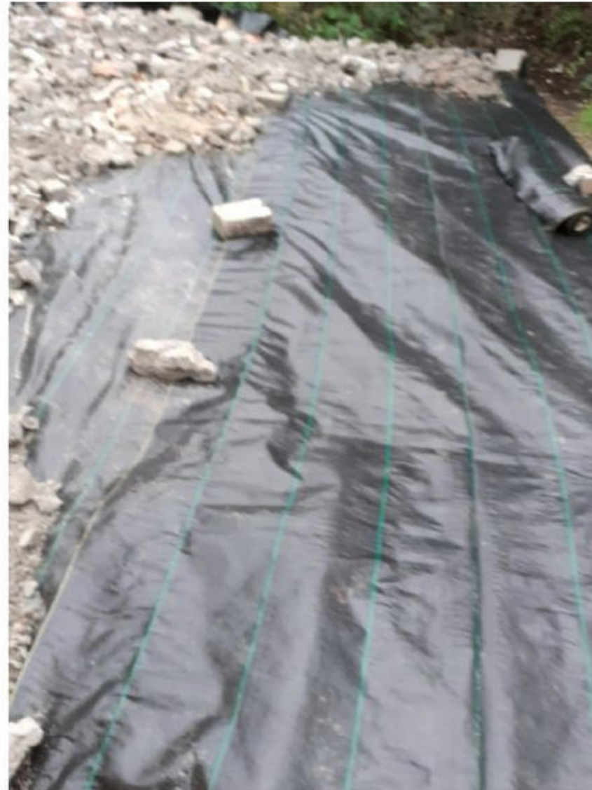
Plate 4 — Further evidence of the geotextile being laid down in the rear garden, before a layer of clean aggregate to build up the correct depth of cover before the decorative chippings were applied.
