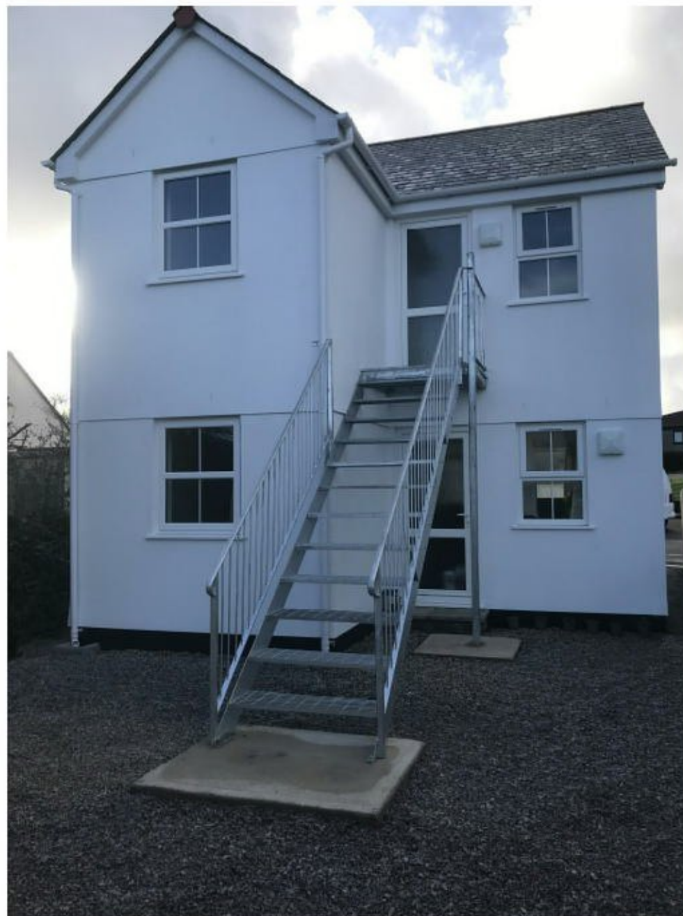
Plate 6 — A view of the rear of the property. The entire rear garden was covered by a gravel cover system of at least 300mm which was considered suitable for breaking the contamination pathway.
